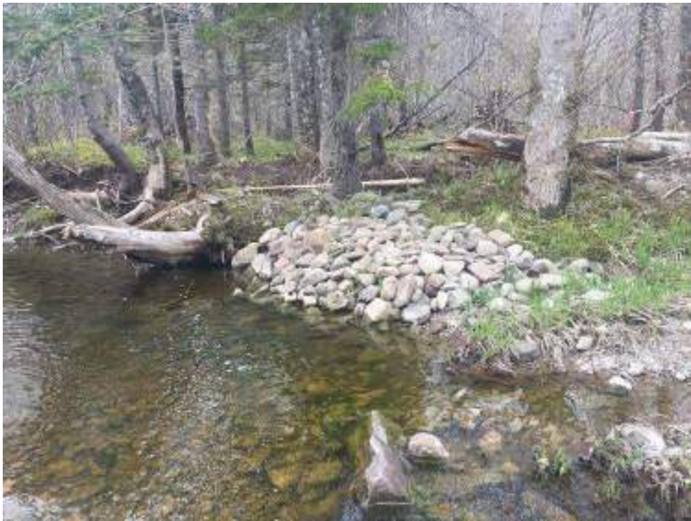
Figure 230. Structure #44 Bank Rock - no maintenance required.
