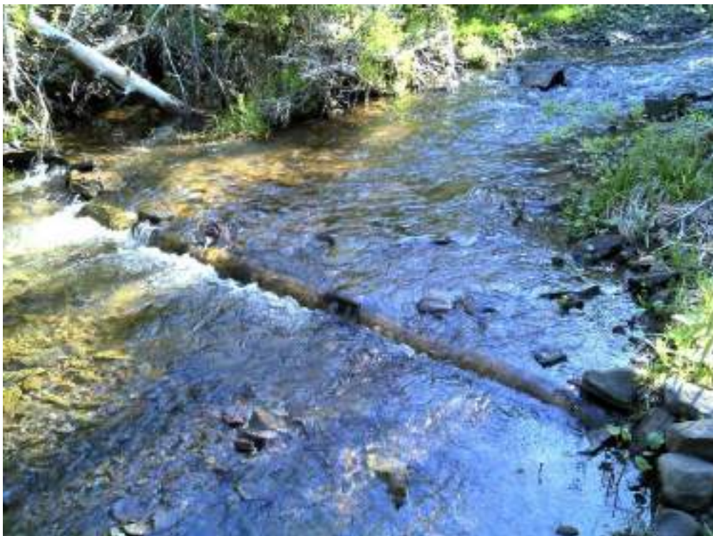
Figure 13. Showing before and after pictures of digger log #5 upstream from the road.
