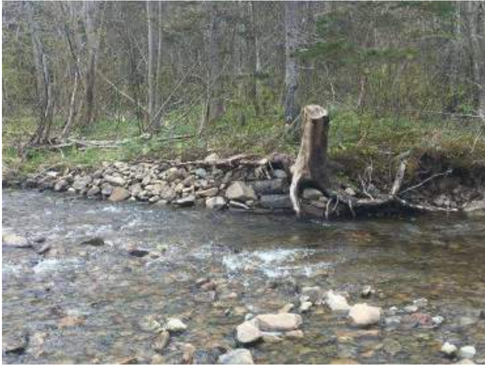
Figure 229. Structure #43 Bank Rock - no maintenance required.
