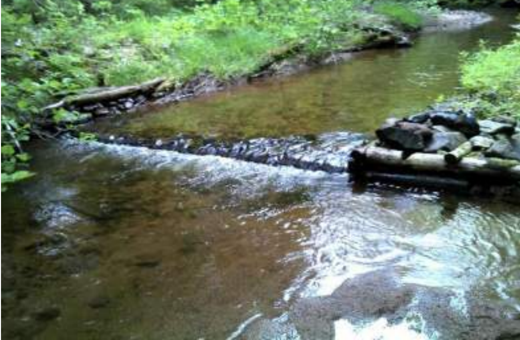
Figure 170. Diggerlog and deflector #9 - after picture of the maintenance performed.
