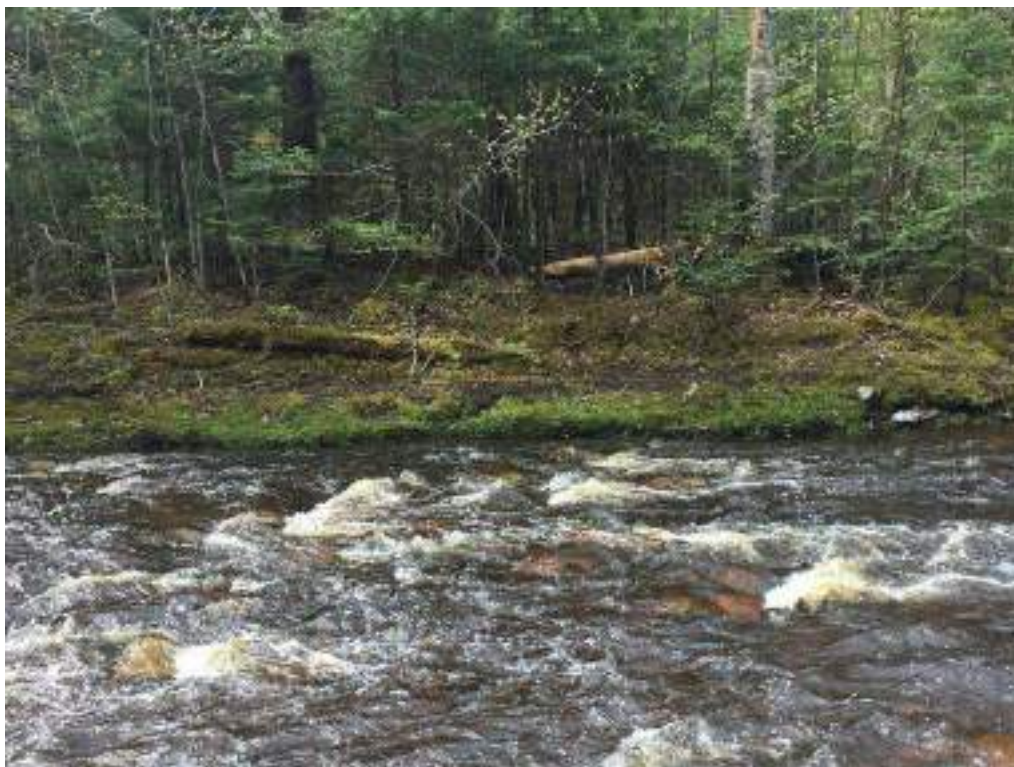
Figure 248. Structure #62 Deflector - missing and requires a rebuild.
