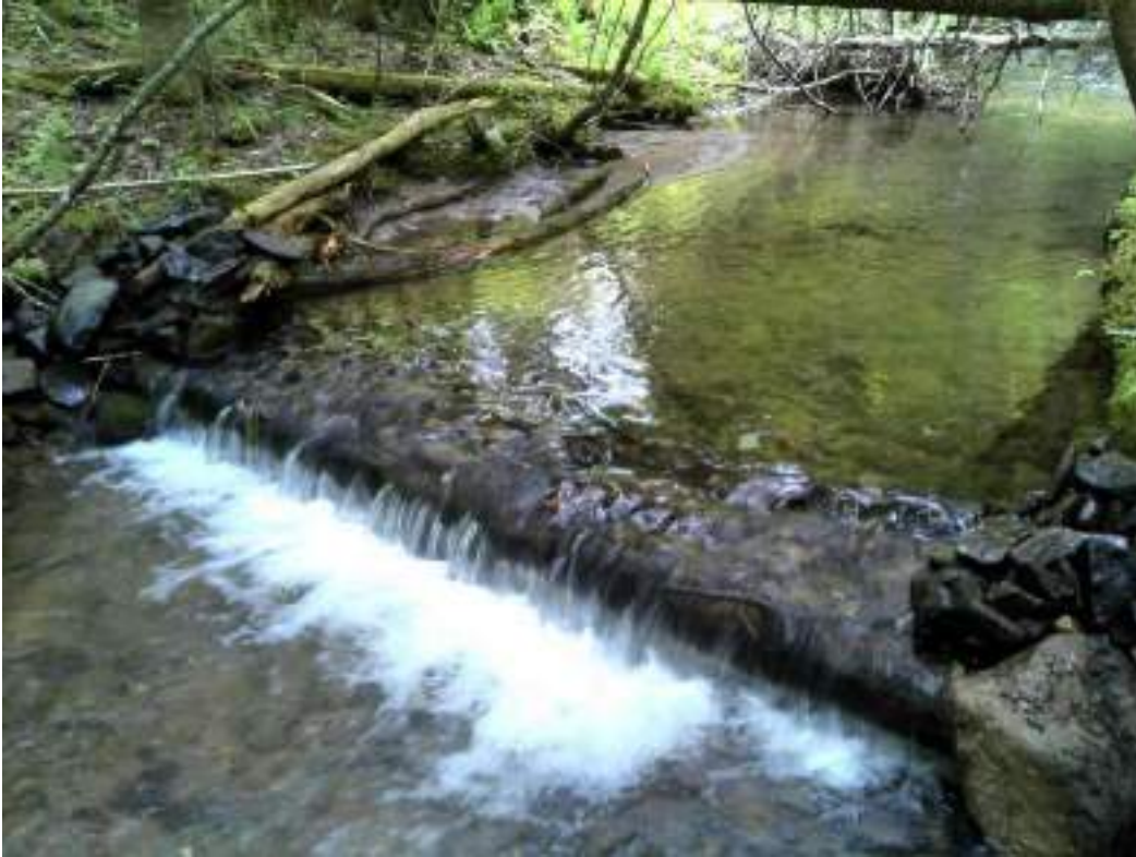
Figure 127. Diggerlog #33 - after picture of maintenance performed.
