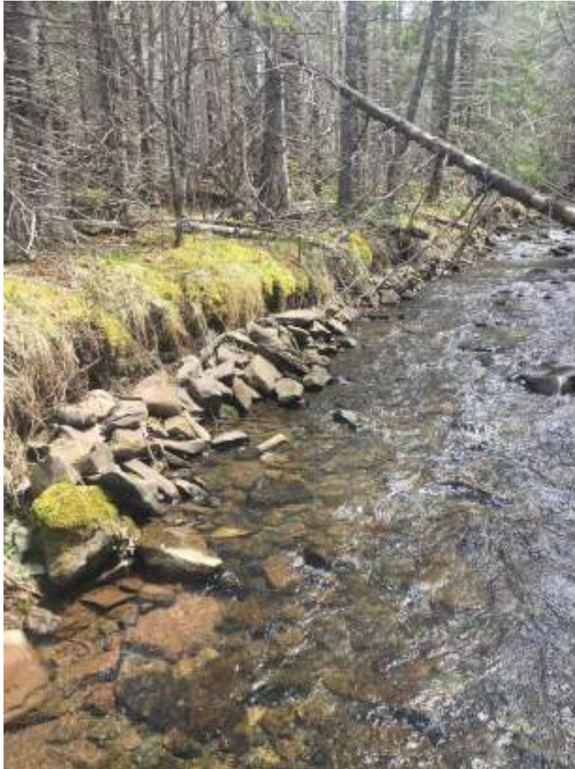
Figure 24. Showing a bank stabilization structure #14 - downstream from the road.
