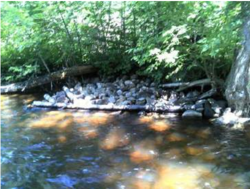
Figure 219. Structure #33 Deflector - before and after picture of completed maintenance.
