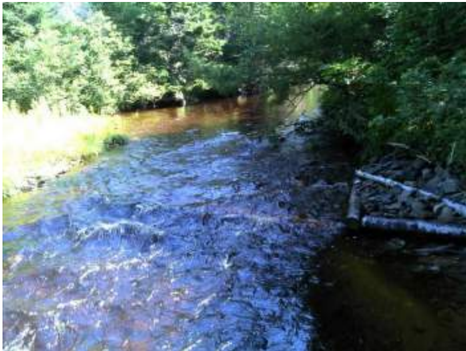
Figure 215. Structure #29 Diggerlog and Deflector - before and after picture of completed maintenance. (water levels are high in the after photo)
