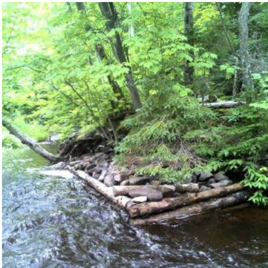
Figure 205. Structure #19 Deflector - before and after pictures of completed maintenance.
