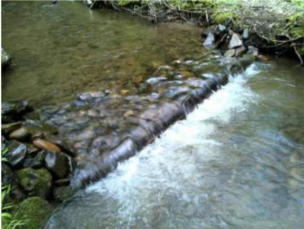
Figure 111. Diggerlog #17 - after picture of maintenance performed.
