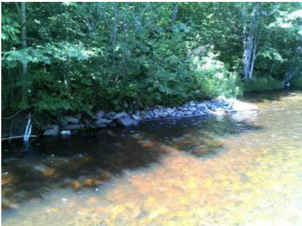
Figure 220. Structure #34 Deflector - before and after picture of completed maintenance.
