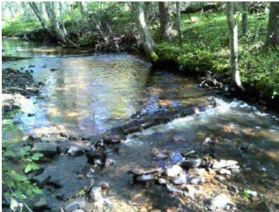
Figure 51. Structure #3 - Diggerlog. Before and after pictures of attempted maintenance. This structure needs an extension on the upstream side of the log.
