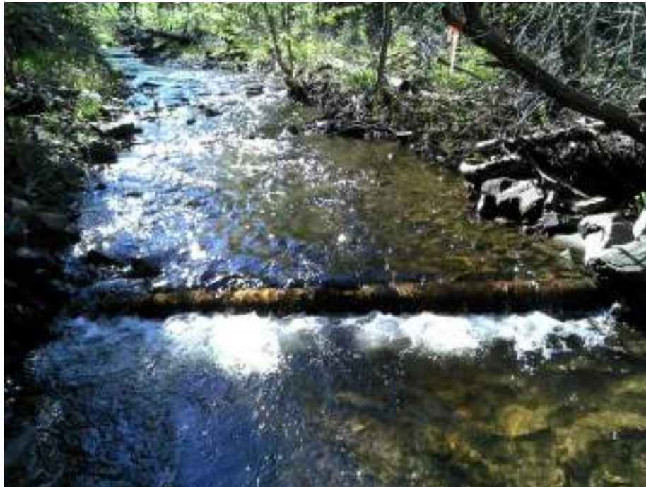
Figure 9. Showing the first digger log structure upstream from the road. Before and after picture of performed maintenance.
