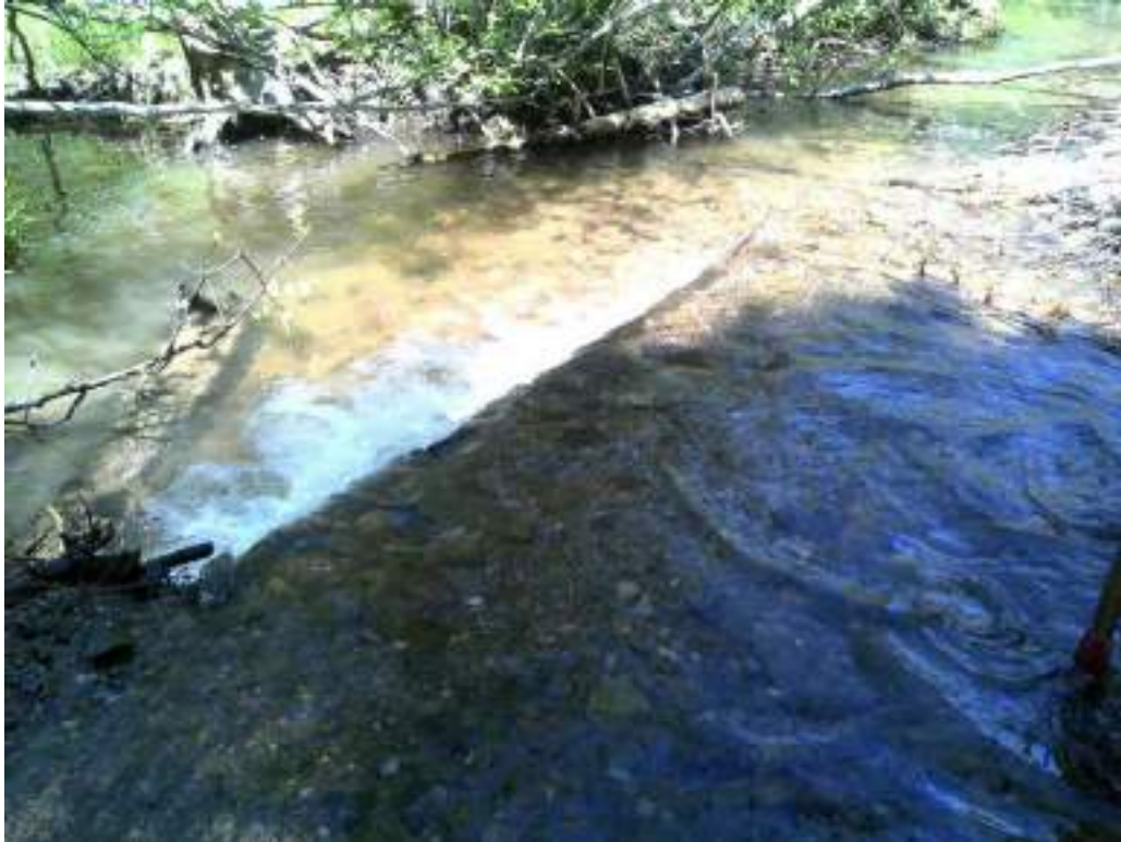
Figure 97. Diggerlog #3 - this picture is taken after maintenance, showing the extension added on the downstream side to restrict water flow to log.
