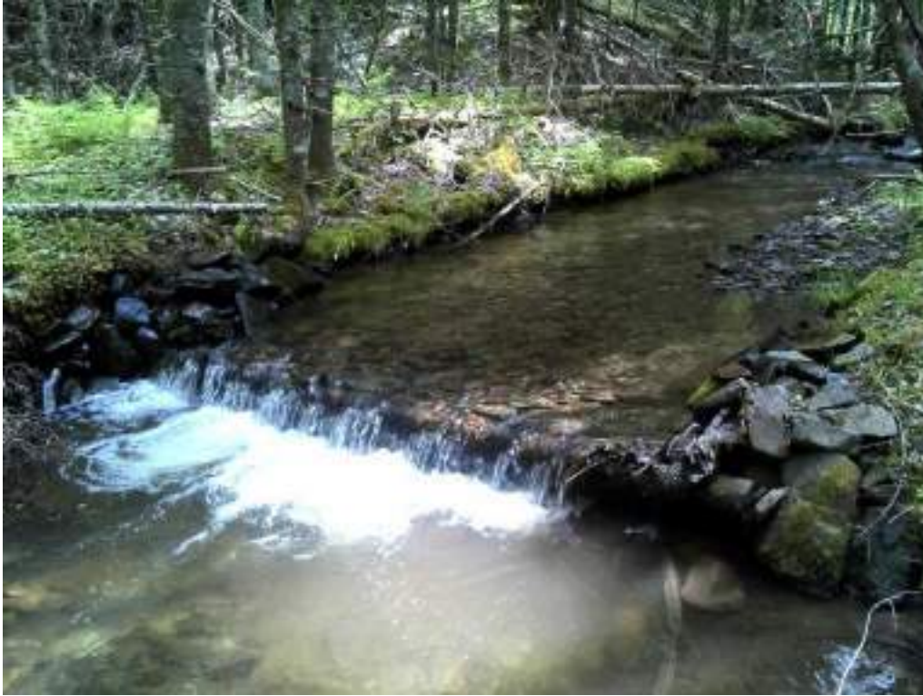
Figure 121. Diggerlog #27 - after picture of maintenance performed.
