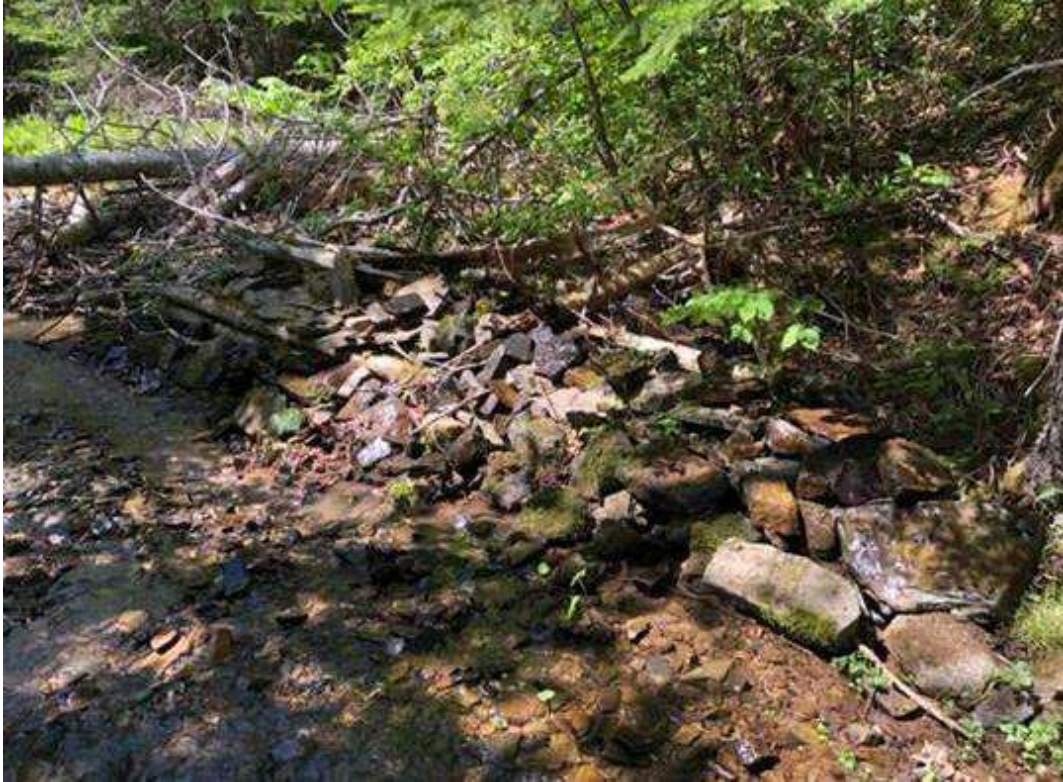
Figure 93. Deflector structure #18 - last structure upstream from Smithville Road.
