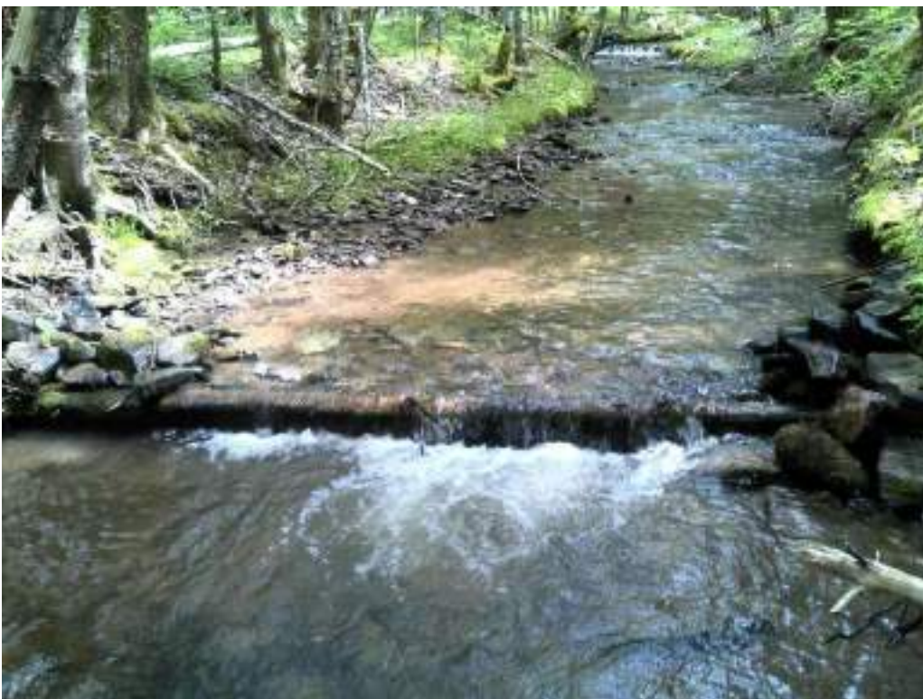
Figure 120. Diggerlog #26 - after picture of maintenance performed.
