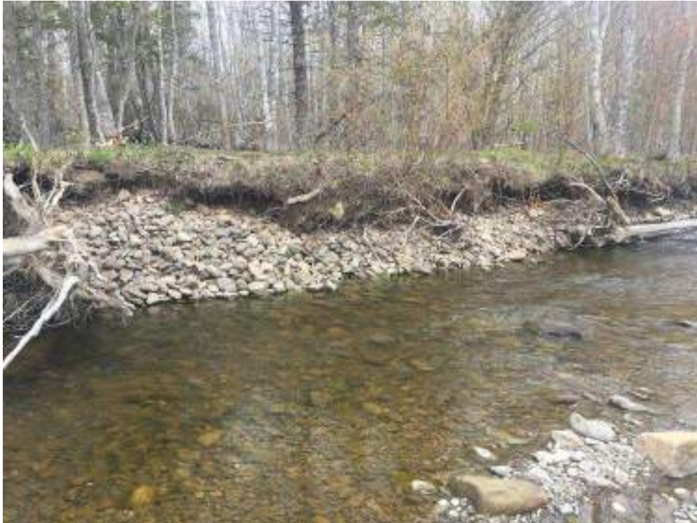
Figure 232. Structure #46 Bank Rock - no maintenance required.
