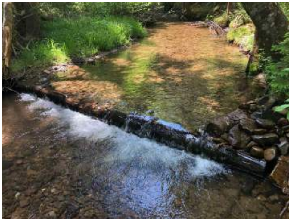
Figure 136. Diggerlog #42 - after picture of maintenance performed.
