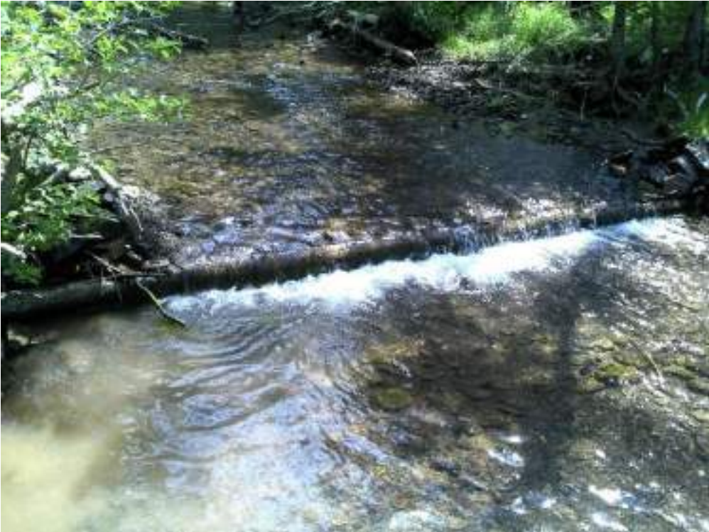
Figure 77. Digger log structure #2 upstream from the Trans Canada Trail.
