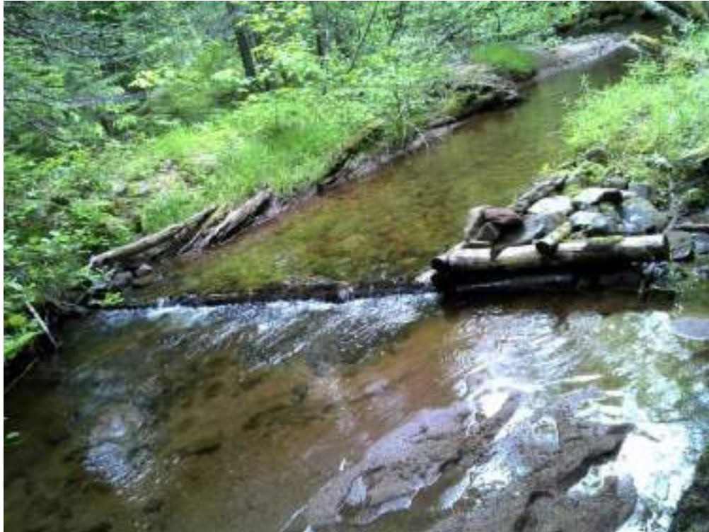
Figure 164 - Diggerlog #3 - after picture of the maintenance performed.
