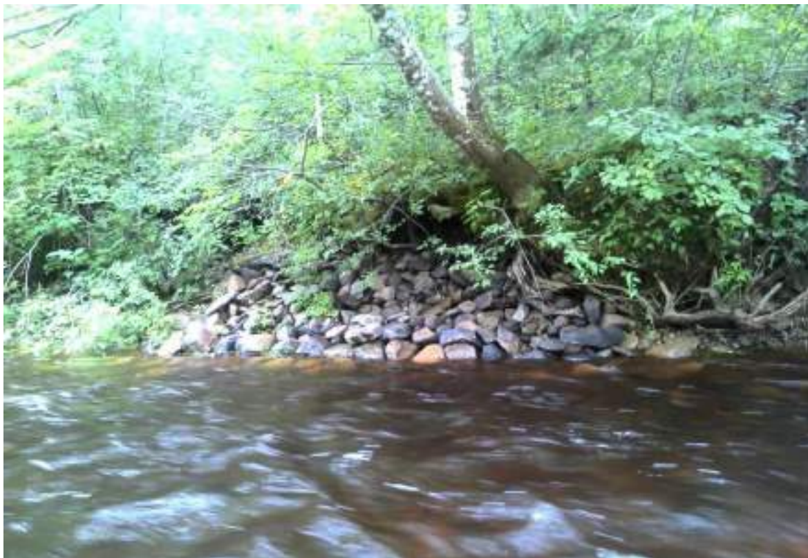
Figure 189. Structure #4 Bank Rock - before and after pictures of completed maintenance.
