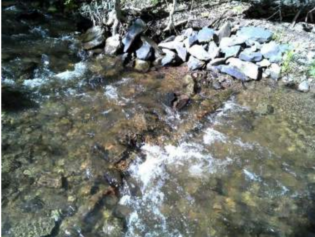
Figure 26. This photo shows a buried digger log - structure #16 on the downstream side of the road. This structure could not be maintained and needs a replacement
