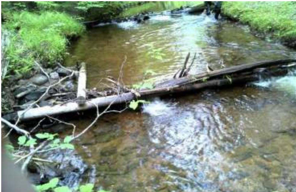
Figure 163. Diggerlog #2 - this structure was undercut in some areas and had a large amount of debris caught on the top of the log. No maintenance was performed.
