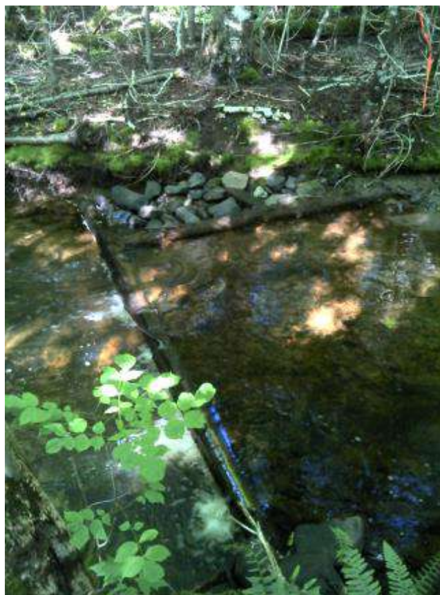
Figure 64. Structure #16 - Before and after picture of the maintenance completed on a digger log and deflector structure.
