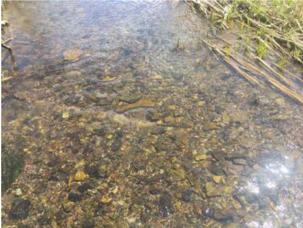
Figure 82. Structure #7 - buried diggerlog that needs a replacement.
