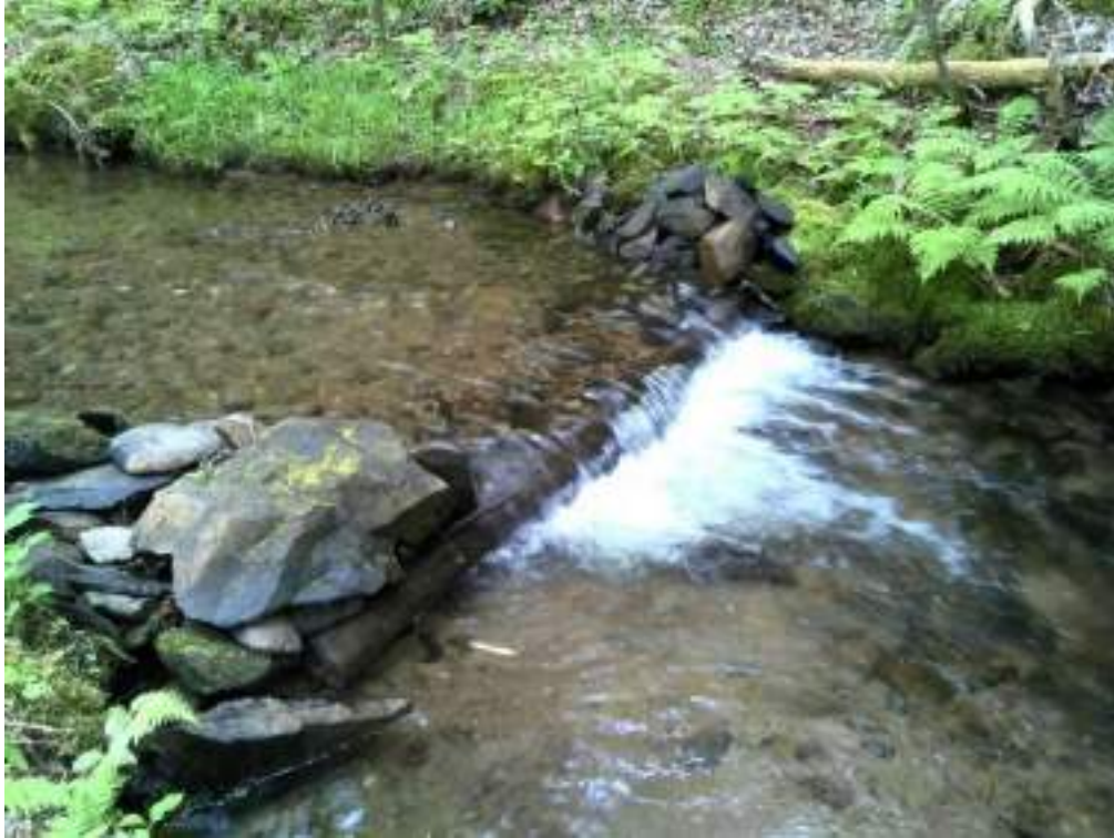
Figure 131. Diggerlog #37 - after picture of maintenance performed.
