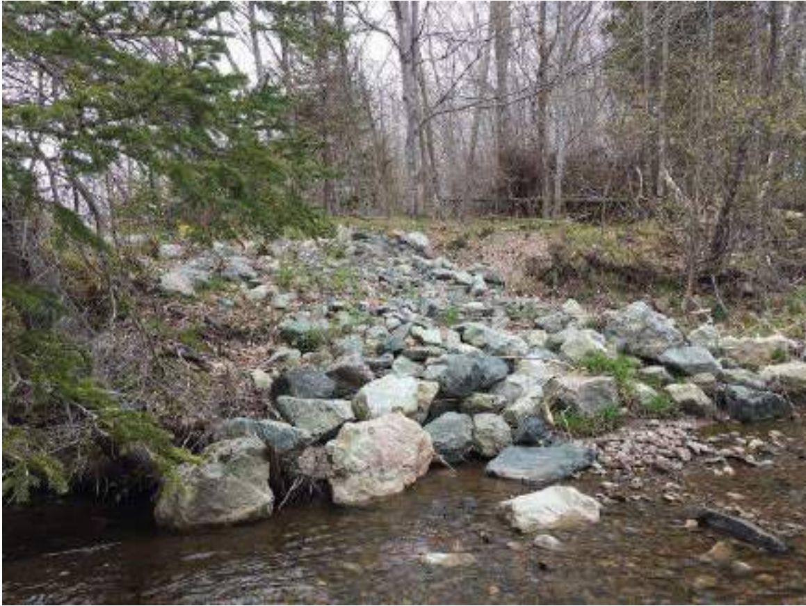
Figure 206. Structure #20 Armour Stone - bank stabilization, across from structure #19.
