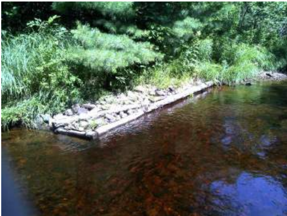
Figure 213. Structure #27 Deflector - before and after picture of completed maintenance.
