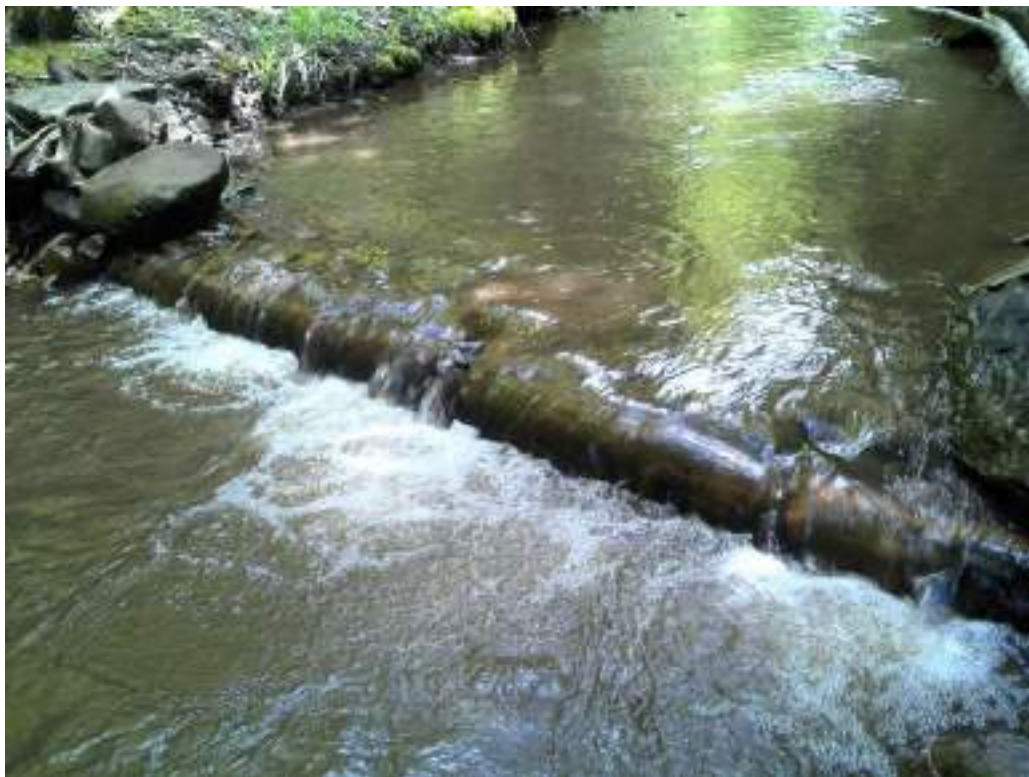
Figure 106. Diggerlog #12 - after picture of maintenance performed.
