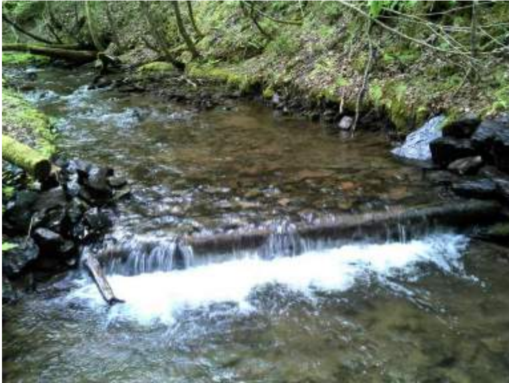
Figure 123. Diggerlog #29 - after picture of maintenance performed.
