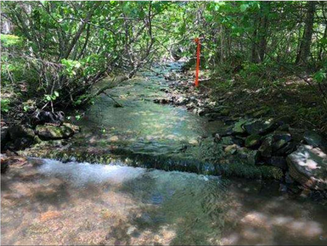
Figure 85. Diggerlog structure #10 - downstream side of Smithville Road.
