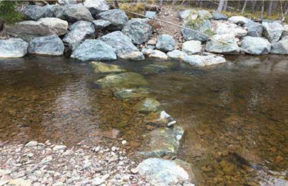
Figure 193. Structure #8 Armour Stone Rock Sill
