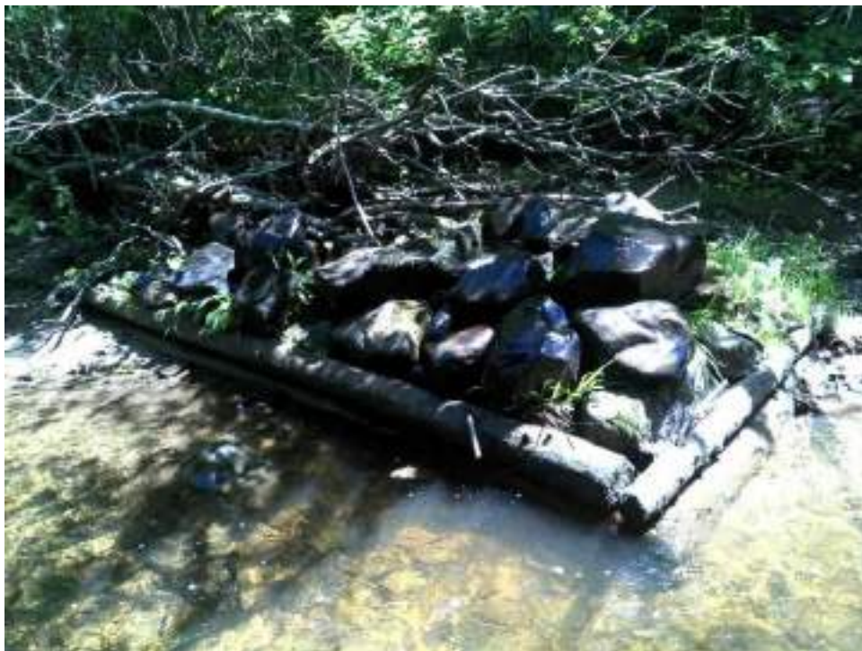
Figure 140. Before and after picture of the maintenance performed on deflector #3.
