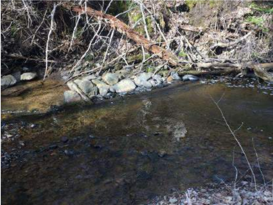
Figure 53. Structure #5 - after picture of the maintenance completed on a deflector.
