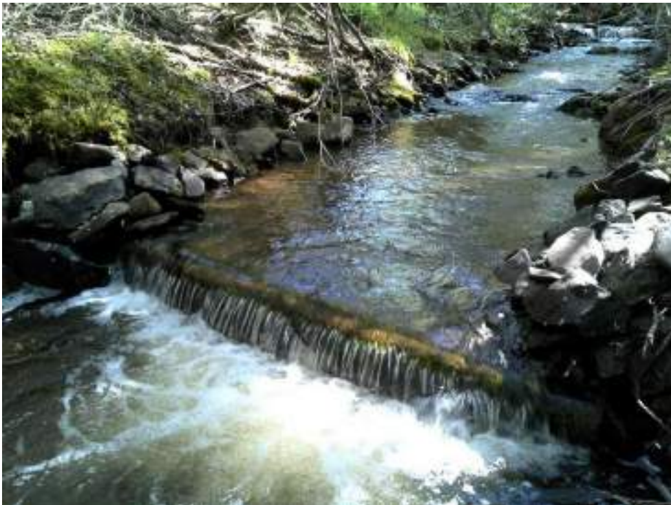
Figure 21. Showing the before and after photos of a digger log - structure #11 downstream from the road.
