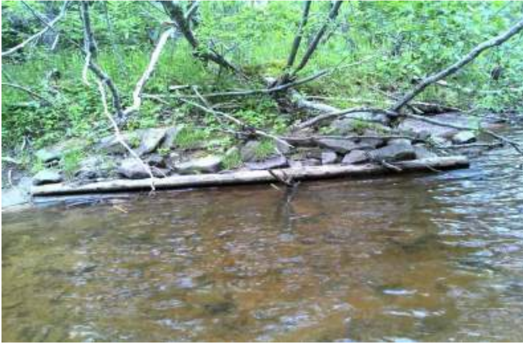
Figure 153. Deflector #6 - this deflector is now growing vegetation on it and is slowly becoming part of the bankside.
