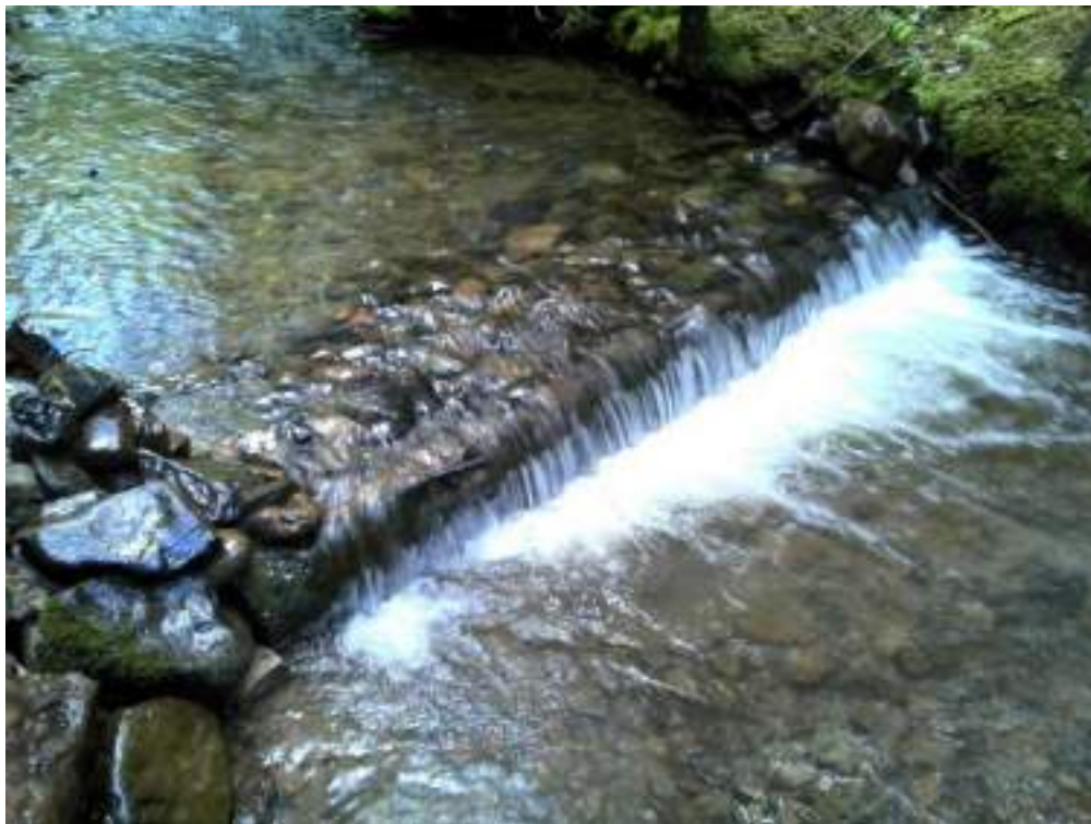
Figure 114. Diggerlog #20 - after picture of maintenance performed.
