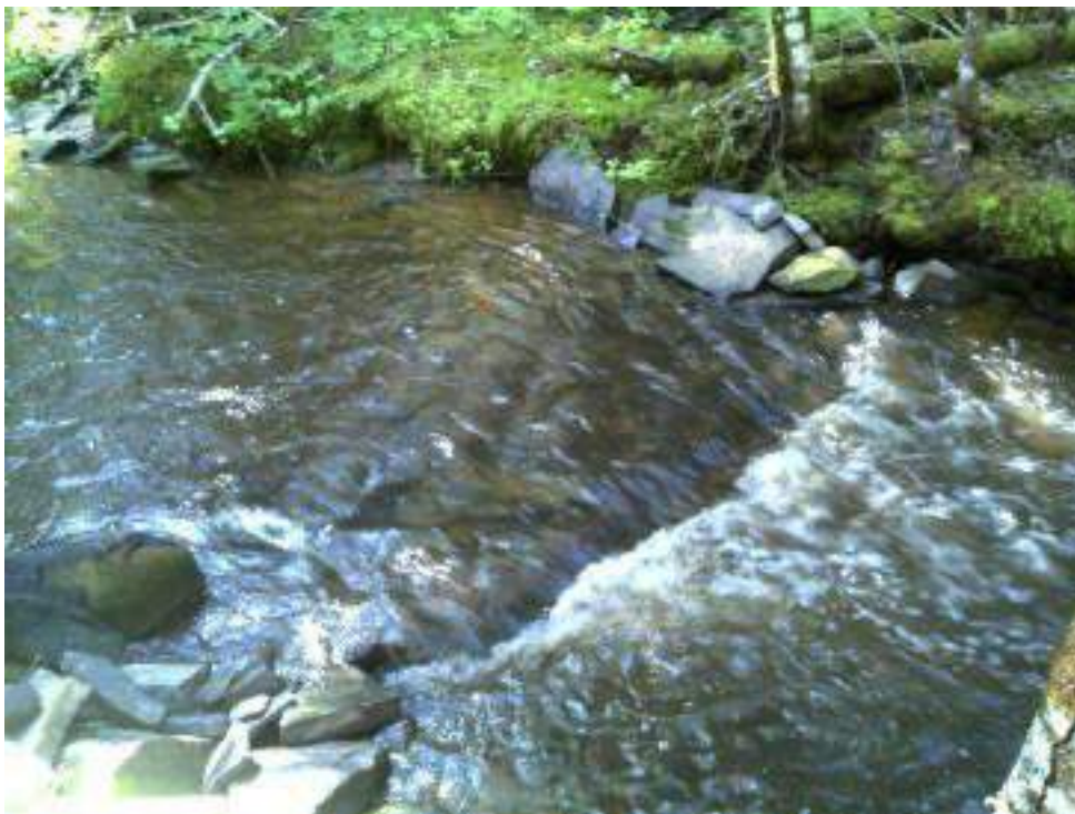
Figure 179. Structure #8 - After picture of the maintenance completed on a digger log.
