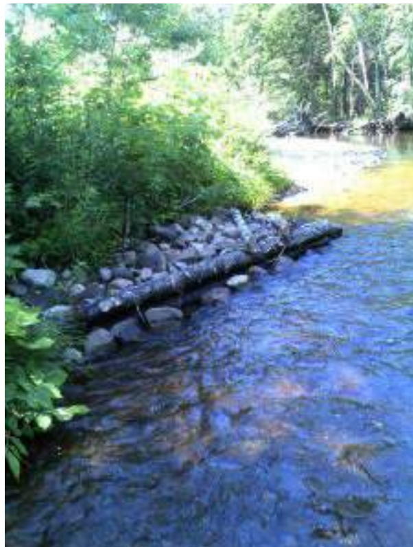
Figure 218. Structure #32 Deflector - before and after picture of completed maintenance.
