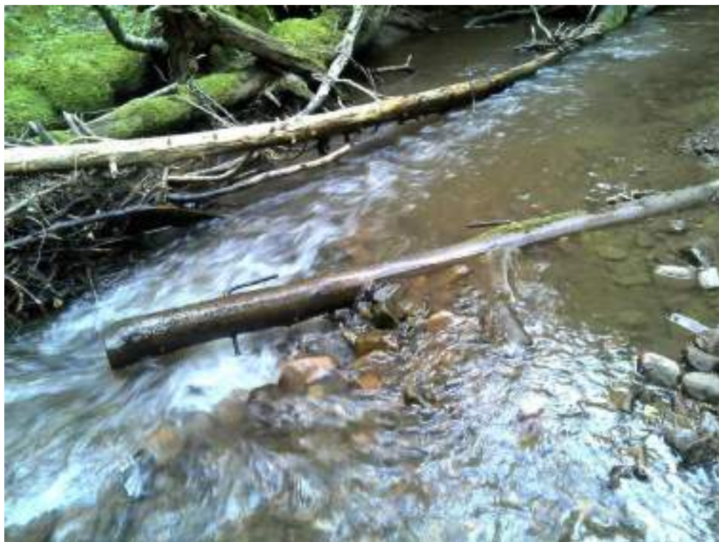
Figure 110. Diggerlog #16 - no maintenance performed. Structure needs to be removed and replaced.
