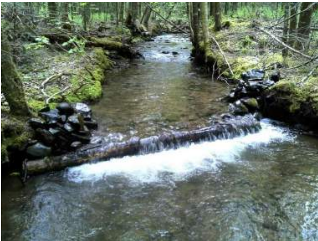
Figure 122. Diggerlog #28 - after picture of maintenance performed.
