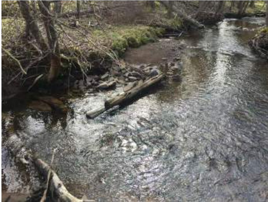
Figure 50. Structure #2 - Deflector that needs replacement. No maintenance completed.
