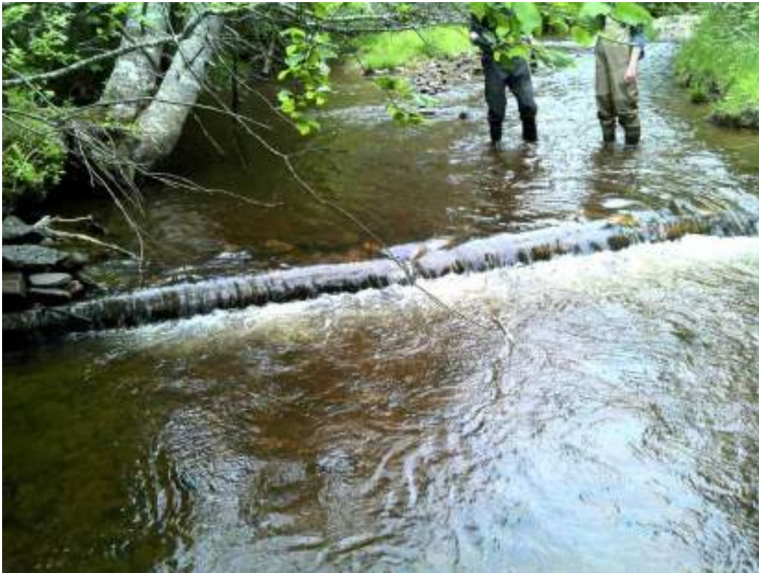
Figure 158. Diggerlog #11 - after picture of the maintenance performed.
