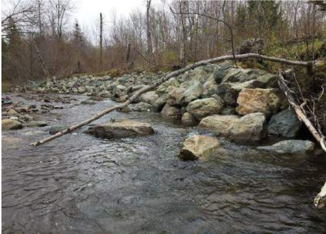
Figure 203. Structure #17 Armour Stone - bank stabilization.
