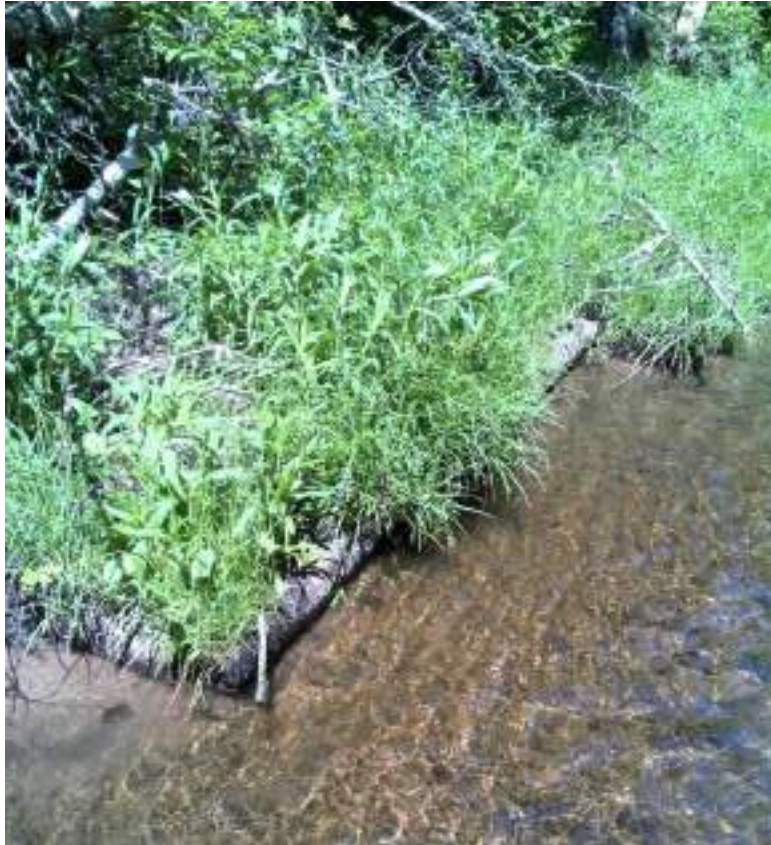
Figure 142. Deflector #5 - this deflector is in very good condition and is now becoming part of the bank side and has lots of vegetation growth.
