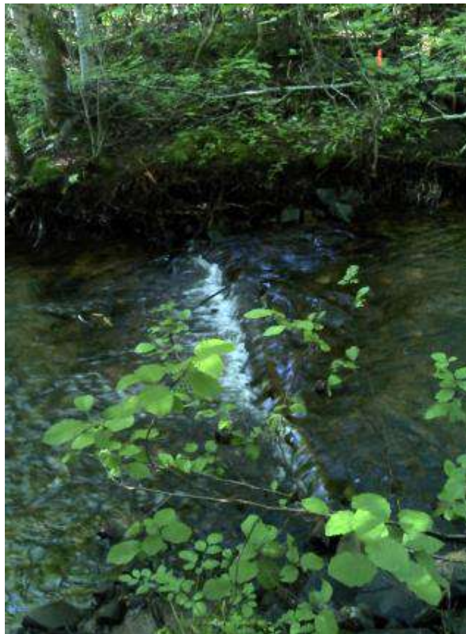
Figure 62. Structure #14 - Before and after picture of the maintenance completed on a diggerlog.
