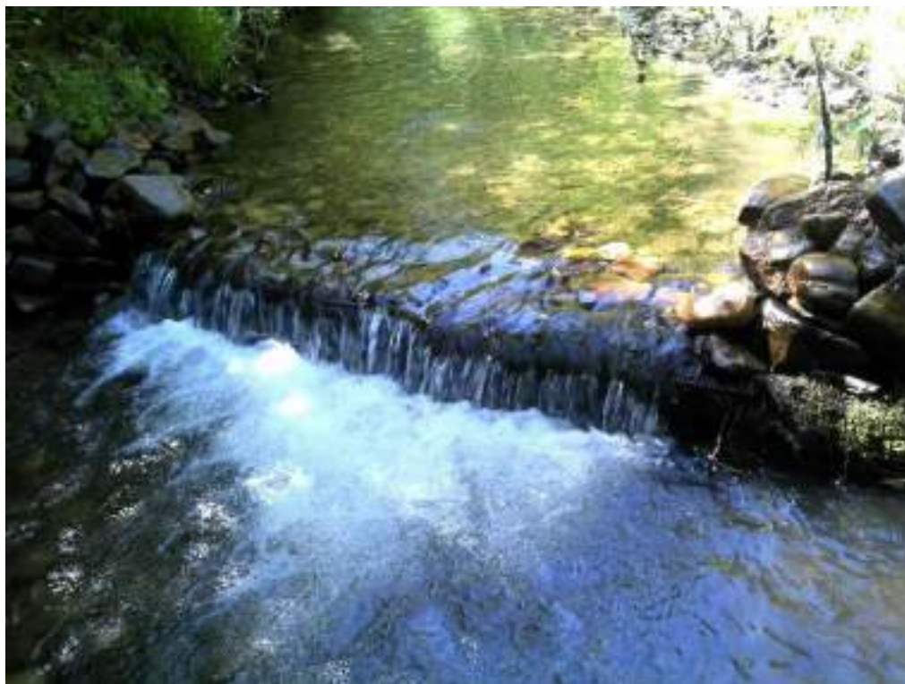
Figure 102. Diggerlog #8 - after picture of maintenance performed.
