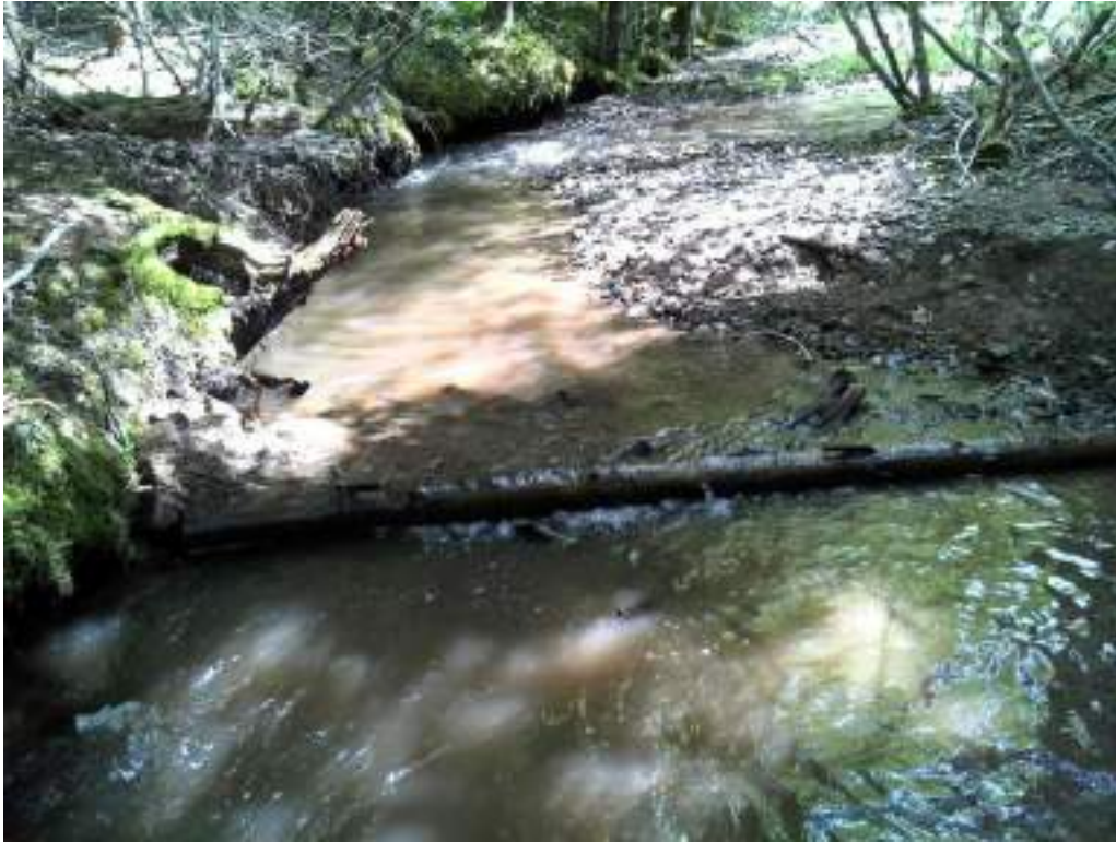
Figure 107. Diggerlog #13 - picture of the maintenance attempted on this structure.
