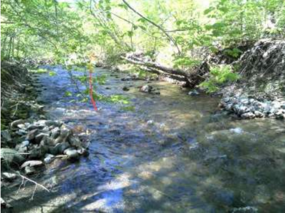
Figure 35. Deflector #8 - before and after pictures of maintenance.
