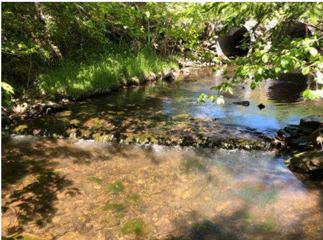
Figure 86. Diggerlog structure #11 - downstream side of Smithville Road.
