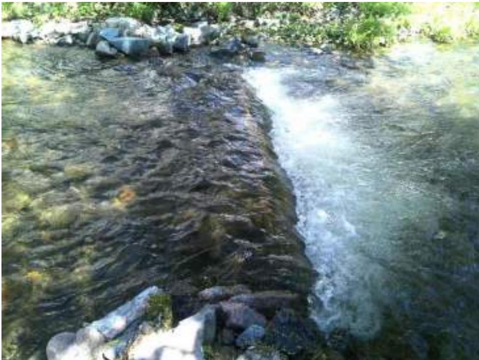
Figure 28. Diggerlog #1 - before and after pictures of maintenance. This is the furthest structure downstream.
