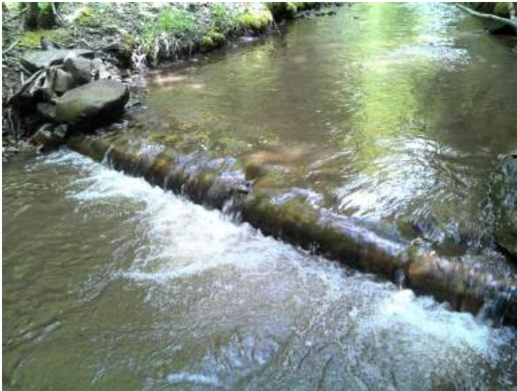
Figure 105. Diggerlog #11 - after picture of maintenance performed.
