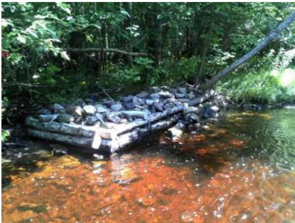
Figure 207. Structure #21 Deflector - before and after pictures of completed maintenance.
