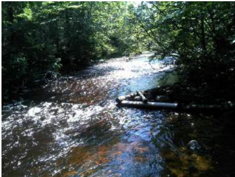
Figure 217. Structure #31 Diggerlog and Deflector - before and after picture of completed maintenance.
