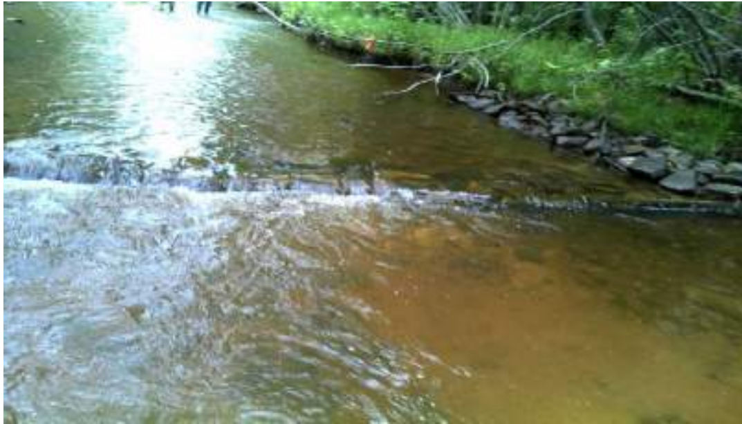
Figure 159. Diggerlog #12 - after picture of maintenance performed.
