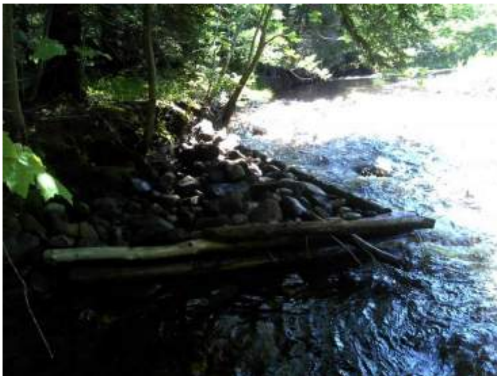
Figure 211. Structure #25 Deflector - before and after picture of completed maintenance.
