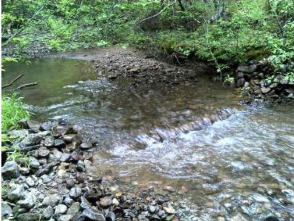
Figure 109. Diggerlog #15 - after picture of maintenance performed.
