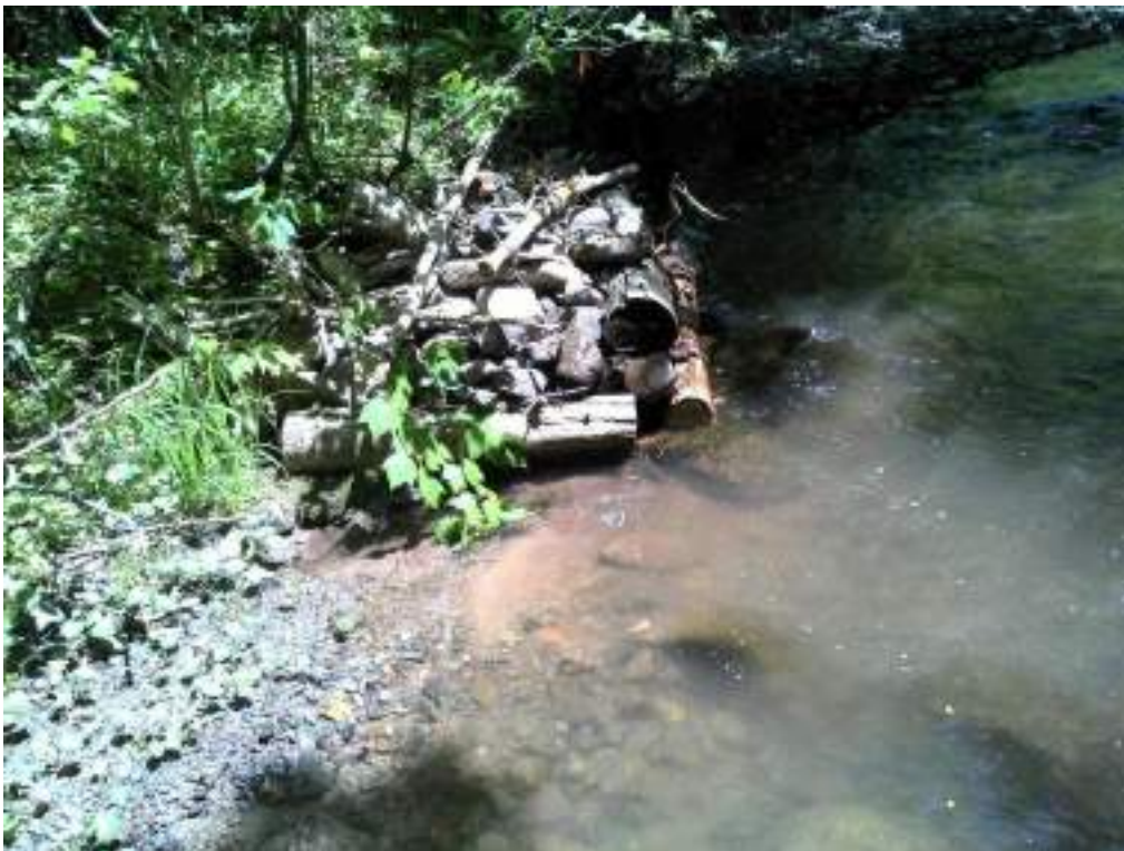
Figure 116. Deflector structure #22 - after picture of maintenance performed.
