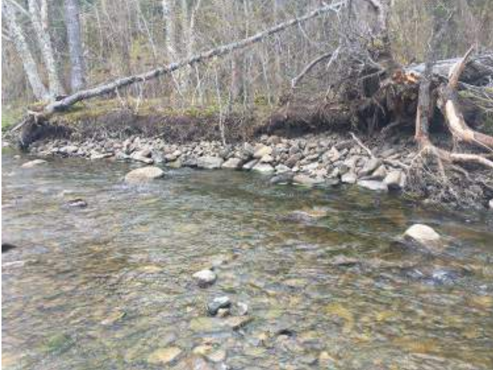
Figure 234. Structure #48 Bank Rock - no maintenance required.
