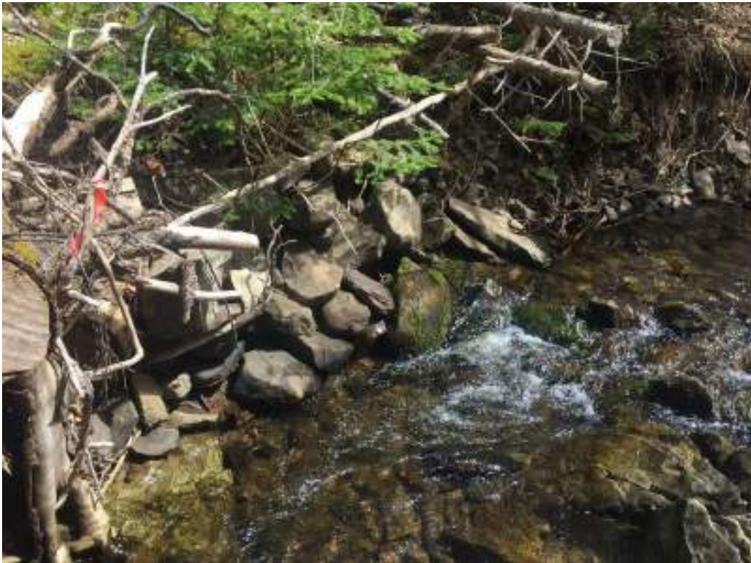
Figure 23. Showing a bank stabilization structure - #13 downstream from the road
