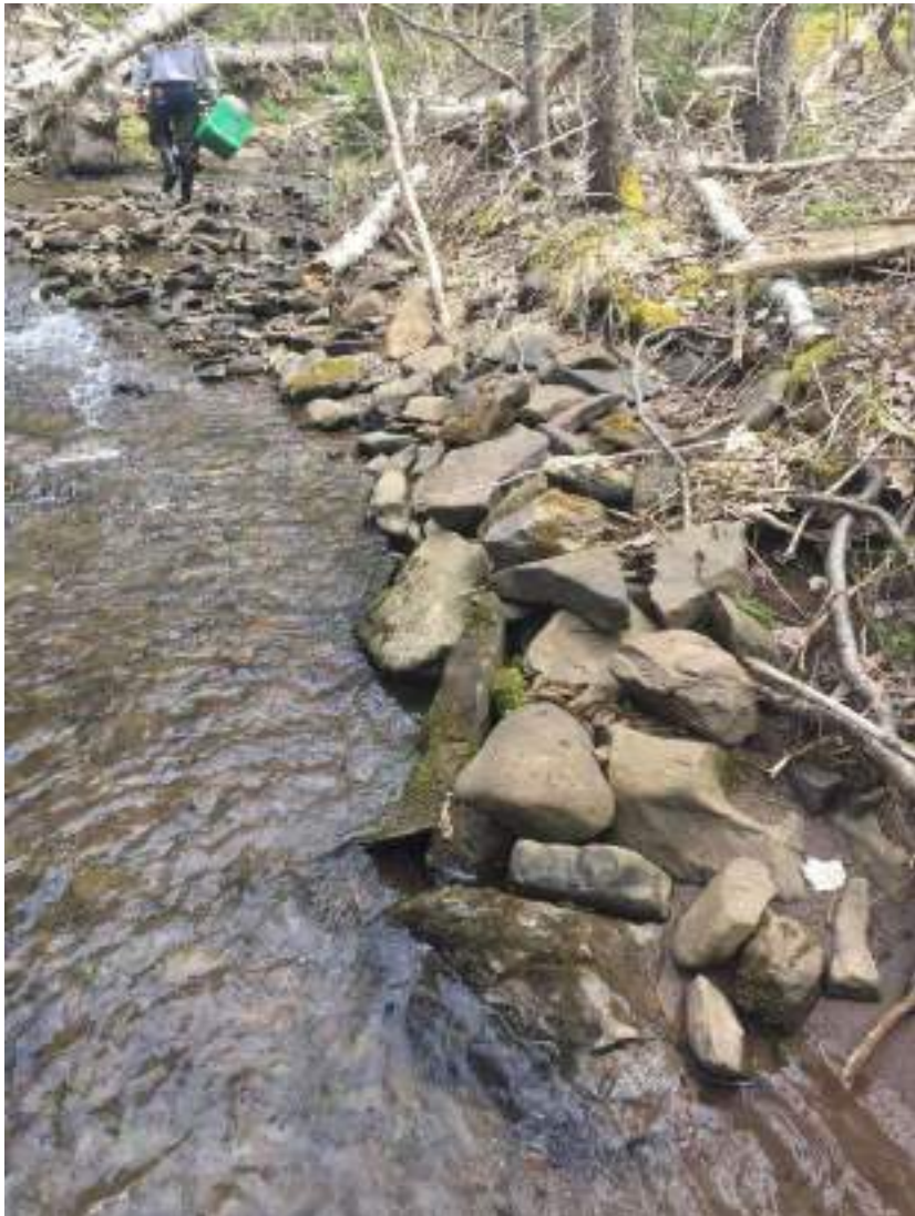
Figure 19. Bank stabilization - structure #9 downstream from the road.
