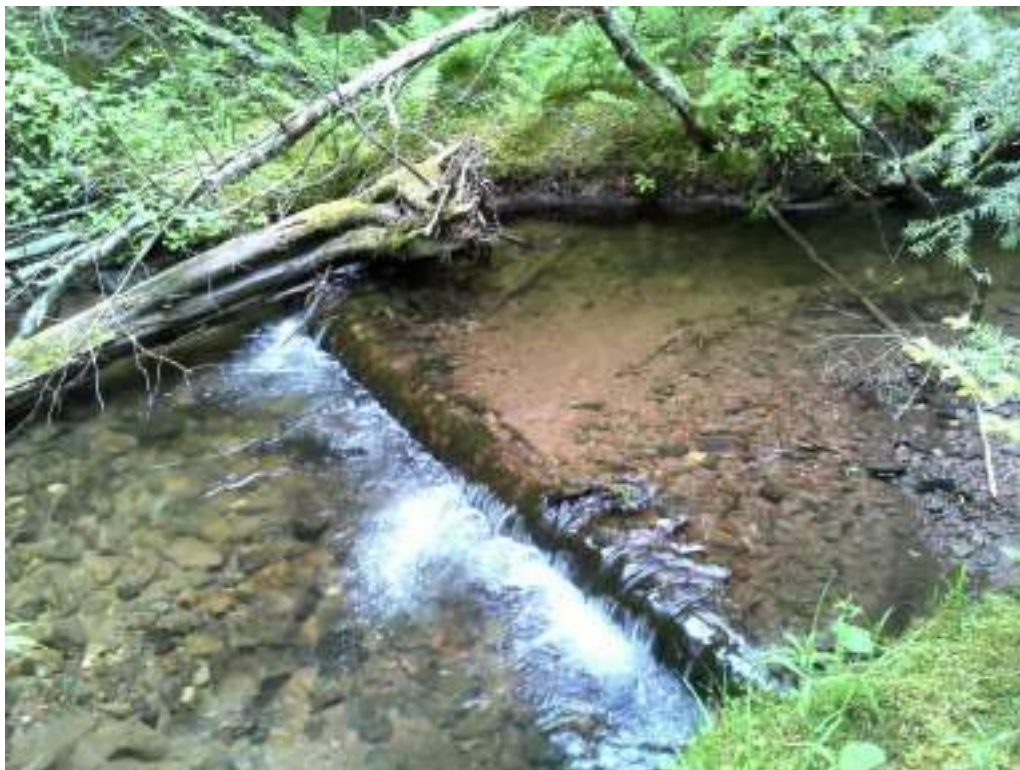
Figure 130. Diggerlog #36 - after picture of maintenance performed.
