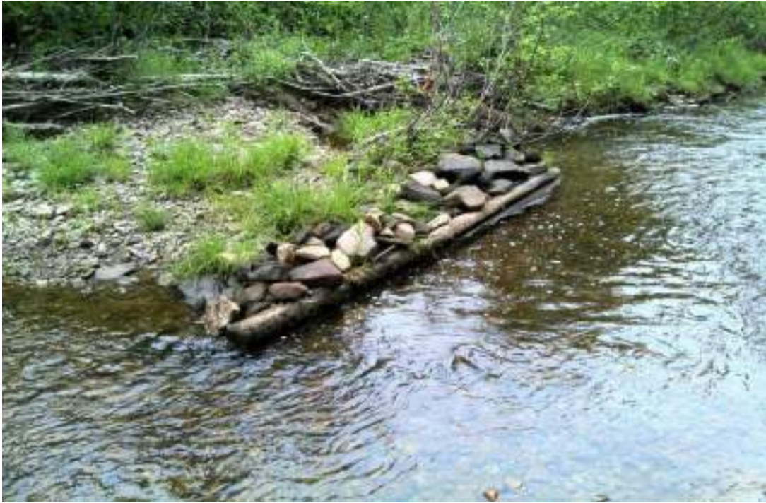
Figure 157. Deflector #10 - after picture of maintenance.
