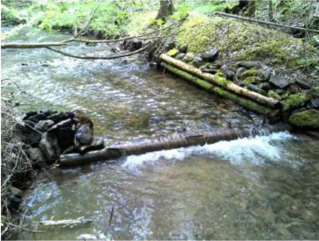
Figure 119. Diggerlog and deflector structure #25 - after picture of maintenance performed.
