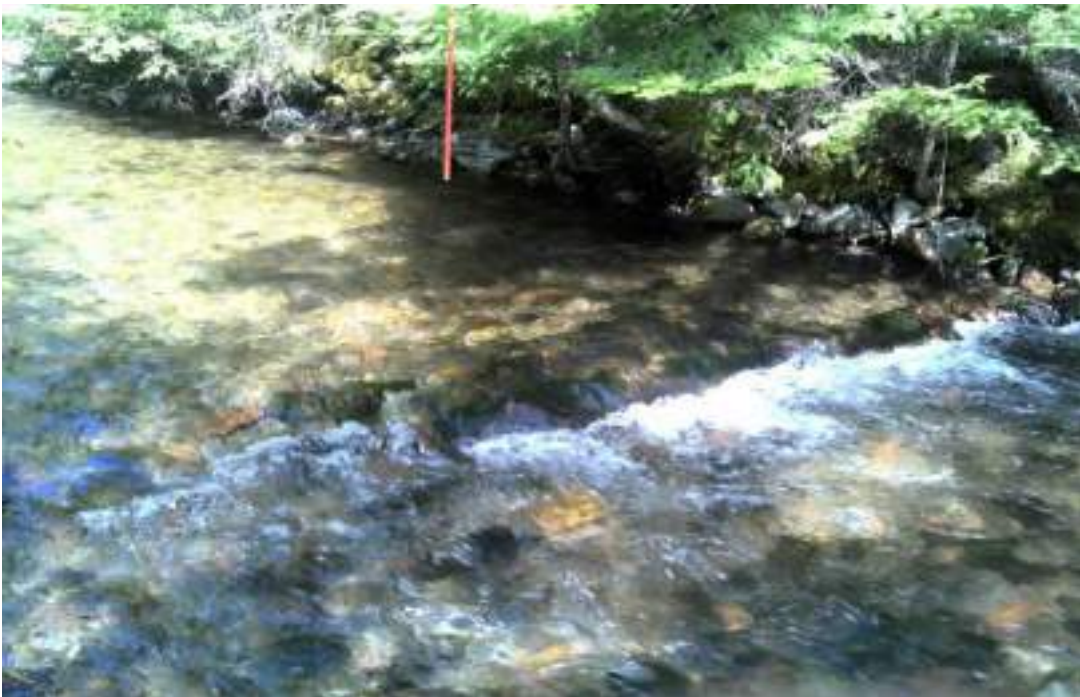
Figure 43. Diggerlog #16 - buried diggerlog. Before and after pictures show attempted maintenance on the structure.
