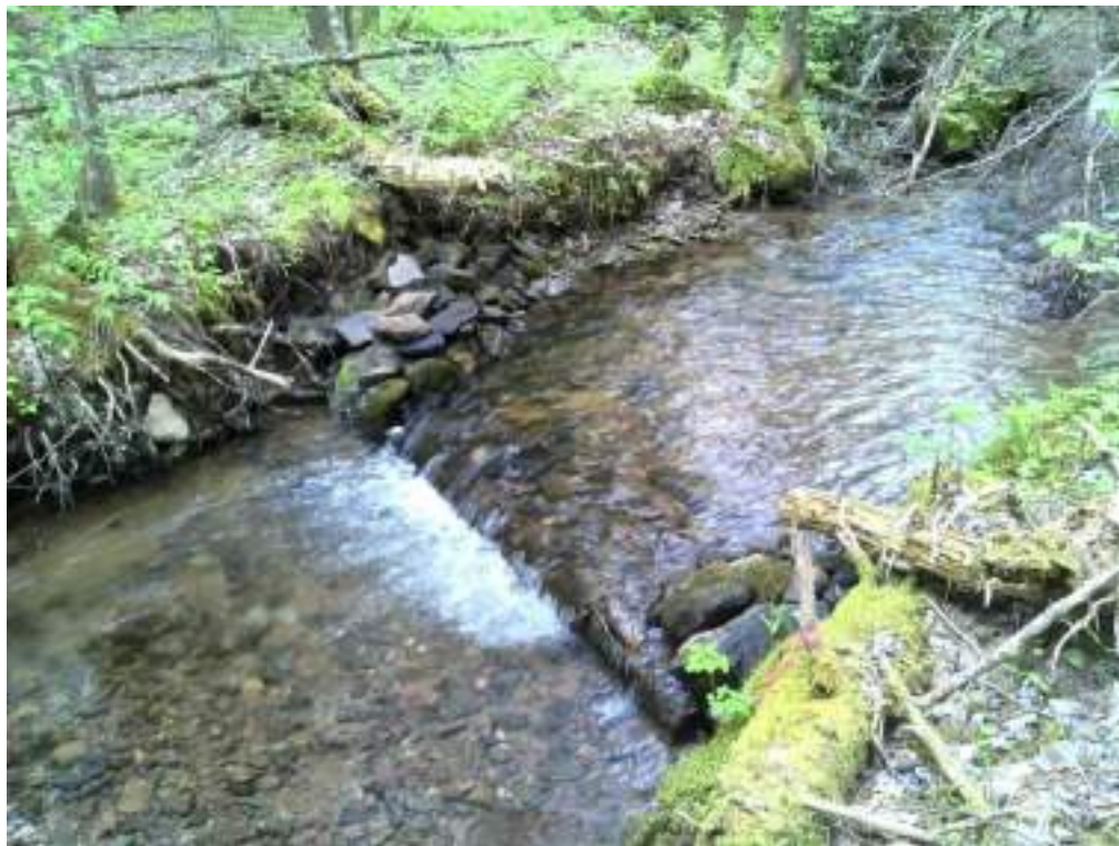
Figure 132. Diggerlog #38 - after picture of maintenance performed.
