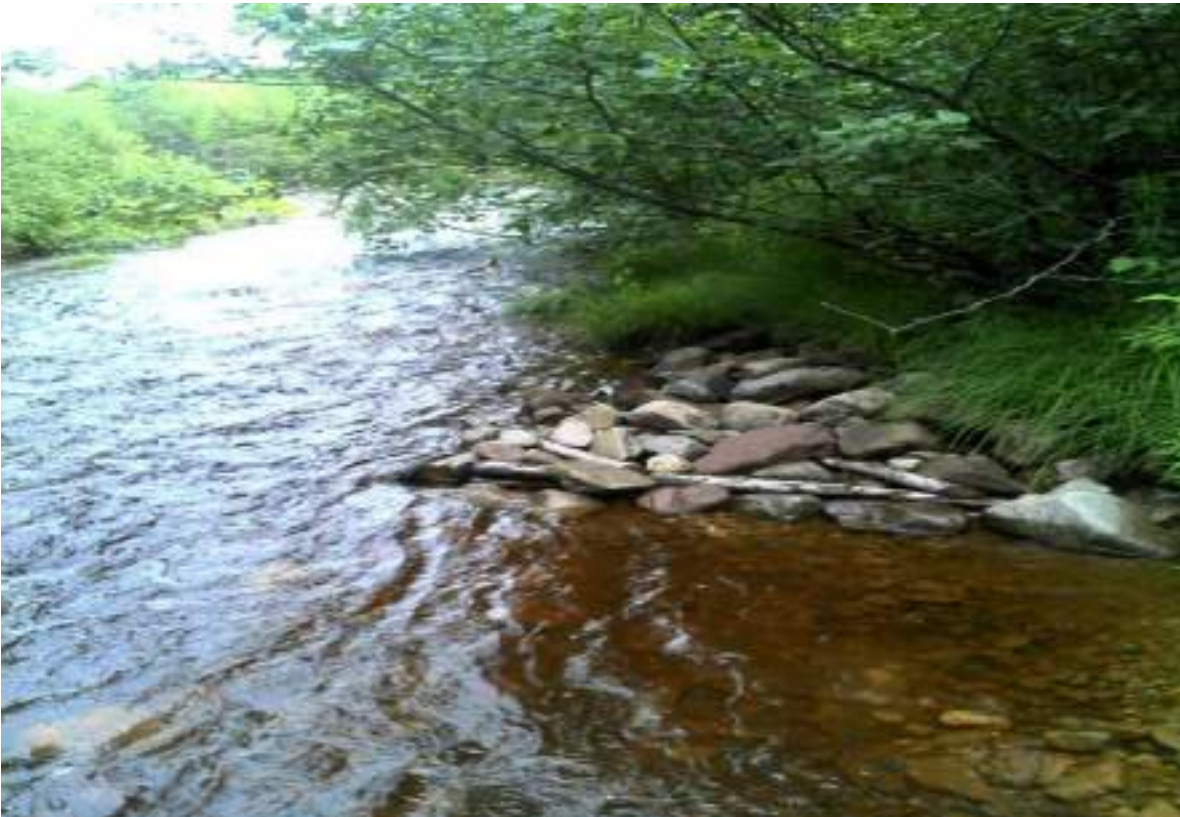
Figure 191. Structure #6 - before and after picture of completed maintenance.
