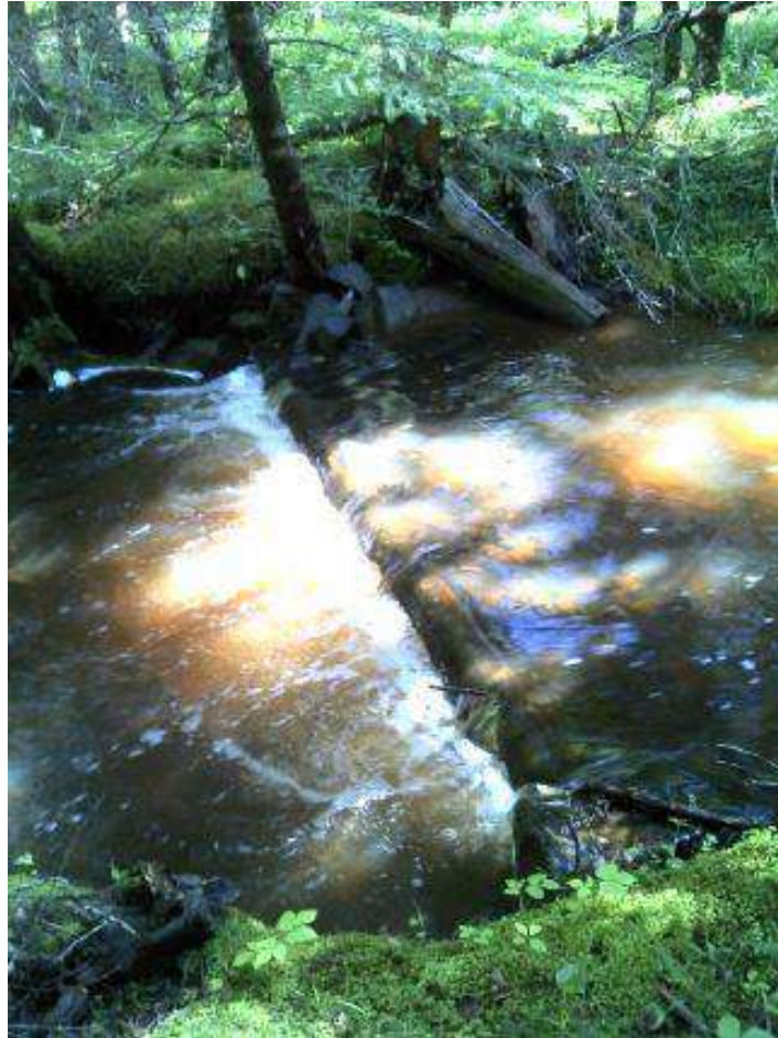
Figure 174. Structure #3 - After picture of the maintenance completed on a digger log.
