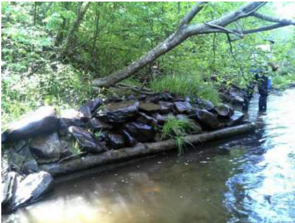
Figure 145. Deflector #8 - before and after picture of maintenance performed.
