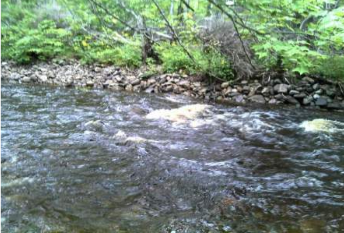
Figure 201. Structure #15 Bank Rock - before and after pictures of completed maintenance.
