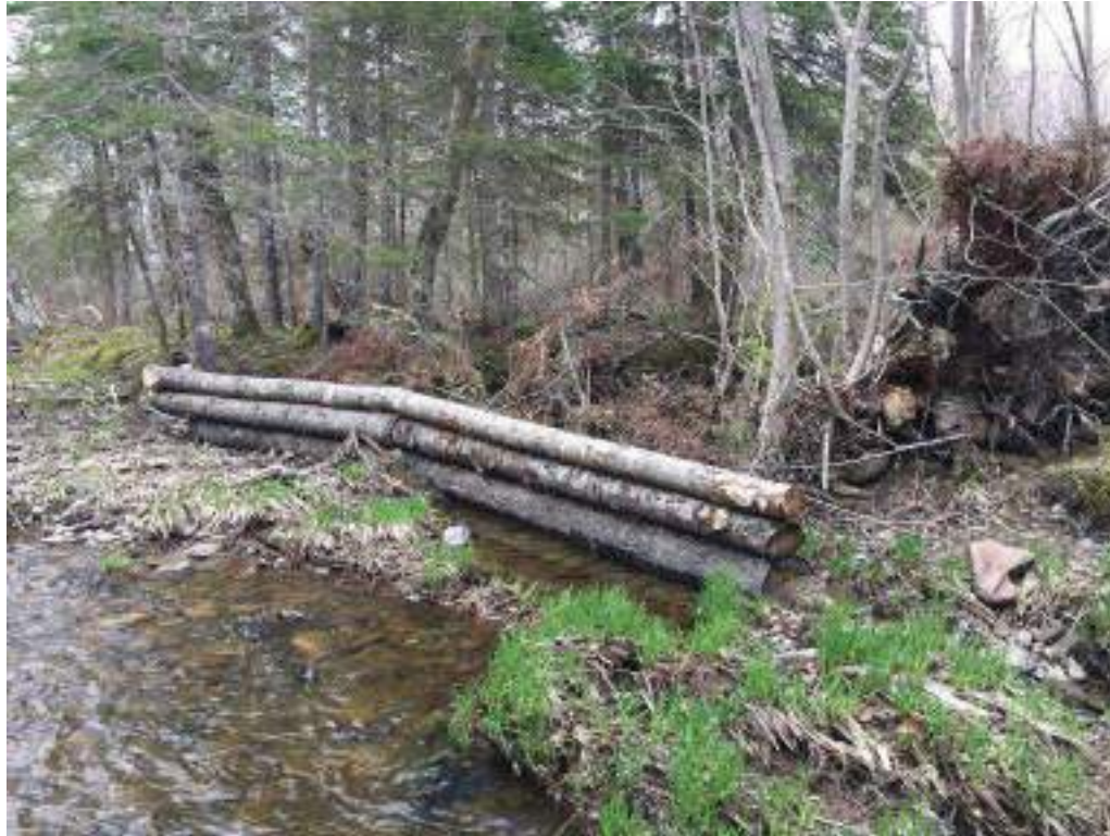
Figure 221. Structure #35 Channel Blocker - no maintenance required.
