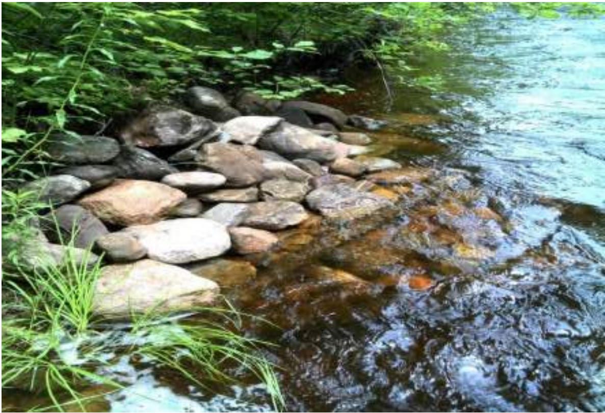
Figure 190. Structure #5 Deflector - before and after pictures of completed maintenance.
