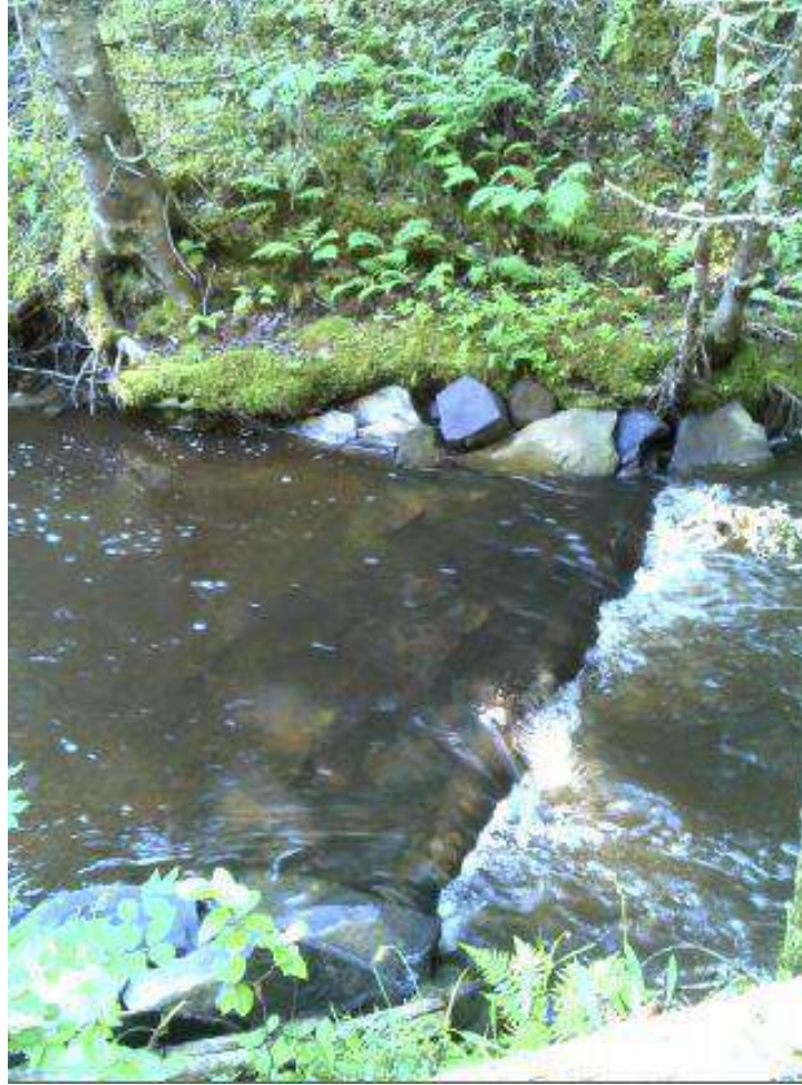
Figure 177. Structure #6 - After picture of the maintenance completed on a digger log.
