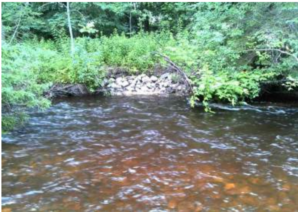
Figure 187. Structure #2 Bank Rock - before and after pictures of the completed maintenance.
