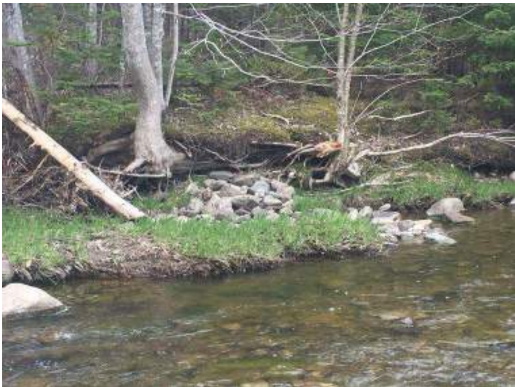
Figure 237. Structure #51 Bank Rock - no maintenance required.
