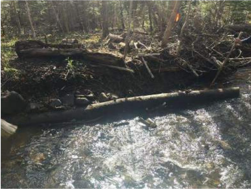
Figure 66. Structure #18 - Before picture of a deflector structure. No after picture of maintenance
