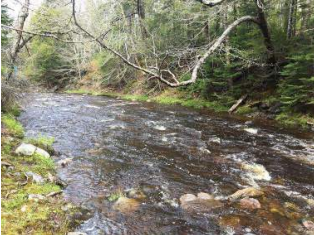
Figure 249. Structure #63 Deflector - missing and requires a rebuild.
