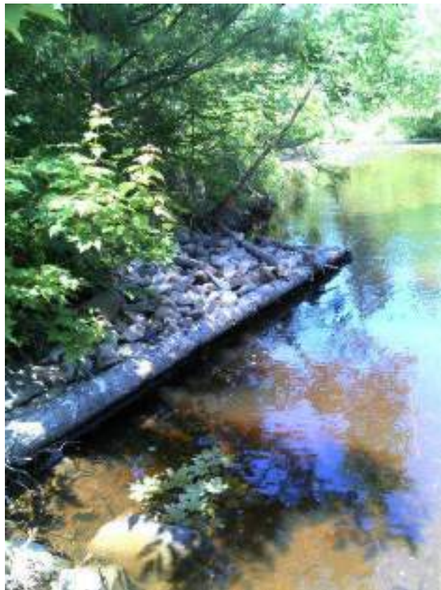
Figure 224. Structure #38 Deflector - before and after picture of completed maintenance.
