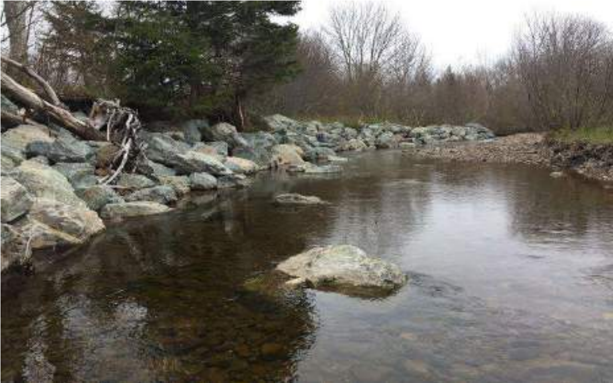
Figure 195. Continuation of structure #9 - Armour stone - bank stabilization.
