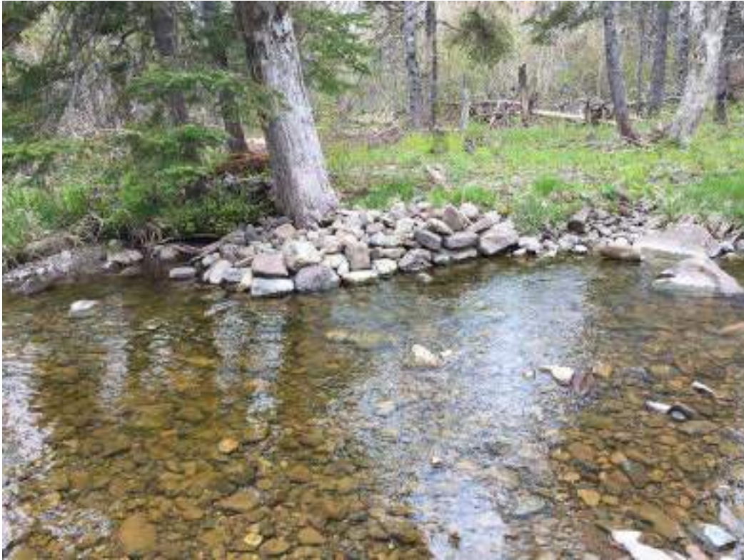
Figure 226. Structure #40 Bank Rock - no maintenance required.
