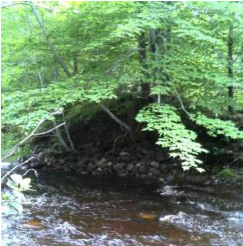
Figure 208. Structure #22 Bank Rock - before and after picture of completed maintenance.
