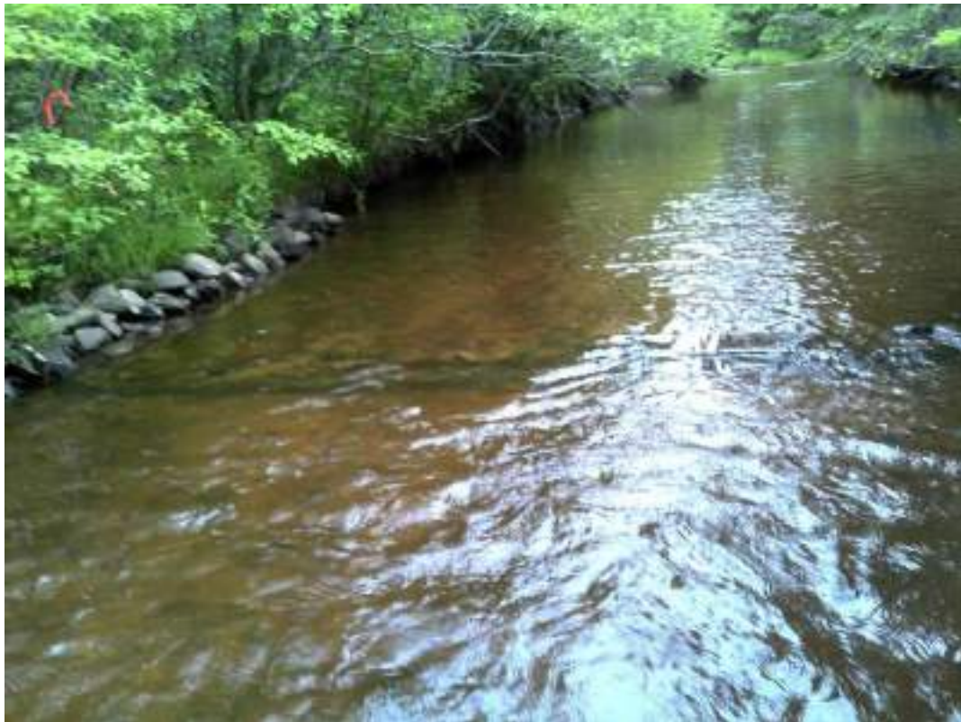
Figure 156. Bank rock/stabilization #9 - after picture of maintenance performed. There is also an old diggerlog log here that is buried into the substrate.
