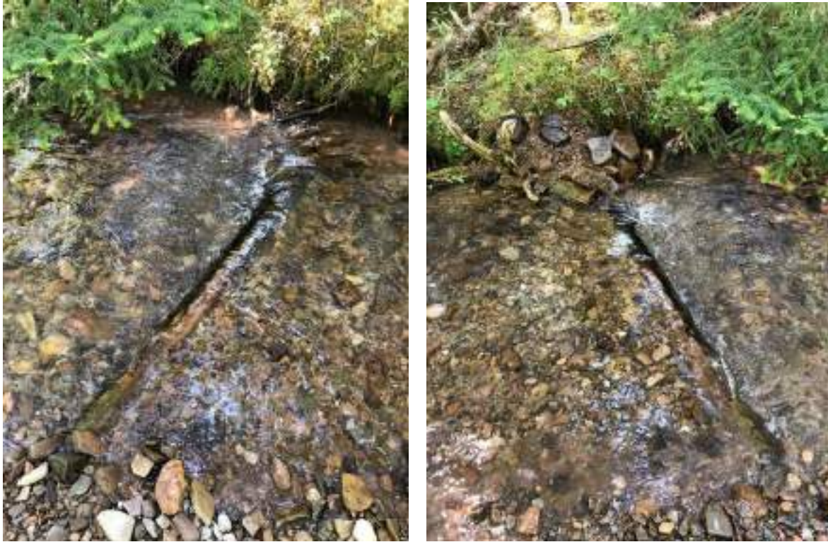
Figure 135. Before and after picture of the maintenance performed on digger log #41.
