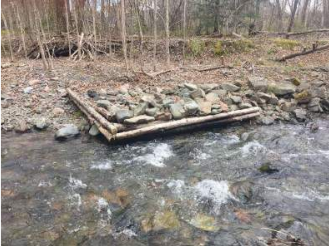
Figure 33. Deflector #6 - before and after picture of maintenance performed.
