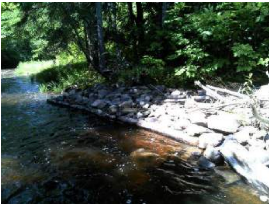
Figure 223. Structure #37 Deflector - before and after pictures of completed maintenance.
