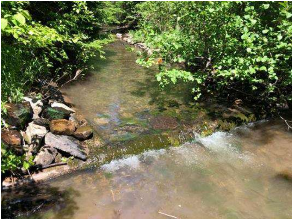
Figure 84. Diggerlog structure #9 - downstream side of Smithville Road.
