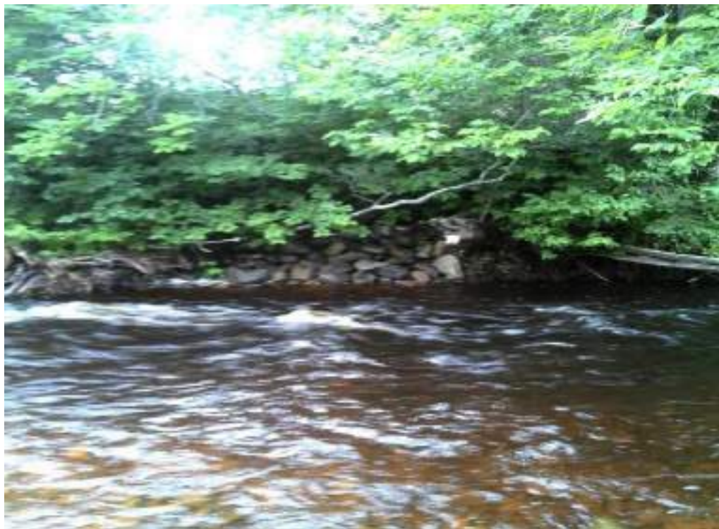
Figure 188. Structure #3 Bank Rock - before and after pictures of completed maintenance.
