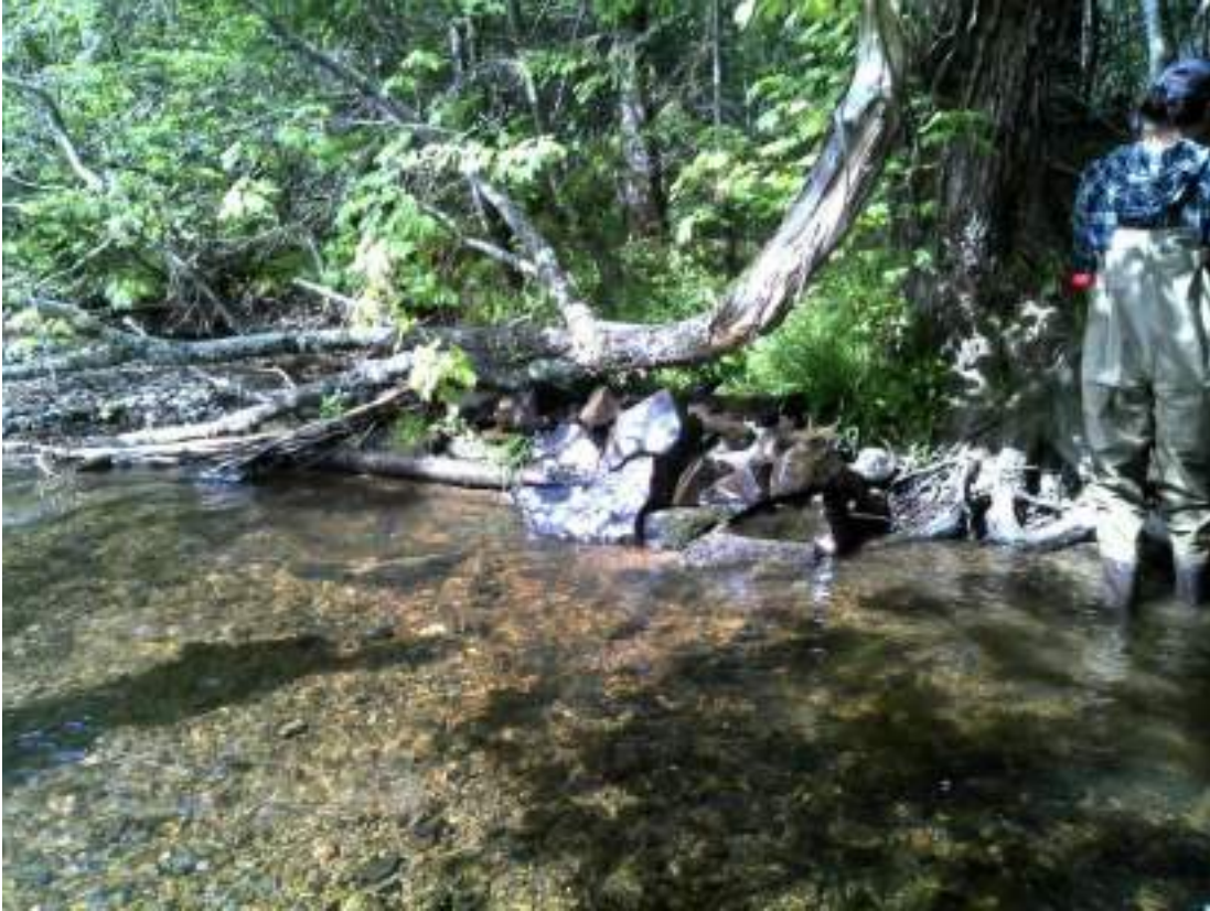
Figure 146. Deflector #9 - after picture of maintenance performed.
