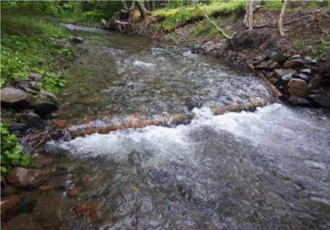
Figure 32. Diggerlog #5 - before and after pictures of maintenance.
