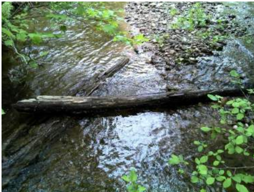
Figure 167. Diggerlog #6 - this structure needs to be replaced.
