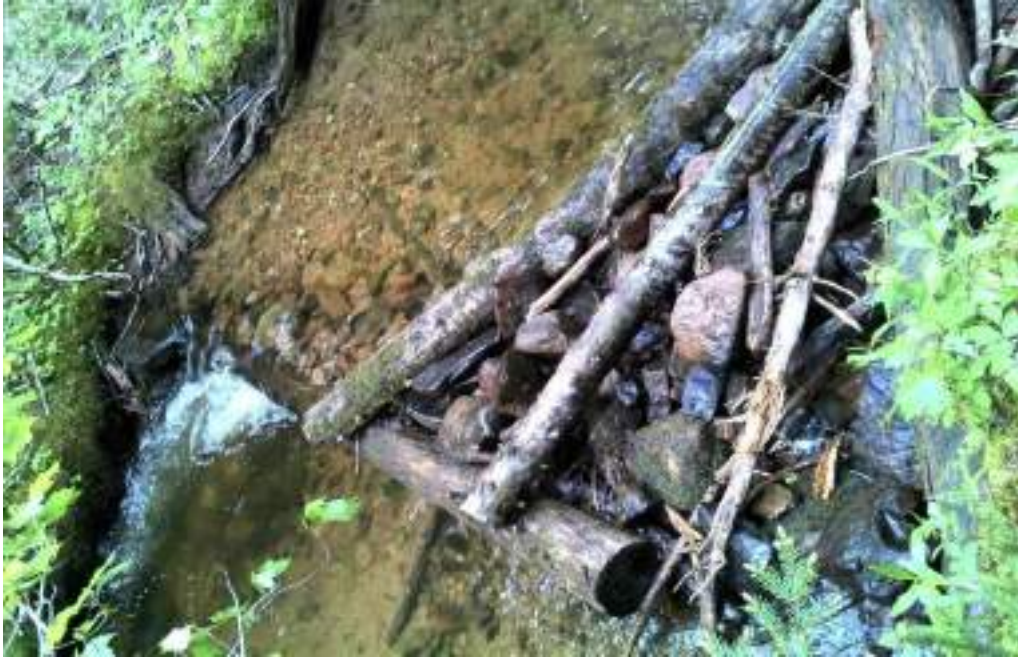
Figure 168. Diggerlog #7 - after picture of the maintenance performed. Debris materials were added to the upstream side of the log to help direct waterflow.
