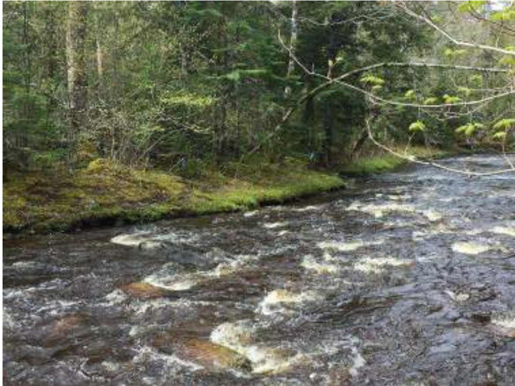
Figure 247. Structure #61 Deflector - missing and requires a rebuild.
