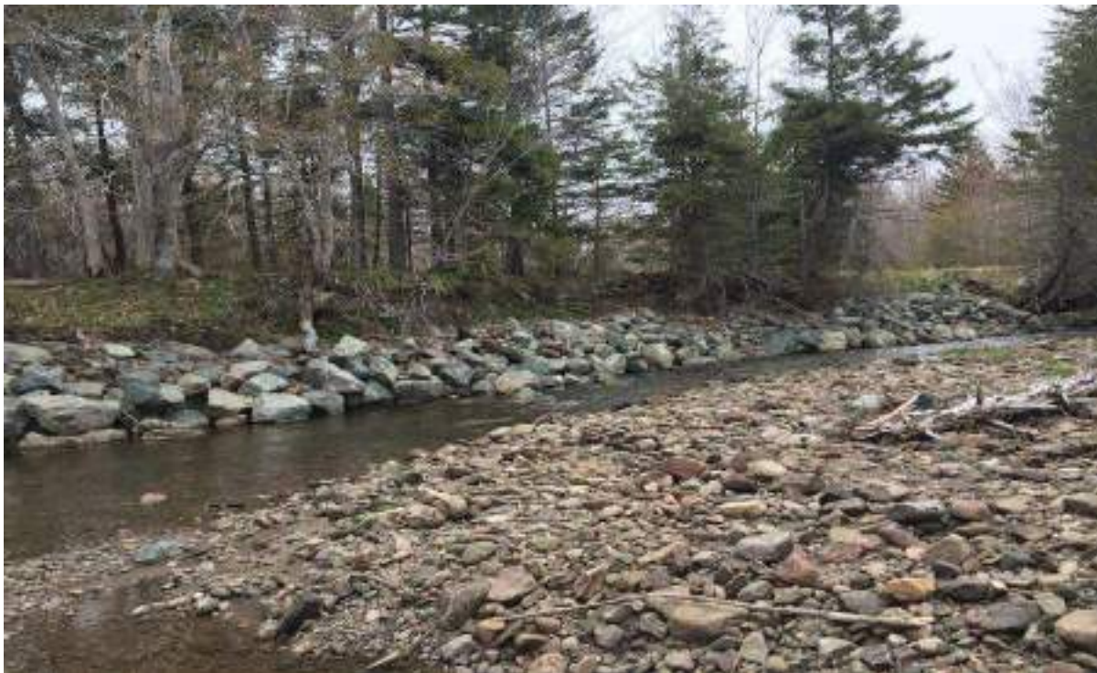
Figure 204. Structure #18 Armour Stone - bank stabilization.
