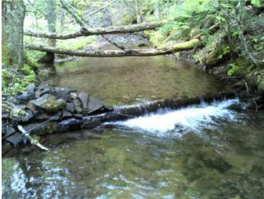
Figure 133. Diggerlog #39 - after picture of maintenance performed.
