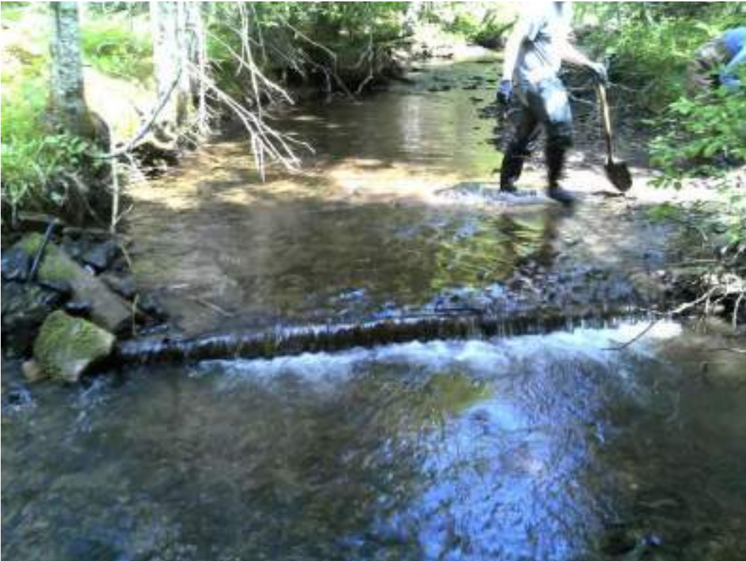
Figure 80. Diggerlog structure #5 upstream from the Trans Canada Trail.
