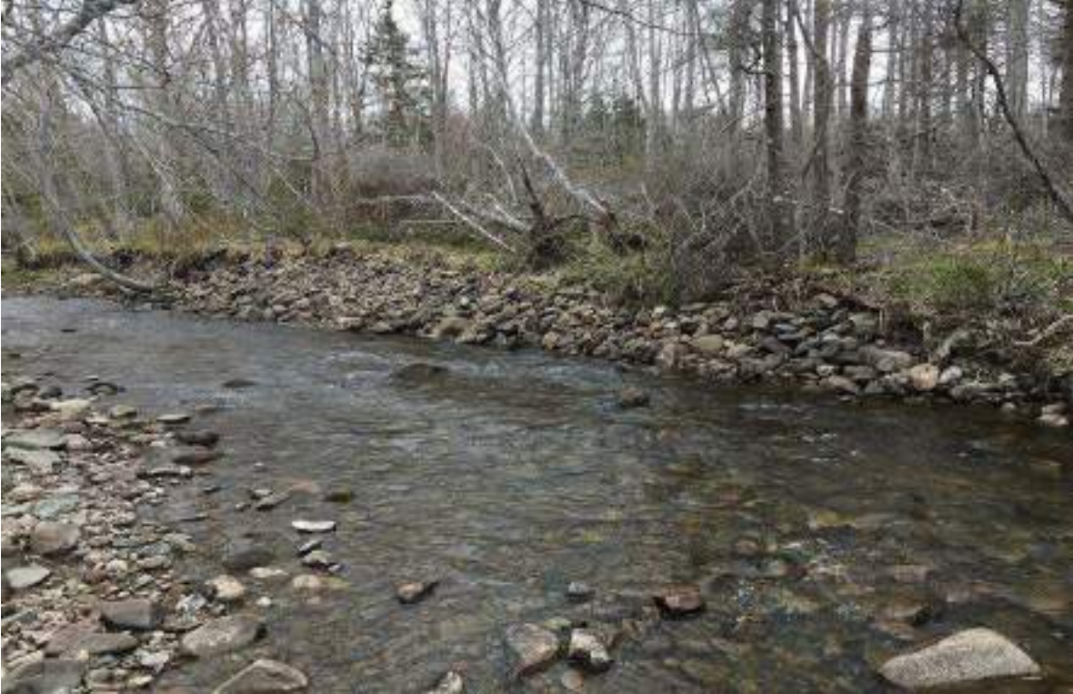
Figure 200. Structure #14 Armour Stone - bank stabilization.
