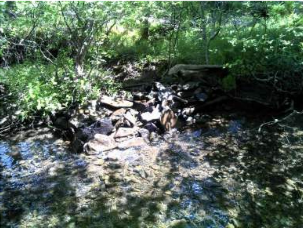
Figure 79. Deflector structure #4 upstream from the Trans Canada Trail..
