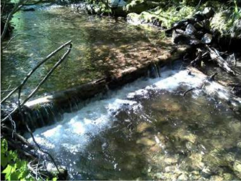
Figure 103. Diggerlog #9 - after picture of maintenance performed.
