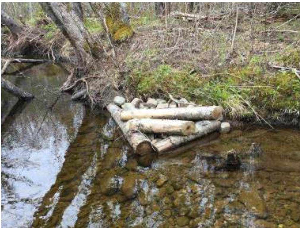
Figure 222. Structure #36 Deflector - didn't require any maintenance.
