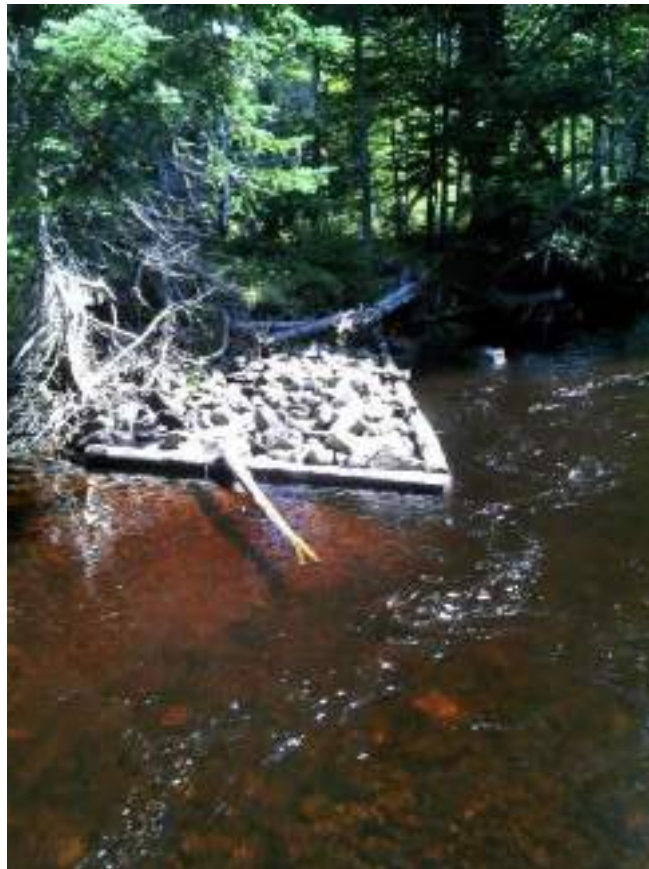
Figure 216. Structure #30 Deflector - before and after picture of completed maintenance.
