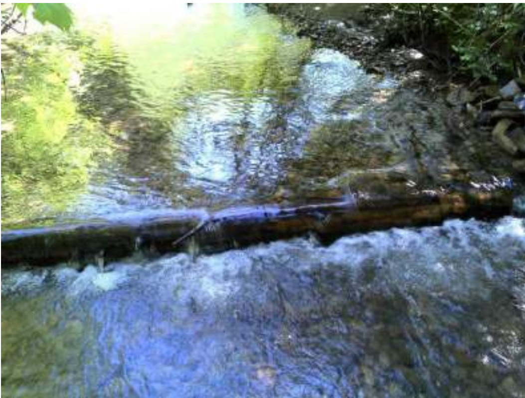
Figure 96. Diggerlog #2 - after photo of maintenance.
