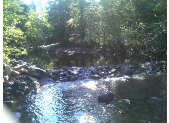
16. Rock Sill and Rock Deflector, N45.90171° W61.35584°
