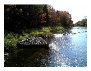
Structure #4. Double Deflector w/ #5 - 6x3 meters, 3 tiers filled in with rock
