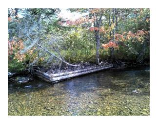
Structure #13. Deflector - 6x3 meters, 3 tiers filled in with rock. Big logs were used.
