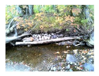
Structure #22. Deflector – 4x2 meters, 2 tiers filled with rock
