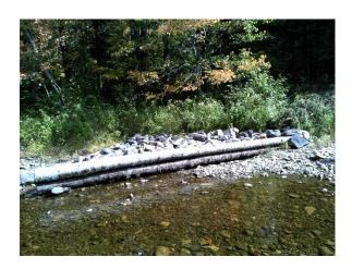
Structure #16. Deflector - 6x3 meters, 3 tiers filled in with rock. Brush was placed below.
