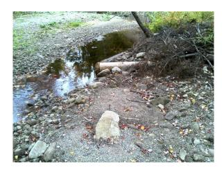
**Structure #21.** Bank Stabilization – log with rock used to protect the bank
