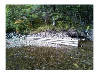
**Structure #11.** Bank Stabilization – approximately 25 ft long, filled in with rock to the bank.
