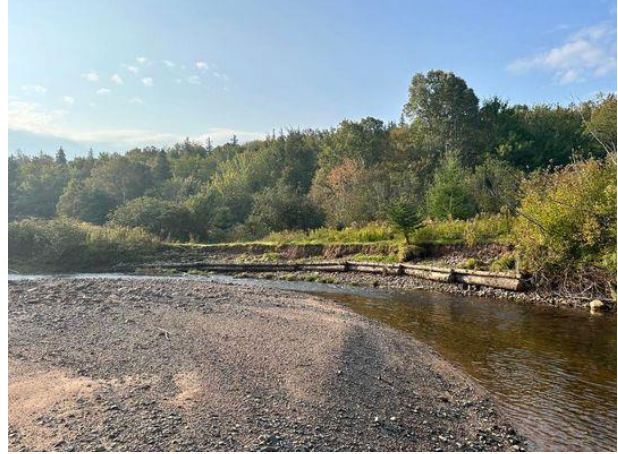
Before and after photo of a bank stabilization structure, built logs and hand rock, 2023.
