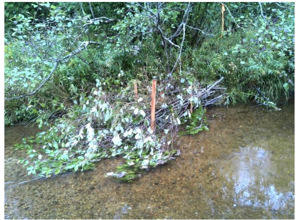
Figure 18. Structure #11 - brush bundle made with alders.
