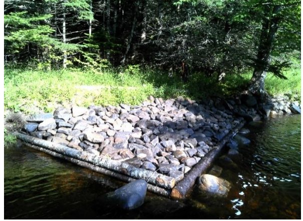
Figure 50. Structure #4 - deflector 6x3 meters, two tier.
