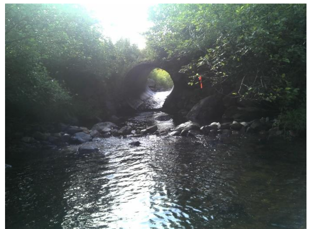
Figure 15. Structure #8 - rock sill just below the culvert
