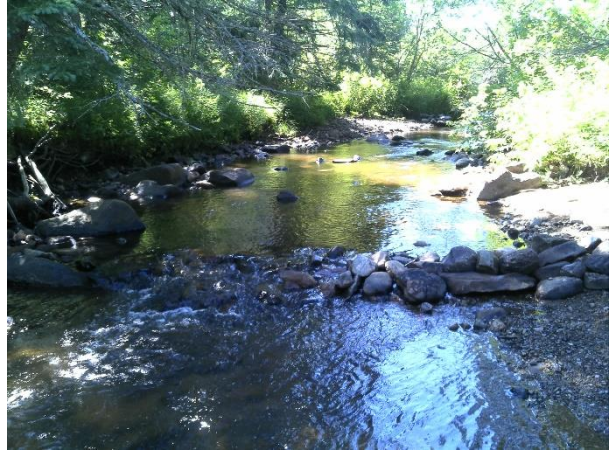
Figure 8. Structure #1 - rock sill. This is the furthest structure downstream.
