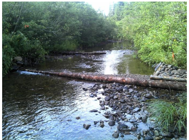
Figure 10. Structure #3 - digger log with deflector.
