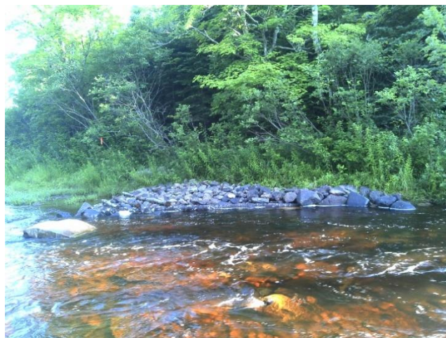
Figure 49. Structure #3 - deflector 6x3 meters, two tier.
