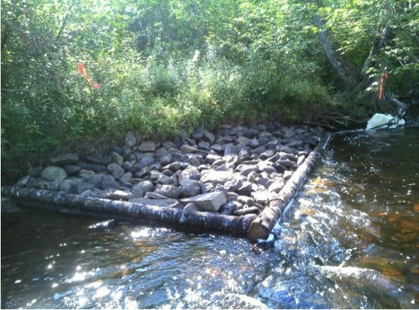
Figure 55. Structure #7 - deflector 6x3 meters, two tier.
