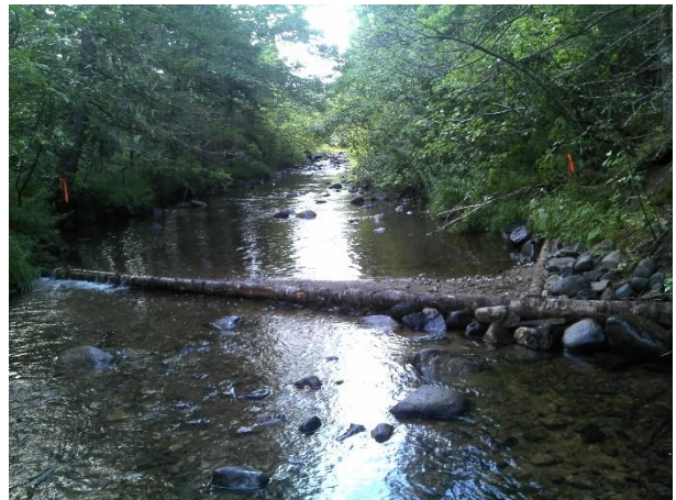
Figure 12. Structure #5 - digger log with deflector.
