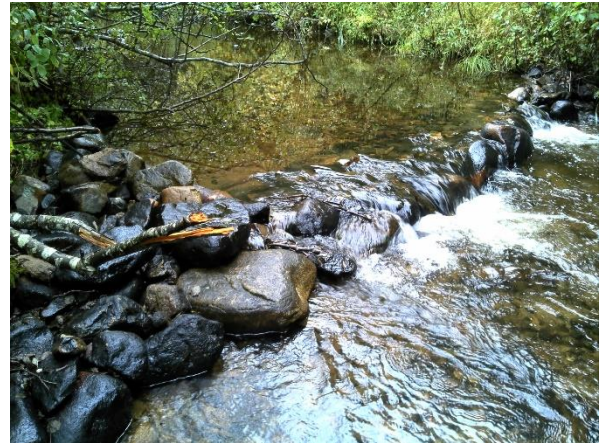
Figure 27. Structure #20 - rock sill with a deflector.
