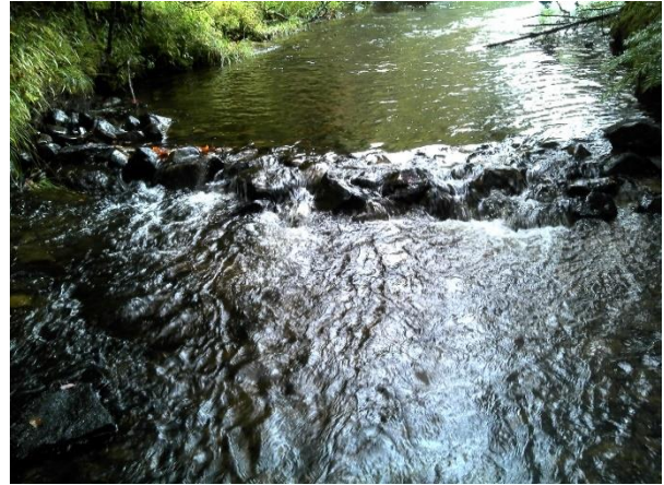
Figure 41. Structure #34 - rock sill.
