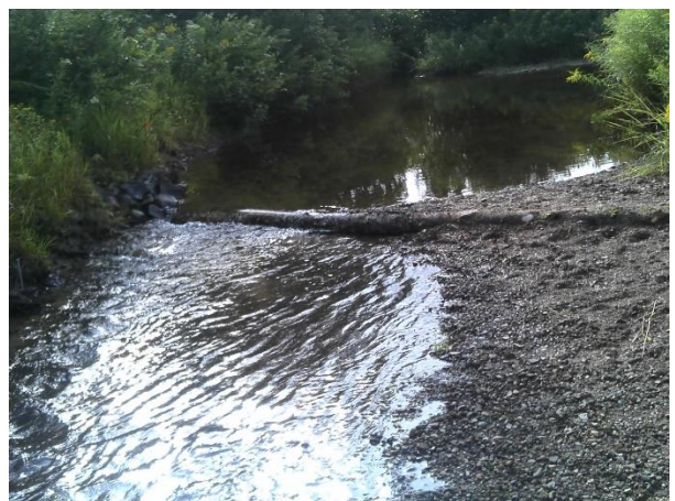
Figure 16. Structure #9 - digger log. This is the first structure installed upstream from the road.
