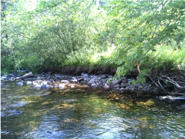
Figure 54. Structure #8 - deflector 6x3 meters, two tier.
