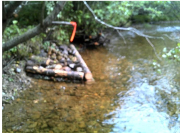
Figure 29. Structure #22 - deflector.
