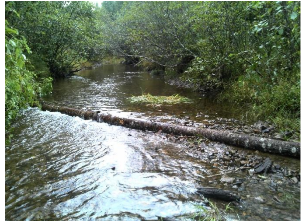
Figure 28. Structure #21 - digger log.
