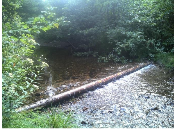
Figure 23. Structure #16 - digger log.
