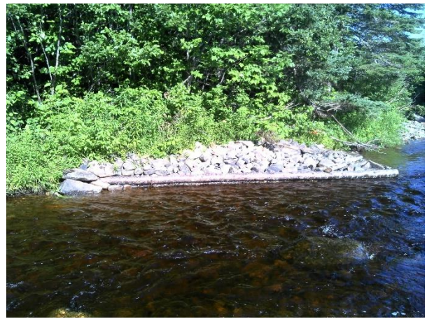
Figure 48. Structure #2 - deflector 6x3 meters, two tier.
