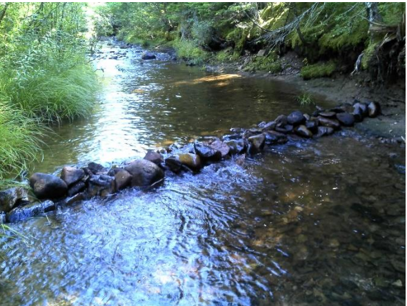
Figure 37. Structure #30 - rock sill.
