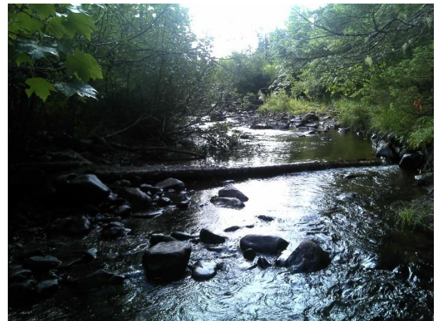
Figure 13. Structure #6 - digger log with deflector.
