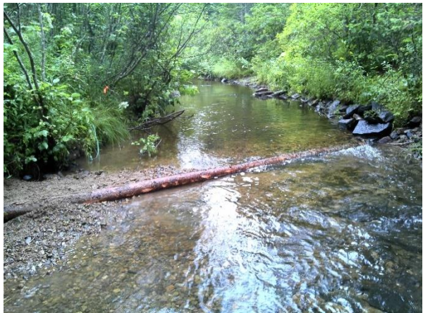
Figure 21. Structure #14 - digger log.
