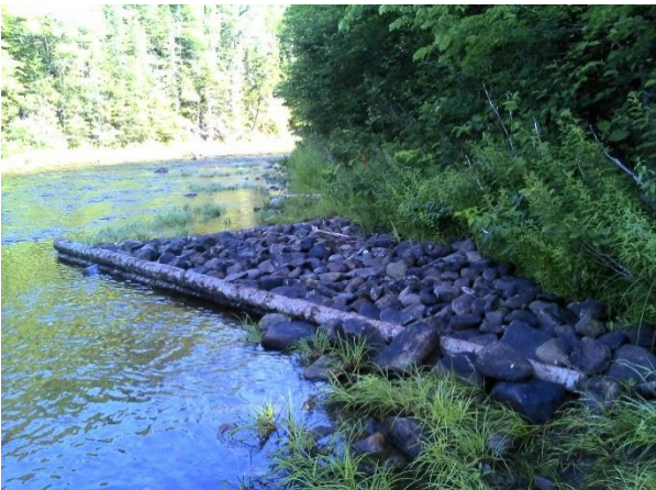
Figure 54. Structure #8 - deflector 6x3 meters, two tier.
