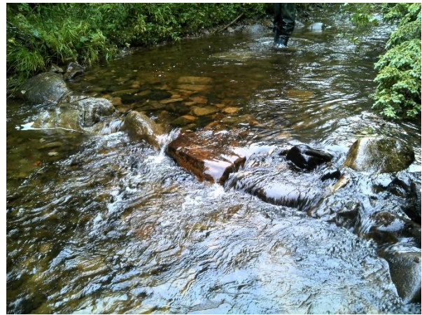
Figure 42. Structure #35 - rock sill.
