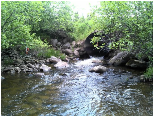
Figure 15. Structure #8 - rock sill just below the culvert
