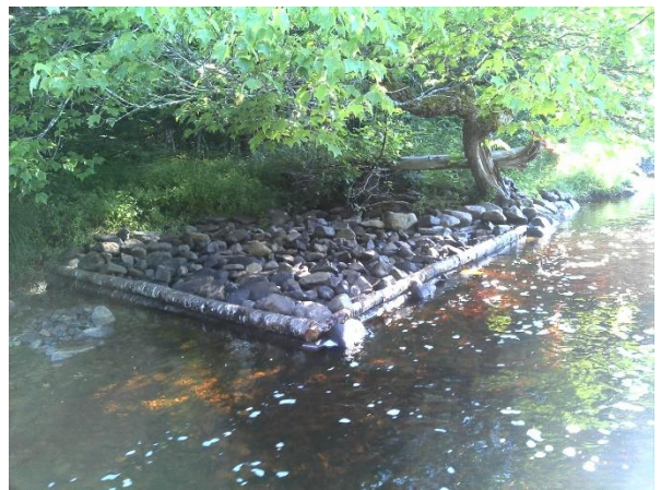
Figure 51. Structure #5 - deflector 6x3 meters, two tier.
