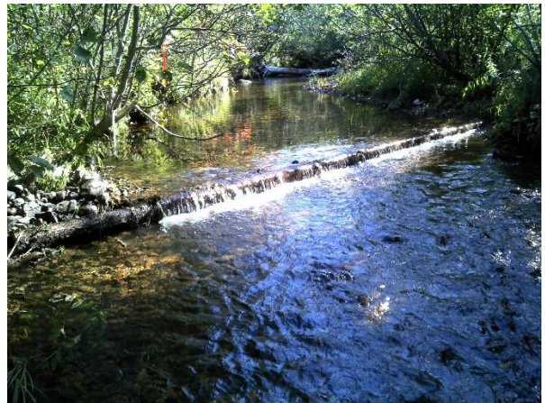
Figure 30. Structure #23 - digger log.
