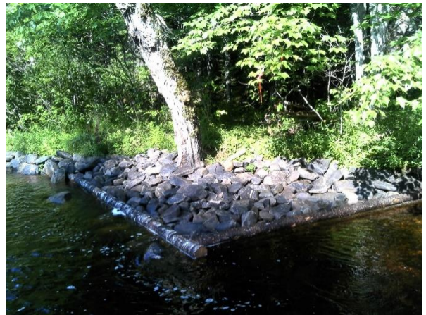
Figure 52. Structure #6 - deflector 6x3 meters, two tier.
