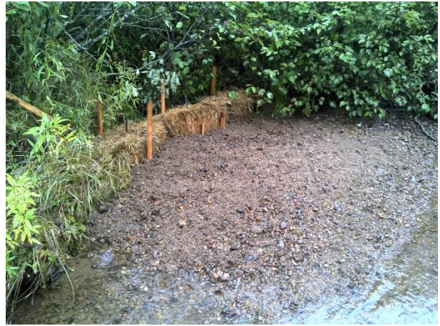
Figure 17. Structure #10 - brush bundle made with hay bails.
