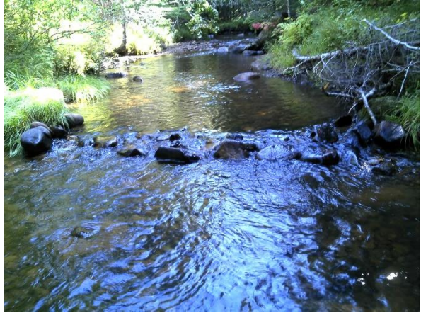
Figure 38. Structure #31 - rock sill.
