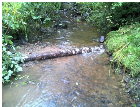
Figure 44. Structure #37 - digger log on cold water tributary.
