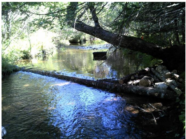
Figure 34. Structure #27 - digger log with deflector.
