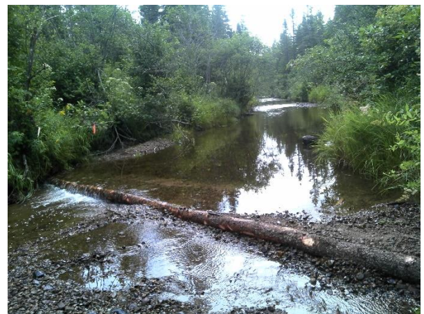
Figure 19. Structure #12 - digger log.
