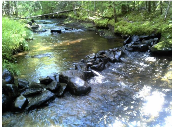
Figure 40. Structure #33 - rock sill.
