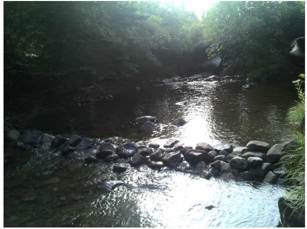
Figure 14. Structure #7 - rock sill.
