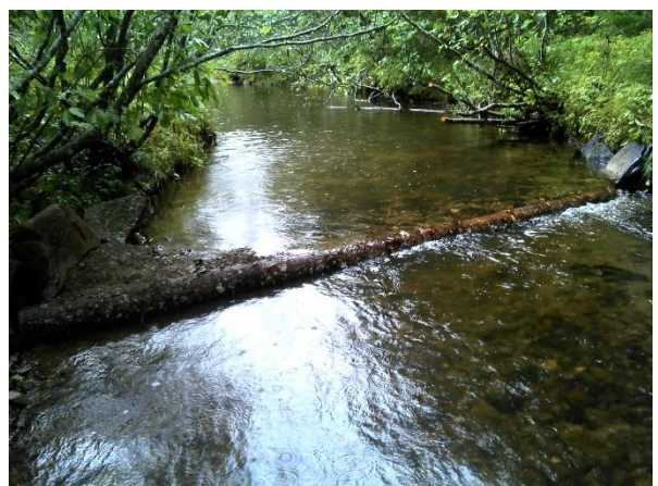
Figure 31. Structure #24 - digger log.
