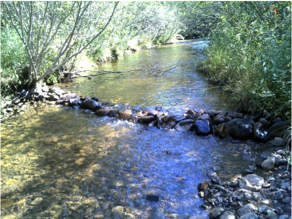
Figure 36. Structure #29 - rock sill.
