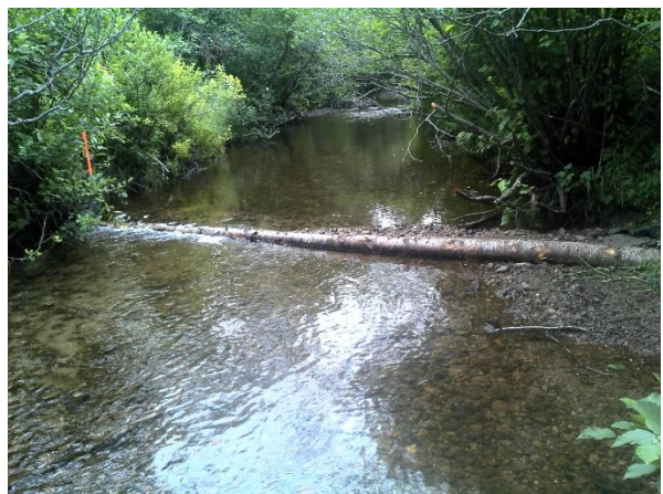
Figure 22. Structure #15 - digger log.
