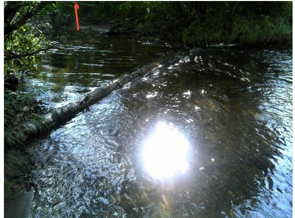
Figure 24. Structure #17 - digger log.
