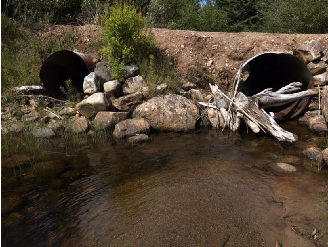
Figure 5: Barrier culvert - lower MacLeod Brook
