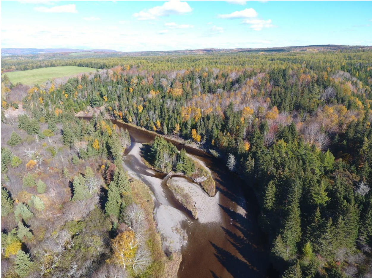
Figure 4: Severely over-widened and split channel.
