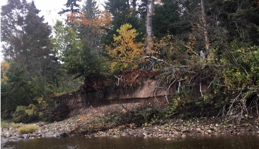
Figure 2: Typical stream bank erosion on lower section of Southwest Mabou
