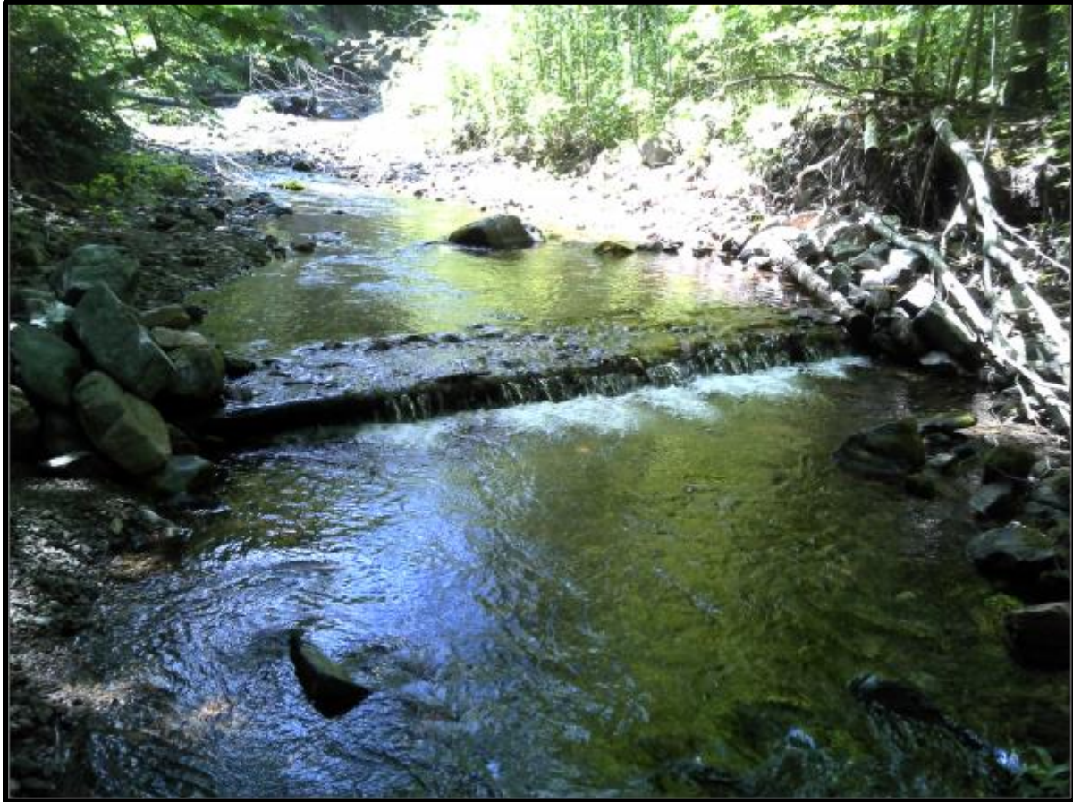
Figure 34. Maintained digger log and deflector structure.
