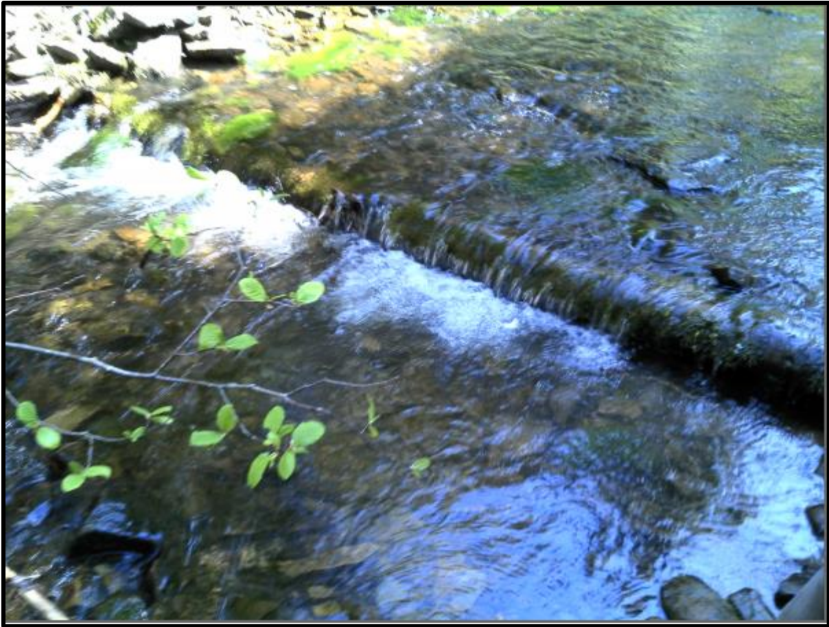
Figure 18. Digger Log and Deflector on the Glendyre River.
