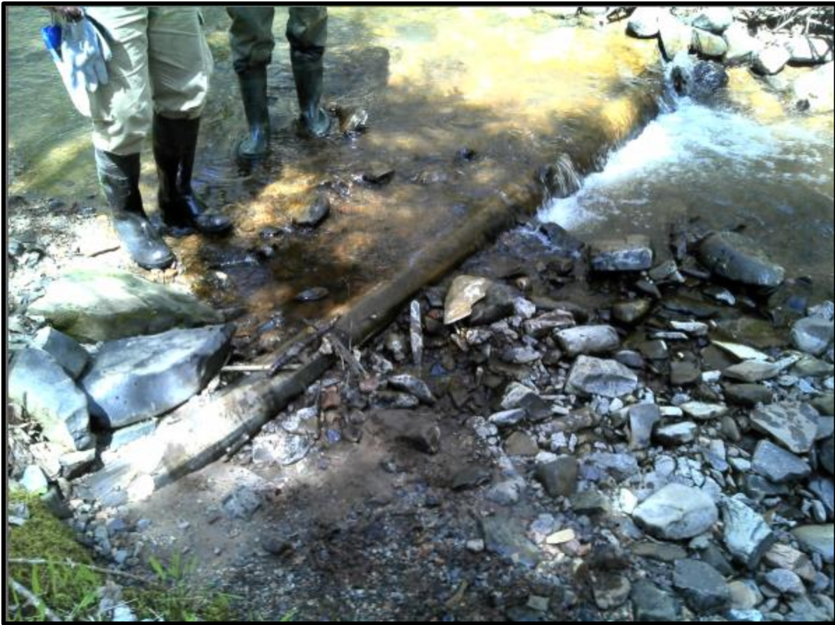
Figure 60. Digger Log structure for waypoint 53.
