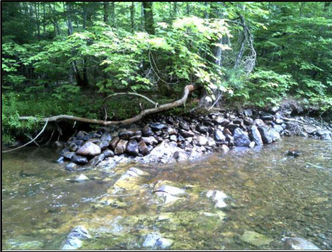
Figure 140. After picture of deflector at waypoint 183.
