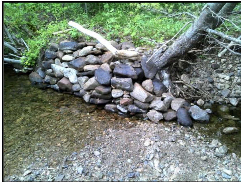
Figure 152. After picture of two tier bank rock at way point 213.
