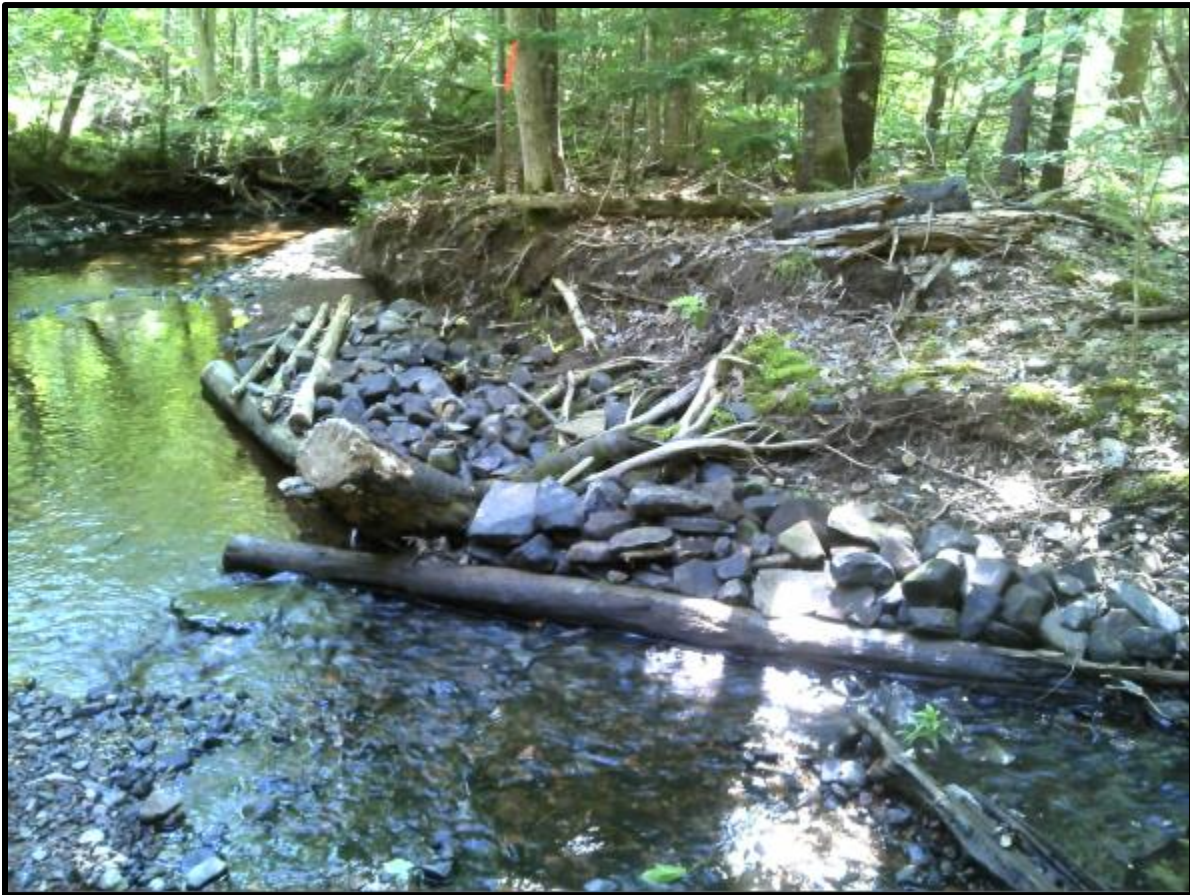
Figure 54. Deflector/Bank log structure at waypoint 42.
