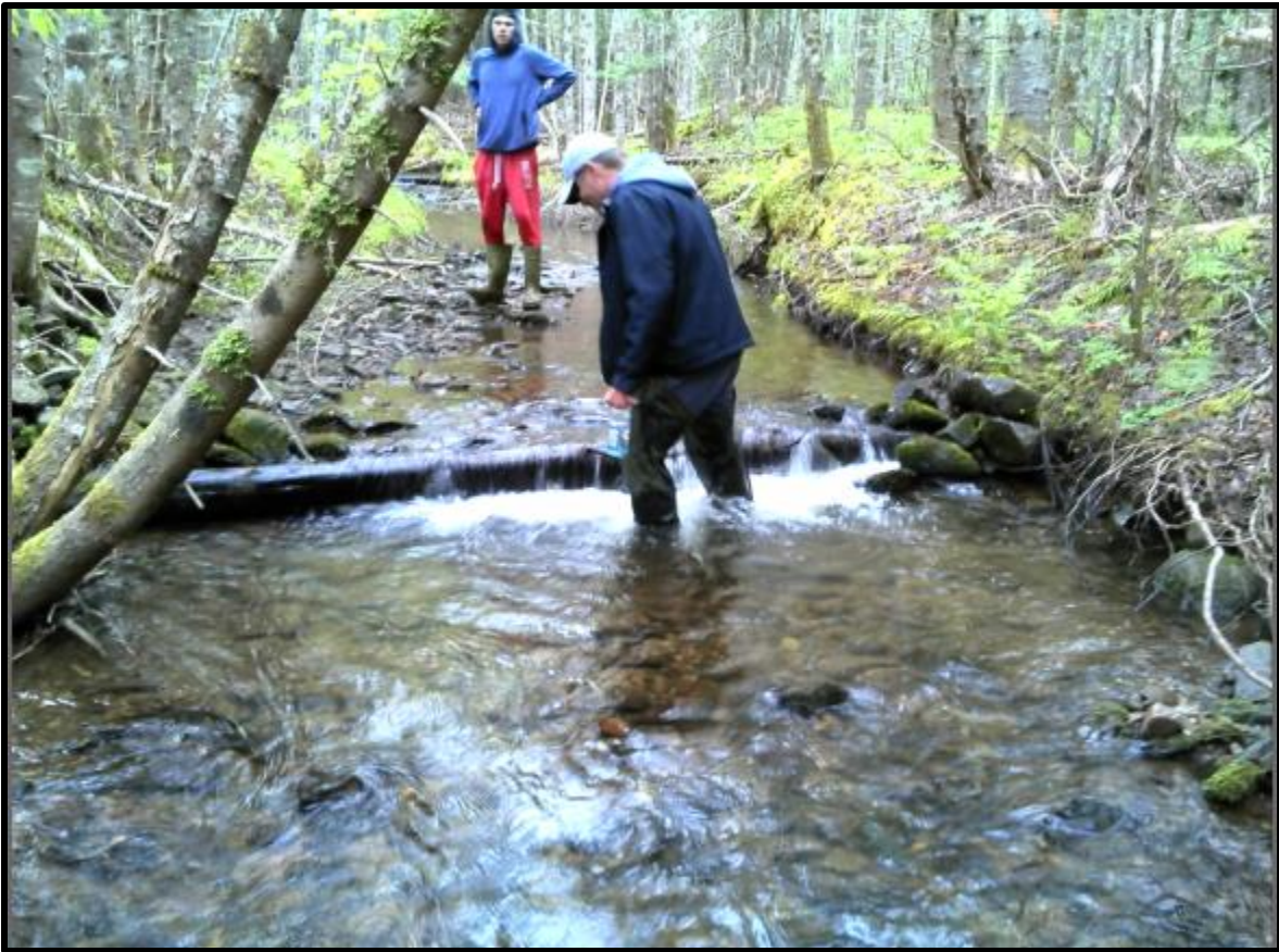
Figure 114. Digger Log and Deflector at waypoint 100.
