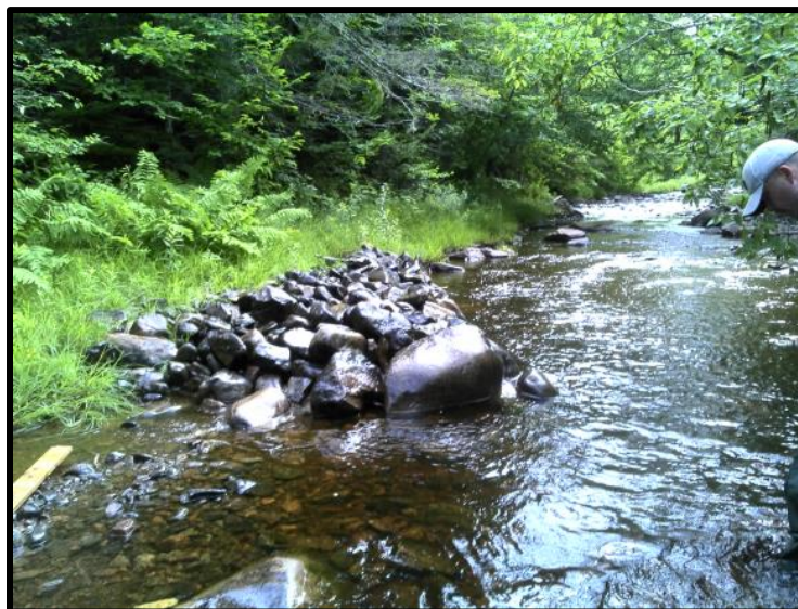
Figure 135. After picture of deflector at way point 176.
