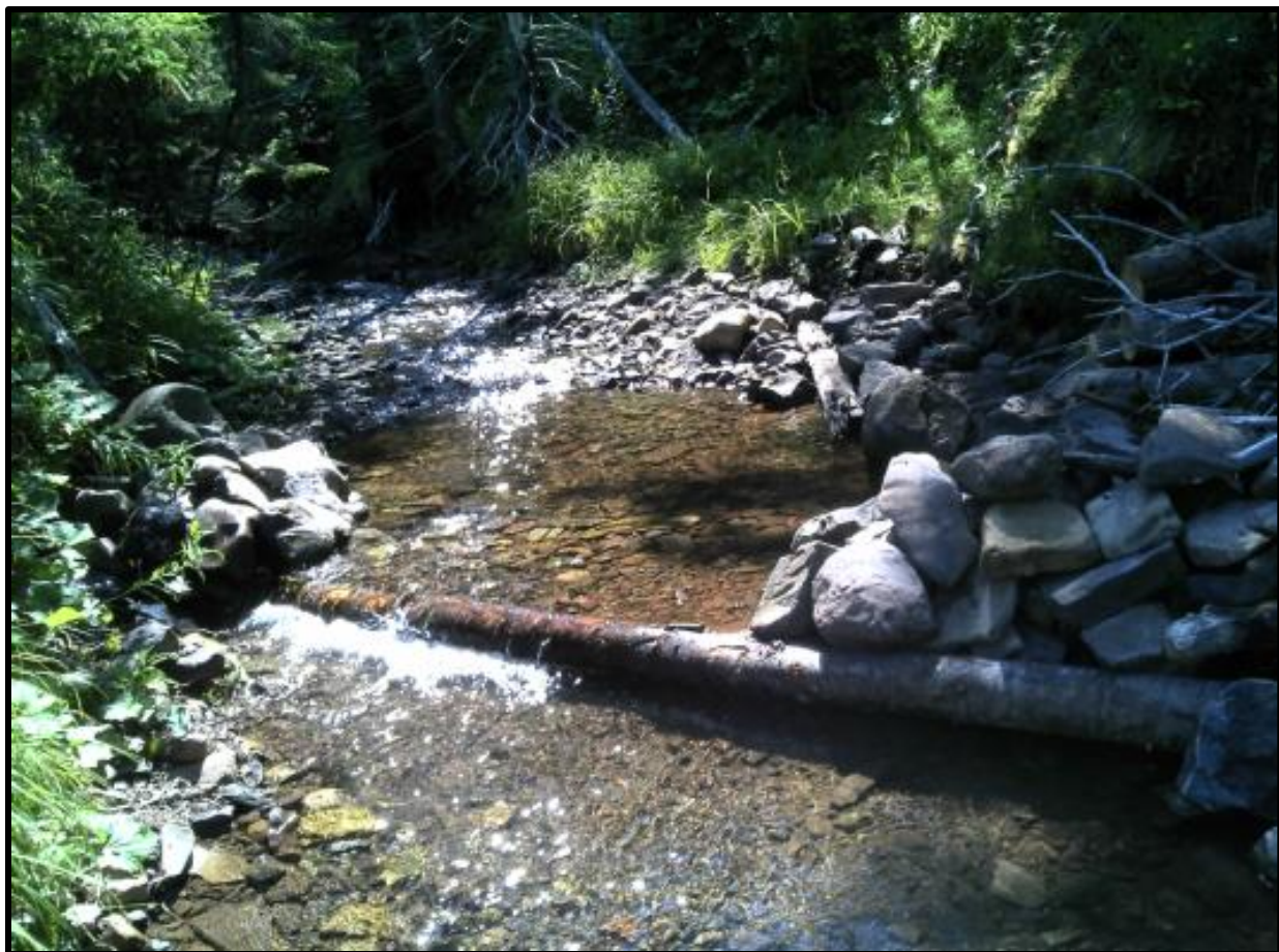
Figure 6: New structure recently built on the More Brook during the Enfield Training Session with Adopt a Stream.
