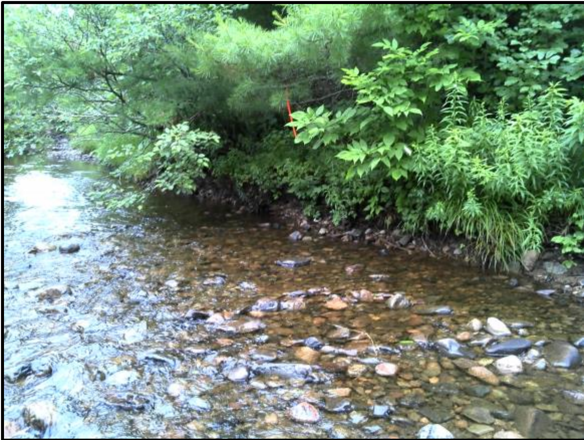
Figure 156. Before picture of a digger log and deflector structure for way point 217 and 218.
