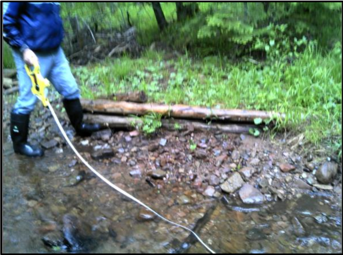
Figure 73. Deflector at waypoint 166 that needed maintenance.
