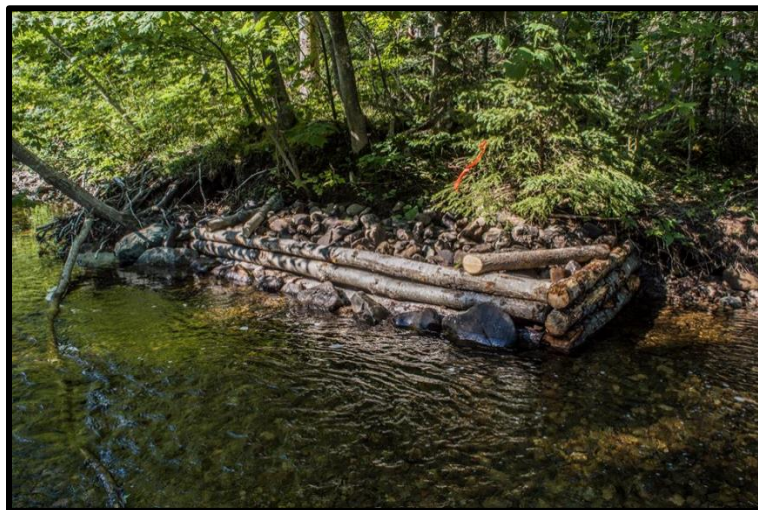
Figure 147. After picture of deflector at waypoint 206.
