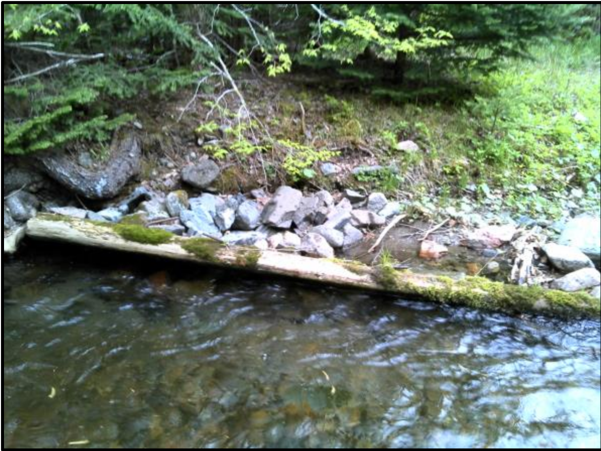
Figure 41. Deflector structure before maintenance.
