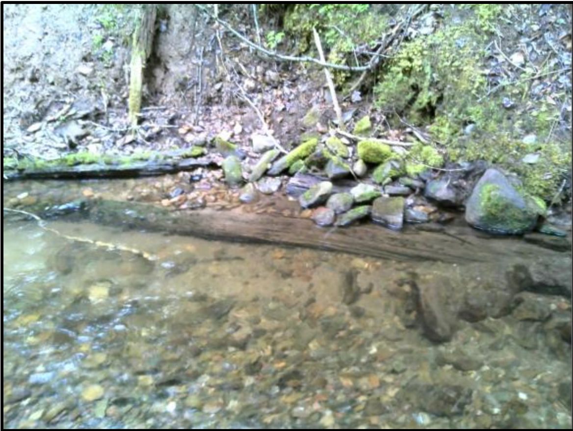
Figure 102. Deflector structure at waypoint 87.
