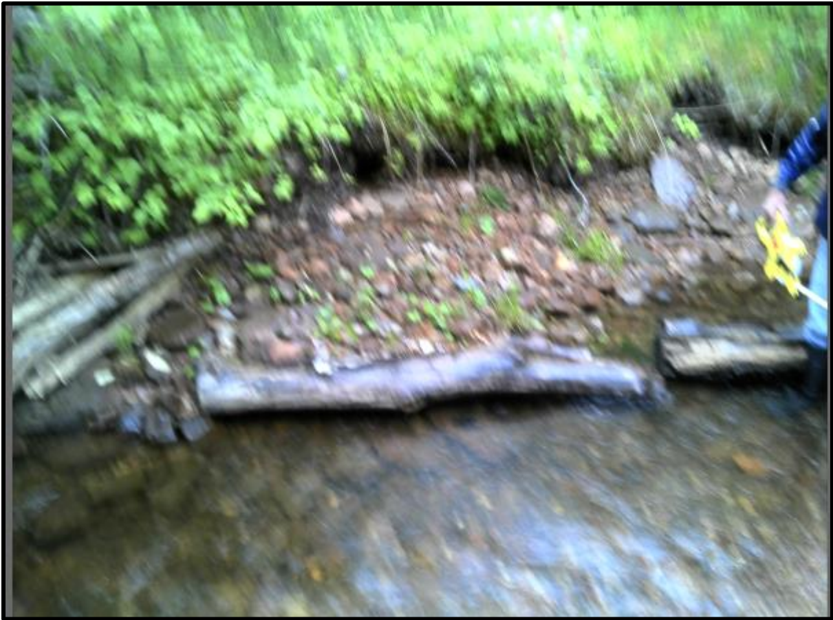
Figure 72. Deflector structure at waypoint 164.
