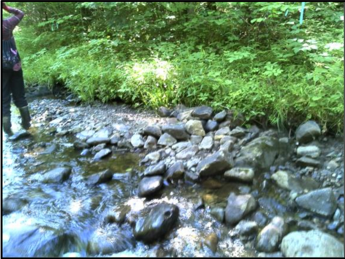
Figure 143. Before picture of deflector at way point 187.
