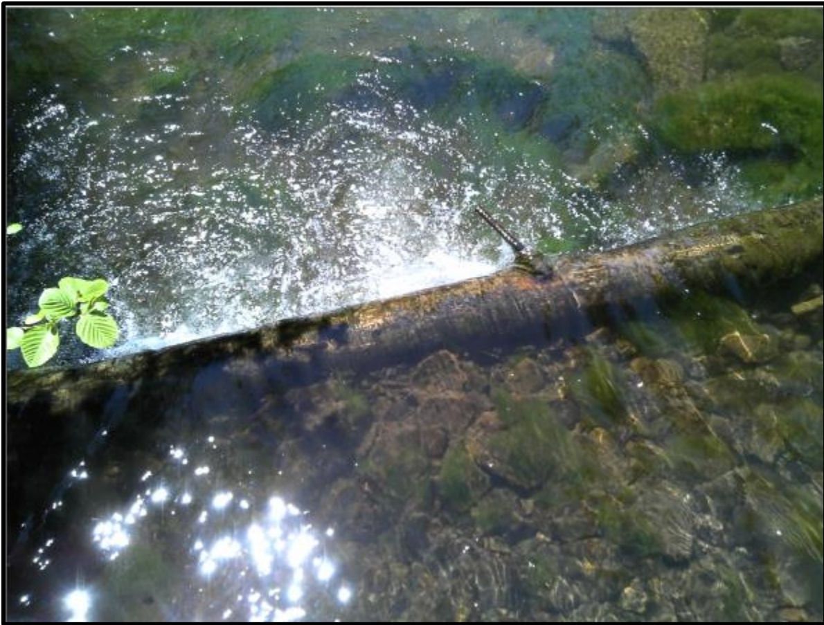
Figure 21. Maintained digger log structure on the Glendyre.
