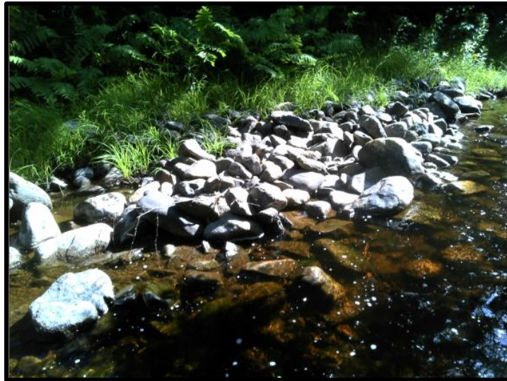
Figure 134. Before picture of deflector at way point 176.
