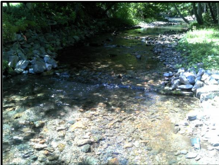
Figure 29. After picture of the digger log and deflector.
