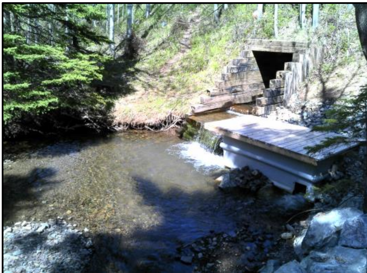
Figure 3: Fish Ladder, Bridge, and Culvert of the More Brook.
