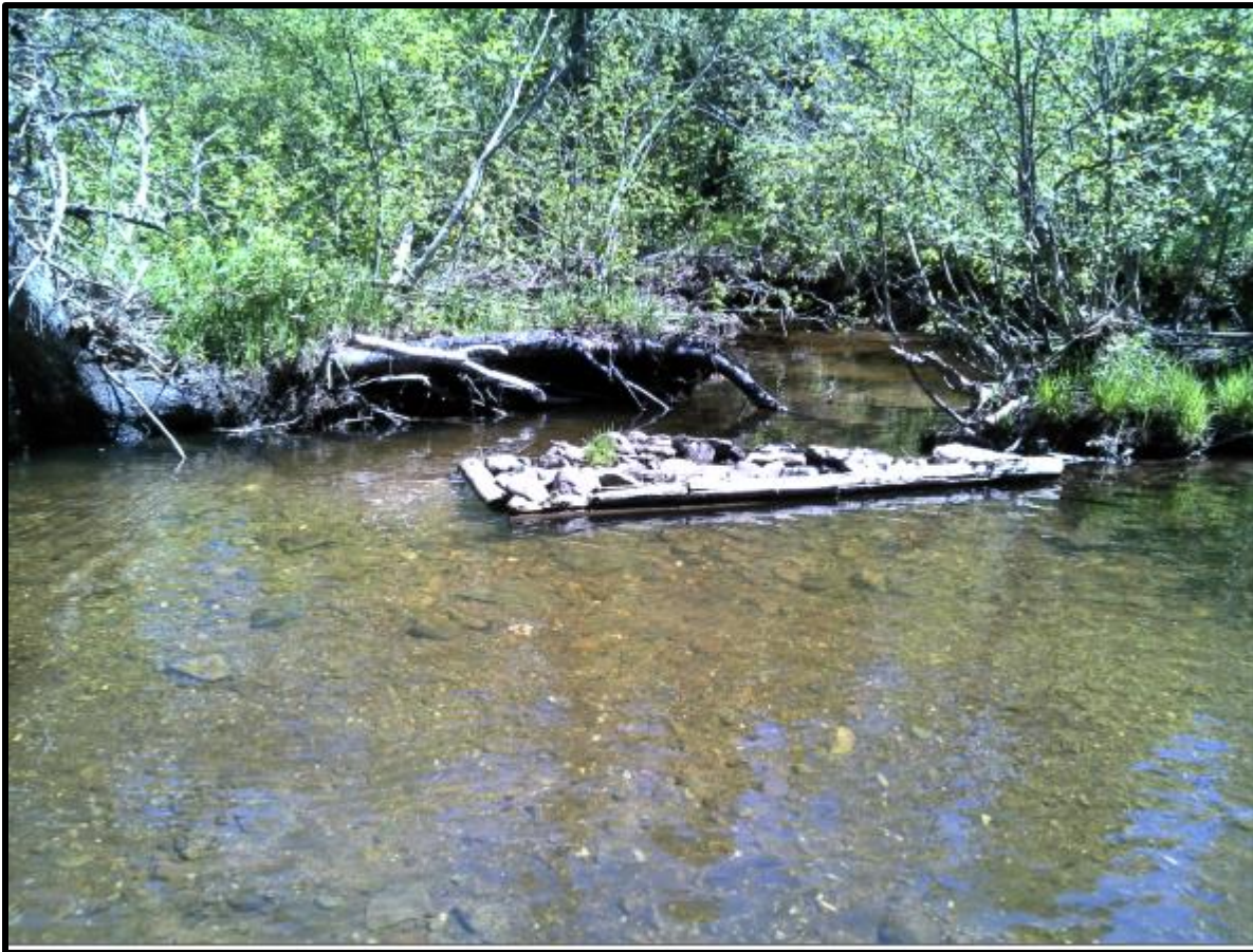
Figure 66. Deflector structure for waypoint 149.
