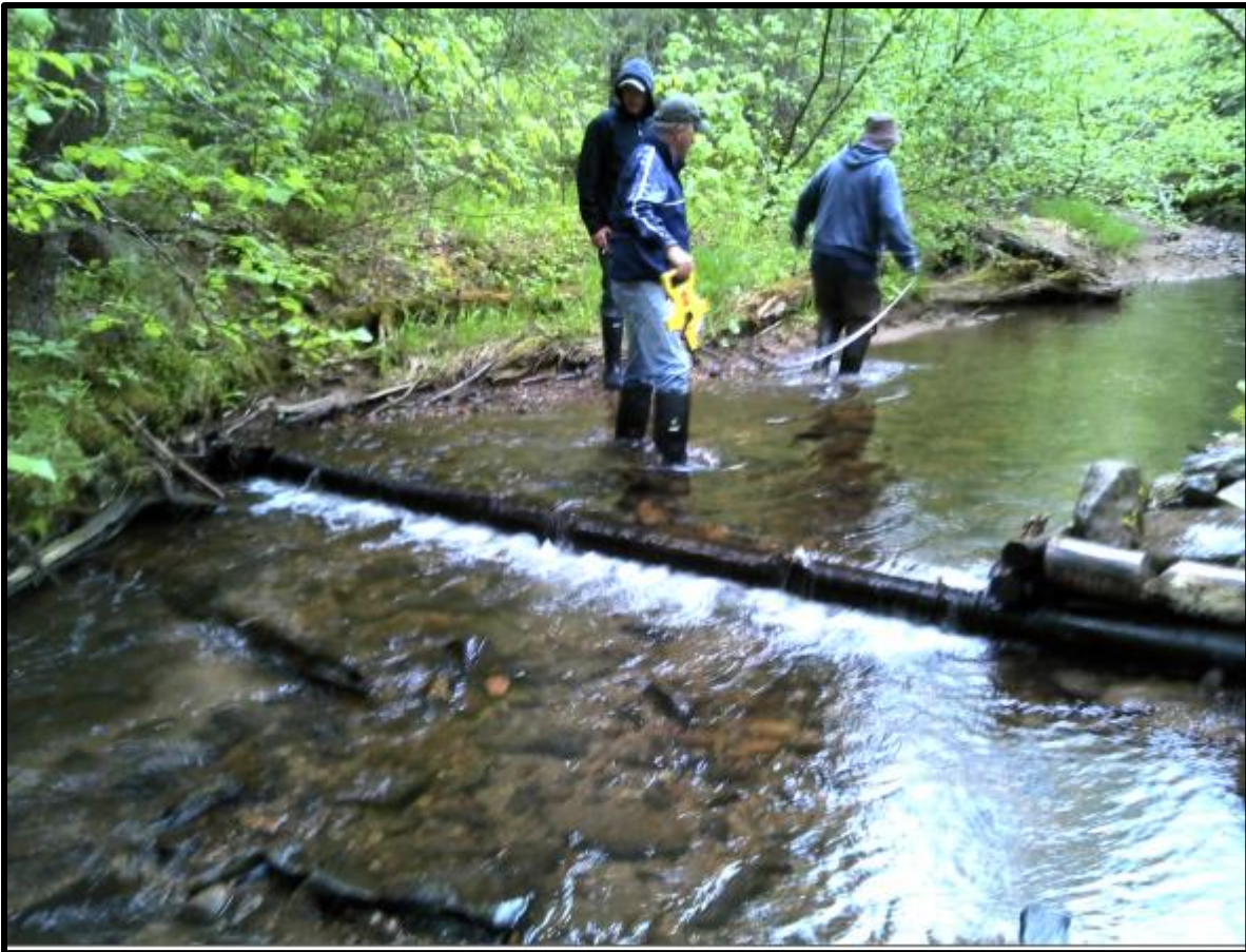
Figure 75. Digger log and deflector that was maintained at waypoint 168.
