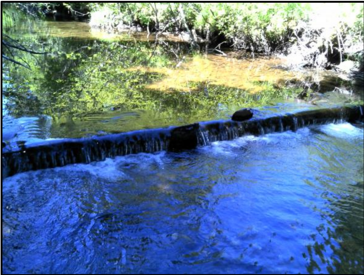
Figure 63. Digger log for waypoint 146.
