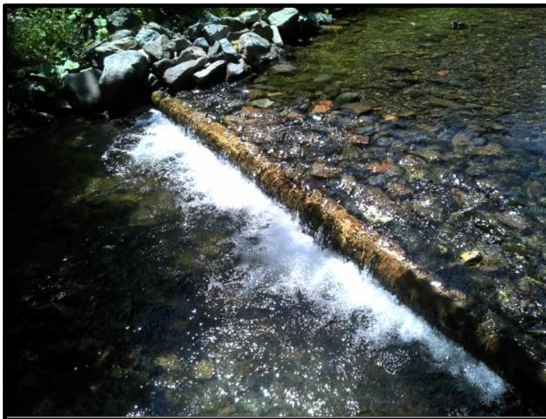
Figure 33. After picture of the digger log and deflector.
