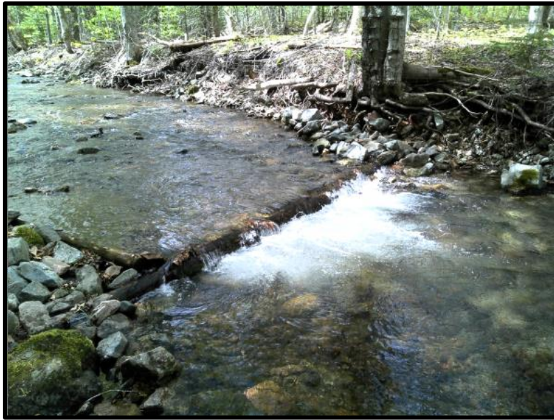
Figure 36. Before picture of a digger log and deflector structure that was maintained.
