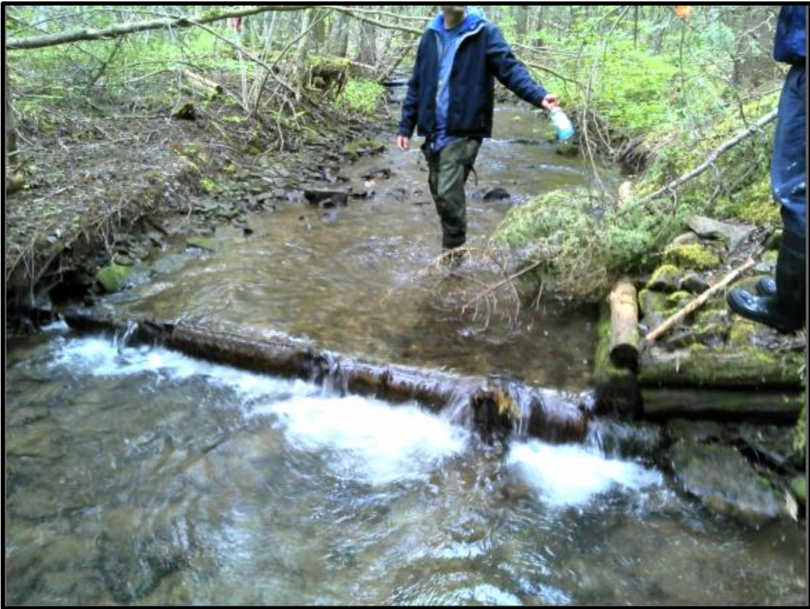
Figure 113. Digger Log and Deflector at waypoint 99.
