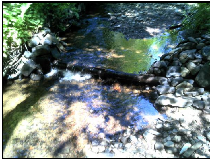
Figure 46. After picture of the digger log structure.
