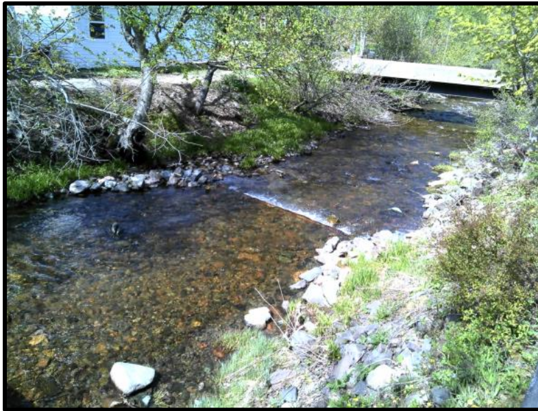
Figure 32. Before picture of the digger log and deflector.
