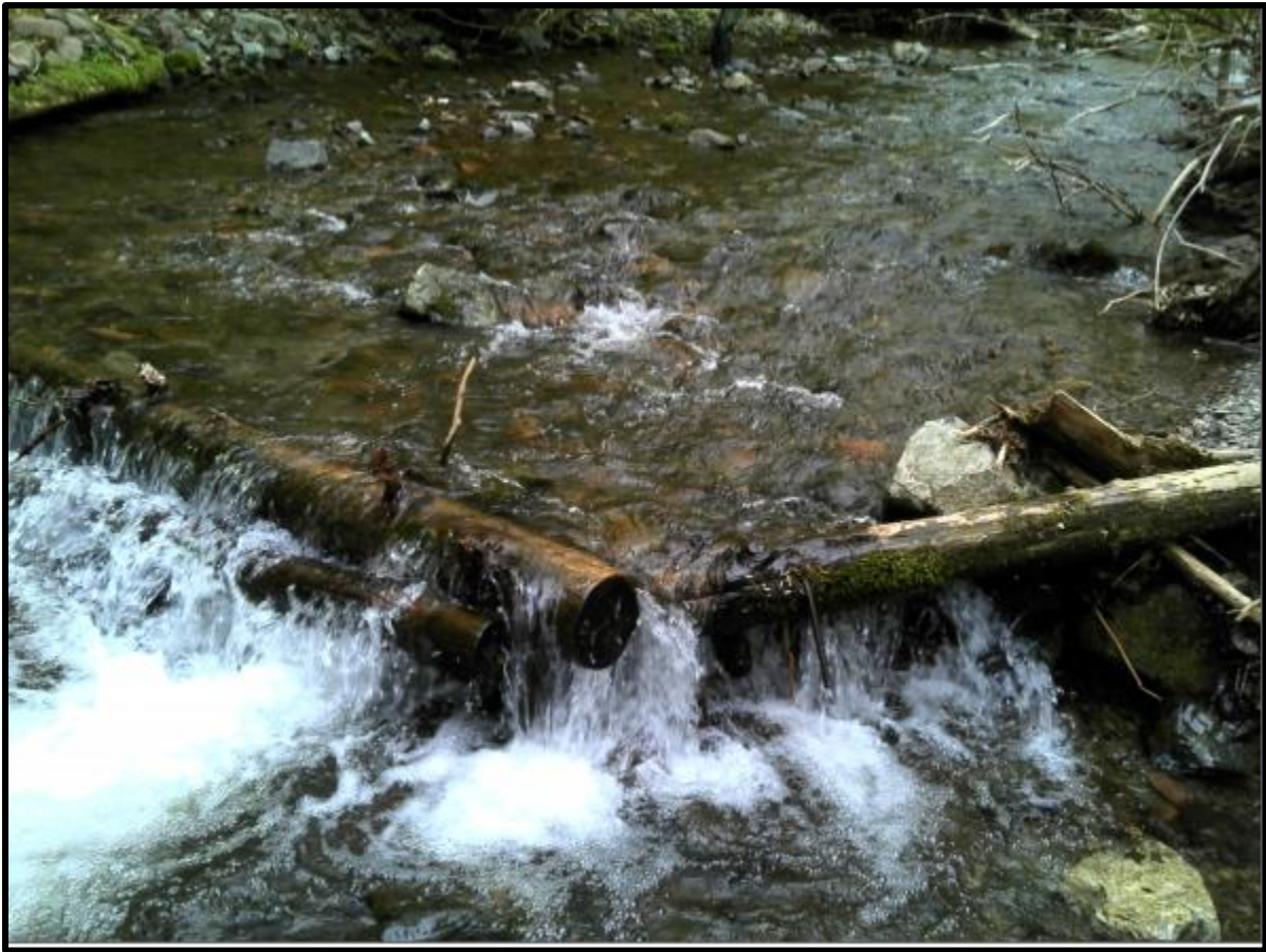
Figure 40. Digger log structure that needed maintenance.
