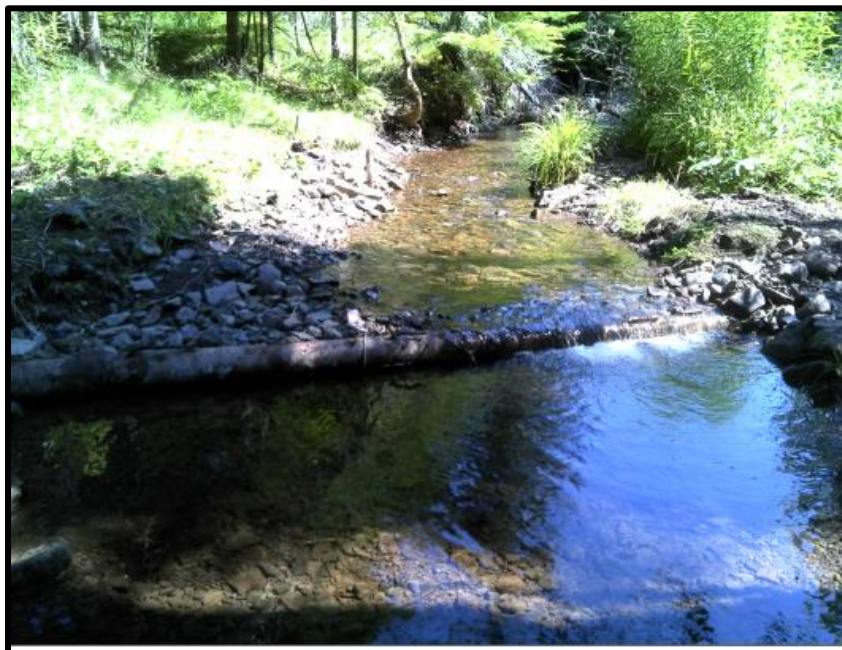
Figure 8. Replaced digger log structure installed by the Enfield Training Session with Adopt a Stream on the More Brook.
