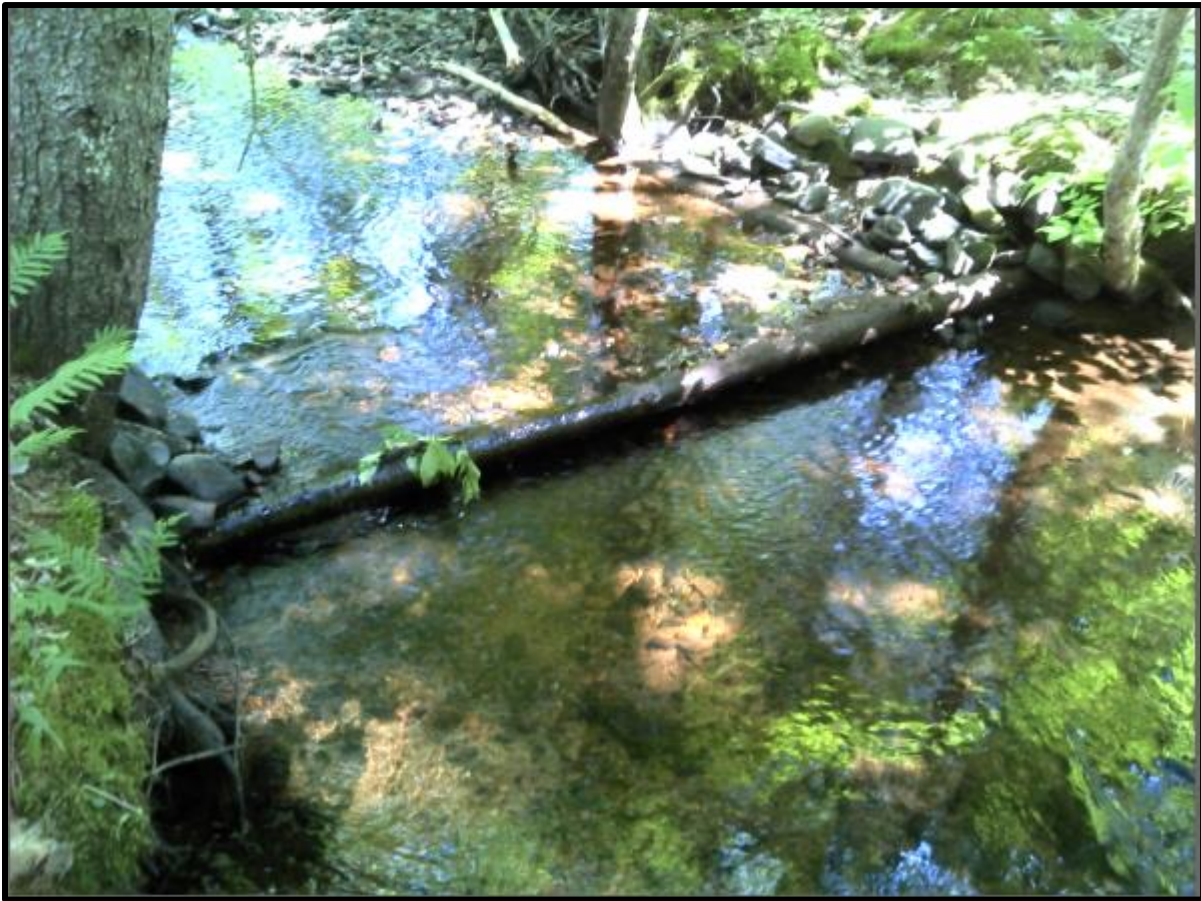
Figure 51. Photo of a digger log structure for waypoint 40.
