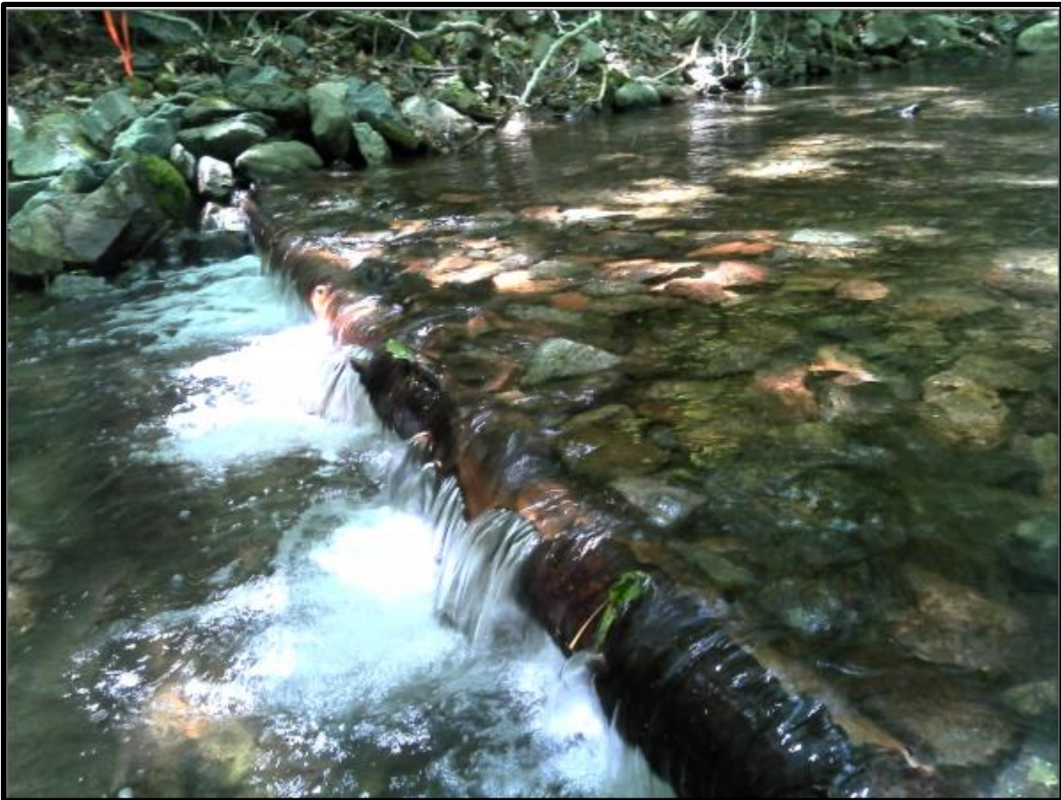
Figure 38. Digger log and deflector structure that was maintained.
