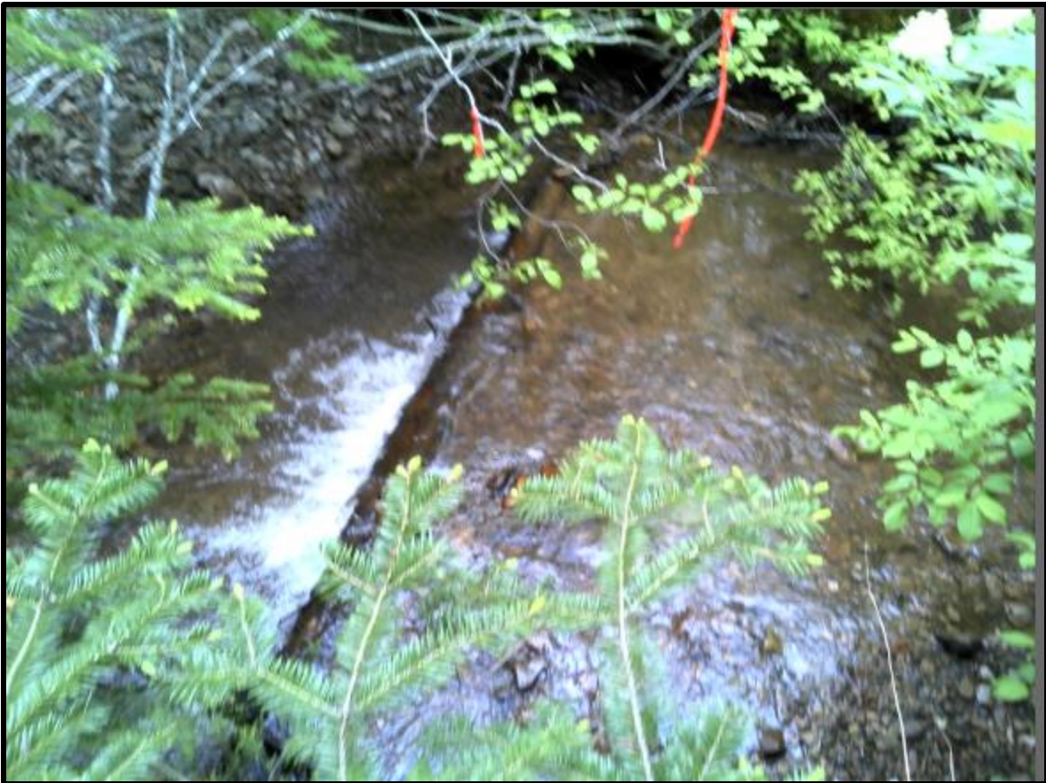
Figure 128. Digger Log structure at waypoint 117.
