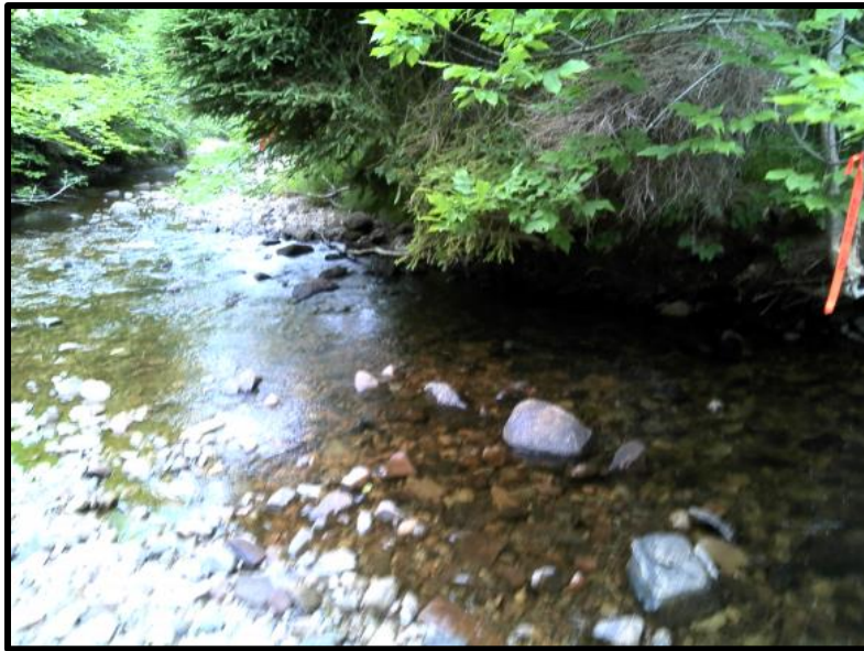
Figure 150. Before picture of deflector structure at way point 211.
