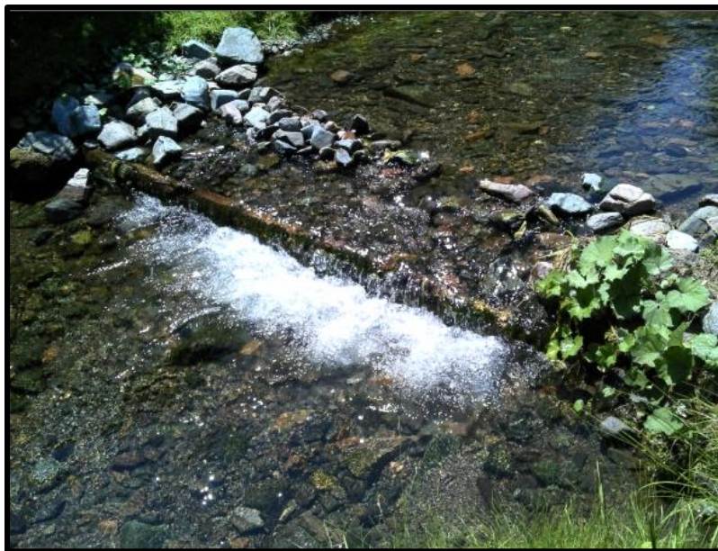
Figure 31. After picture of the digger log and deflector.
