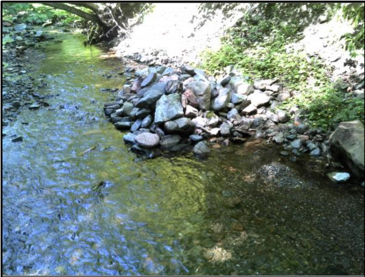
Figure 35. Deflector structure that was maintained. Digger log was buried.
