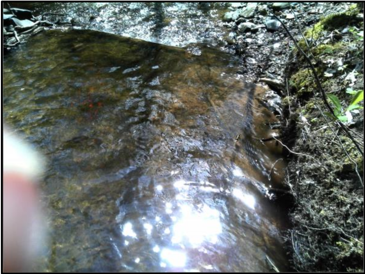
Figure 55. Digger Log structure for waypoint 44.
