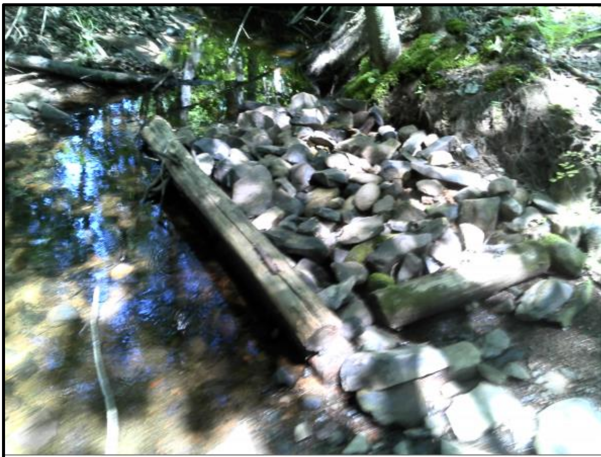
Figure 48. Deflector structure that was maintained.
