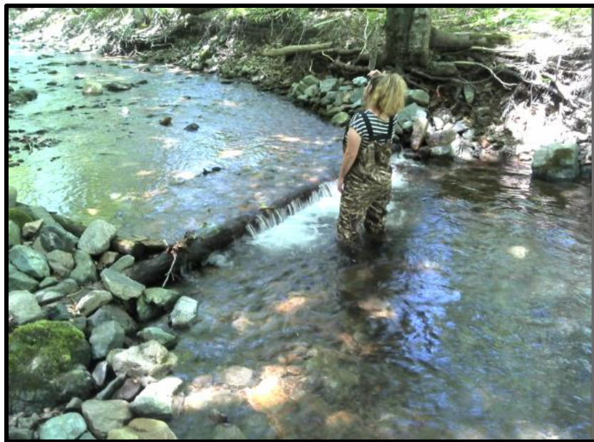
Figure 37. After picture of the digger log and deflector structure.
