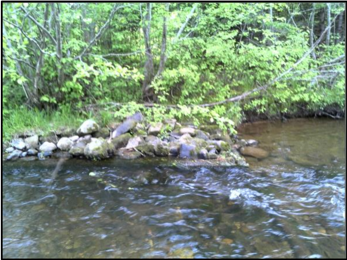
Figure 89. Deflector structure at waypoint 137.
