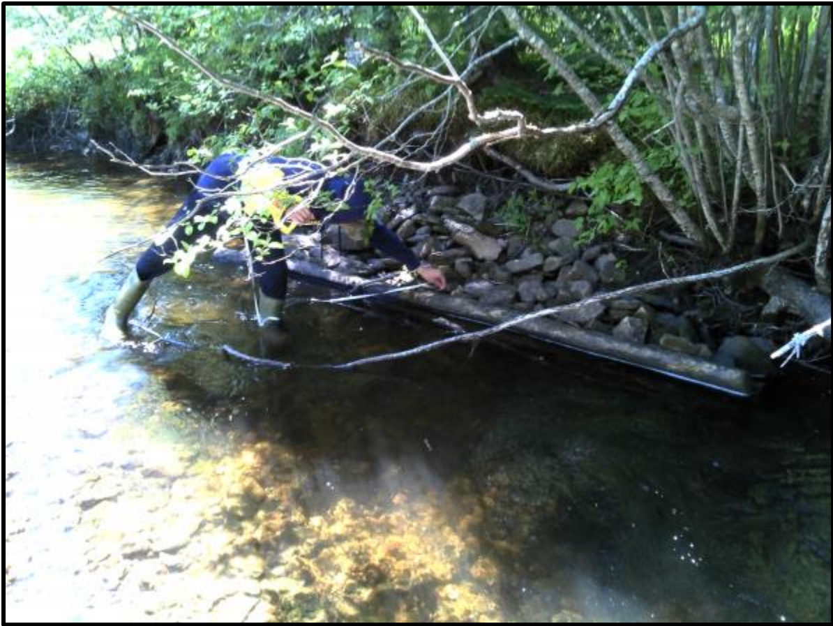
Figure 68. Deflector structure at waypoint 151 that was maintained.
