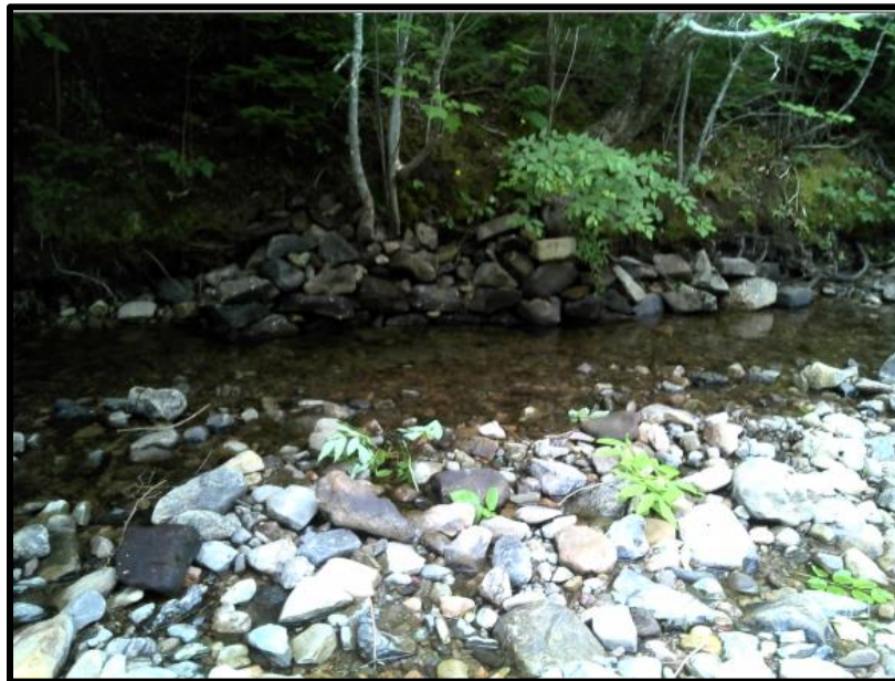
Figure 149. Progress picture of bank rock structure for way point 209.
