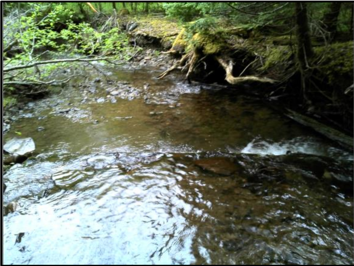
Figure 111. Digger Log Structure at waypoint 96.
