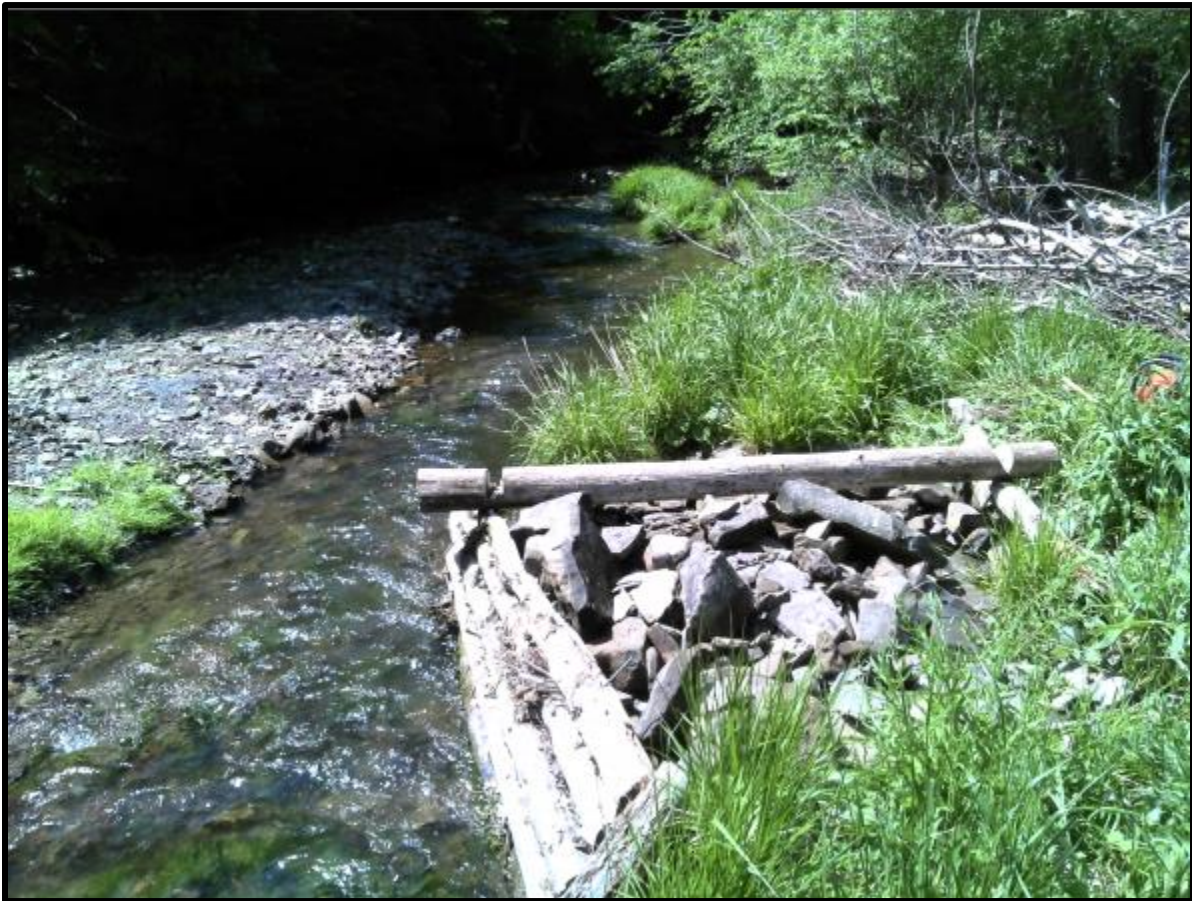
Figure 22. Deflector that was maintained at waypoint 139.
