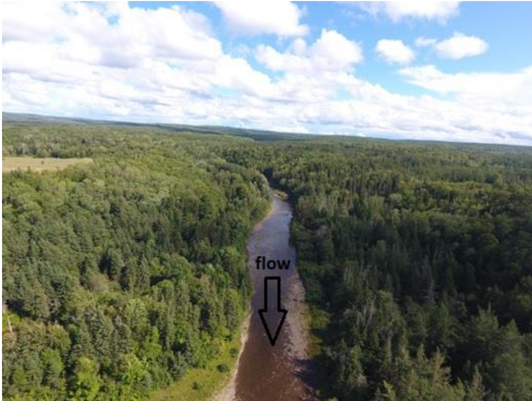
Figure 26: 3.5km above Moran Road bridge. Channel lacks meander pattern and is over-widened (Upstream view).
