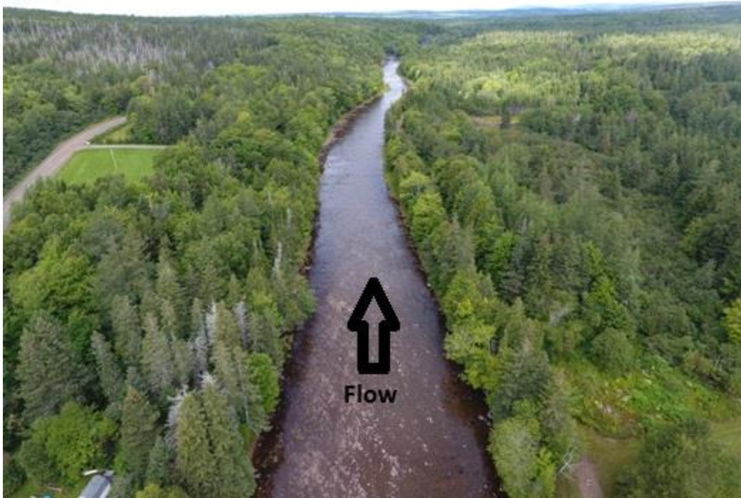
Figure 28: Downstream view below Rear Intervale Rd. Bridge. Channel lacks meander pattern, is over-widened and heavily bedrock laden.
