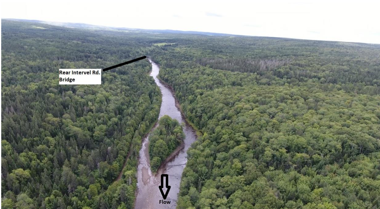
Figure 27: Looking upstream towards Rear Intervale Rd. bridge. Channel is over-widened, and the bottom substrate is predominantly bedrock for over 1km. This section of stream is easily accessible by heavy machinery.
