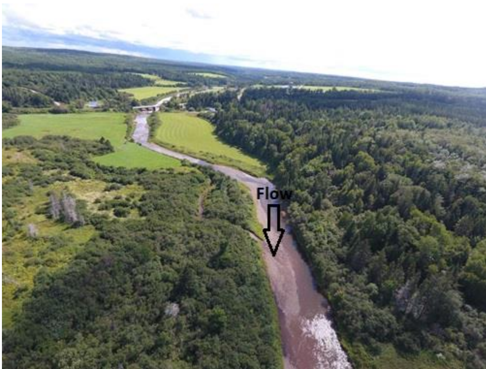
Figure 8: Upstream view of Route 19 Bridge. Channel lacks proper meander pattern, is over widened and has insufficient riparian zone.
