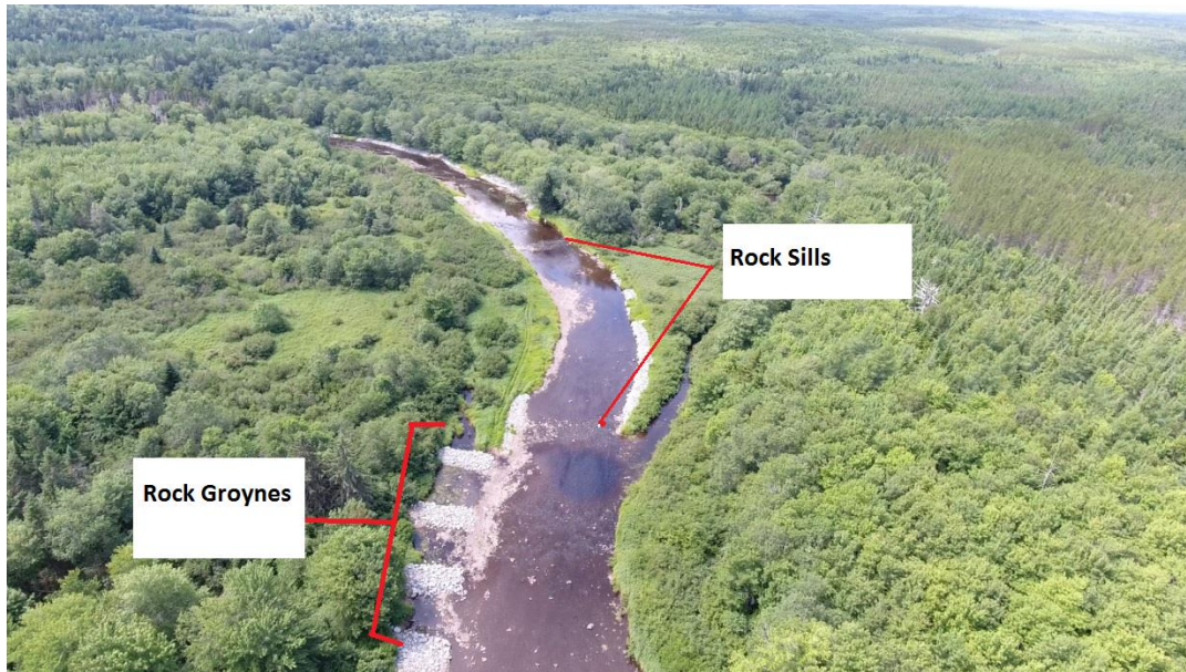
Figure 48: An example of how multiple structures function in combination. Sills dig pools and groynes collect settling sediments below (Source – MacInnis Natural Resource Services Inc).
