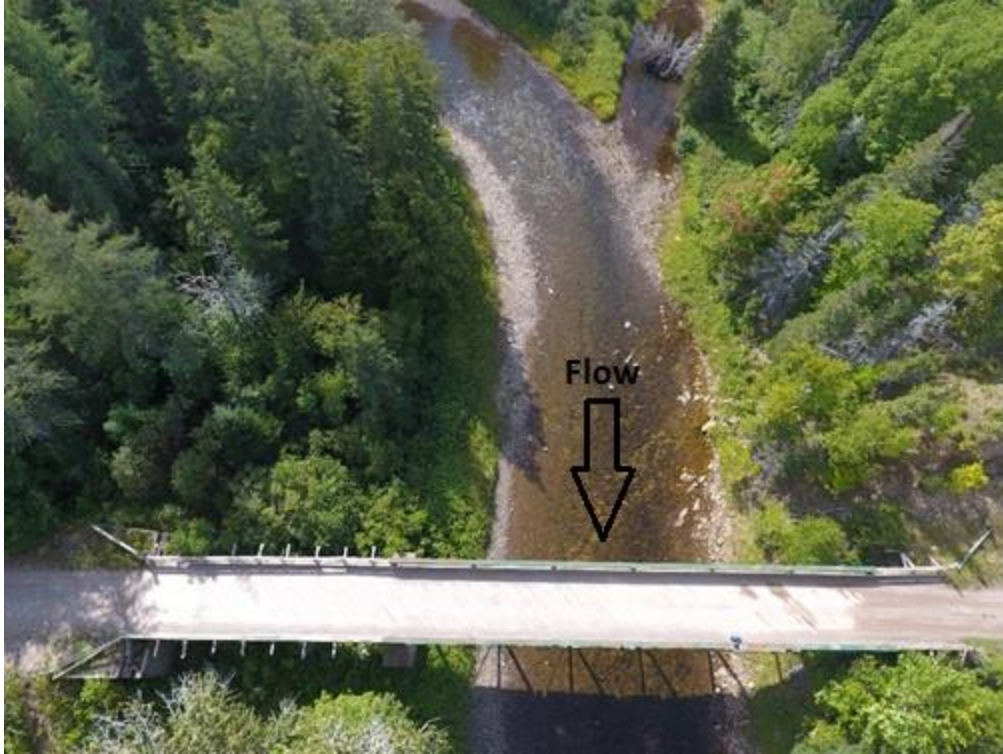
Figure 20: View above Moran Road bridge. (Note: little access for machines below bridge due to steep slopes)
