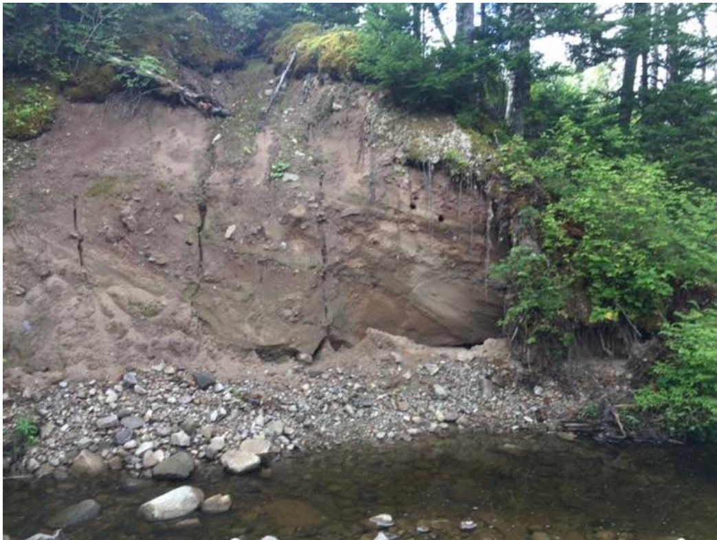
Figure 44: Actively eroding bank, downstream from unnamed tributary - MacLeod Settlement road crossing
